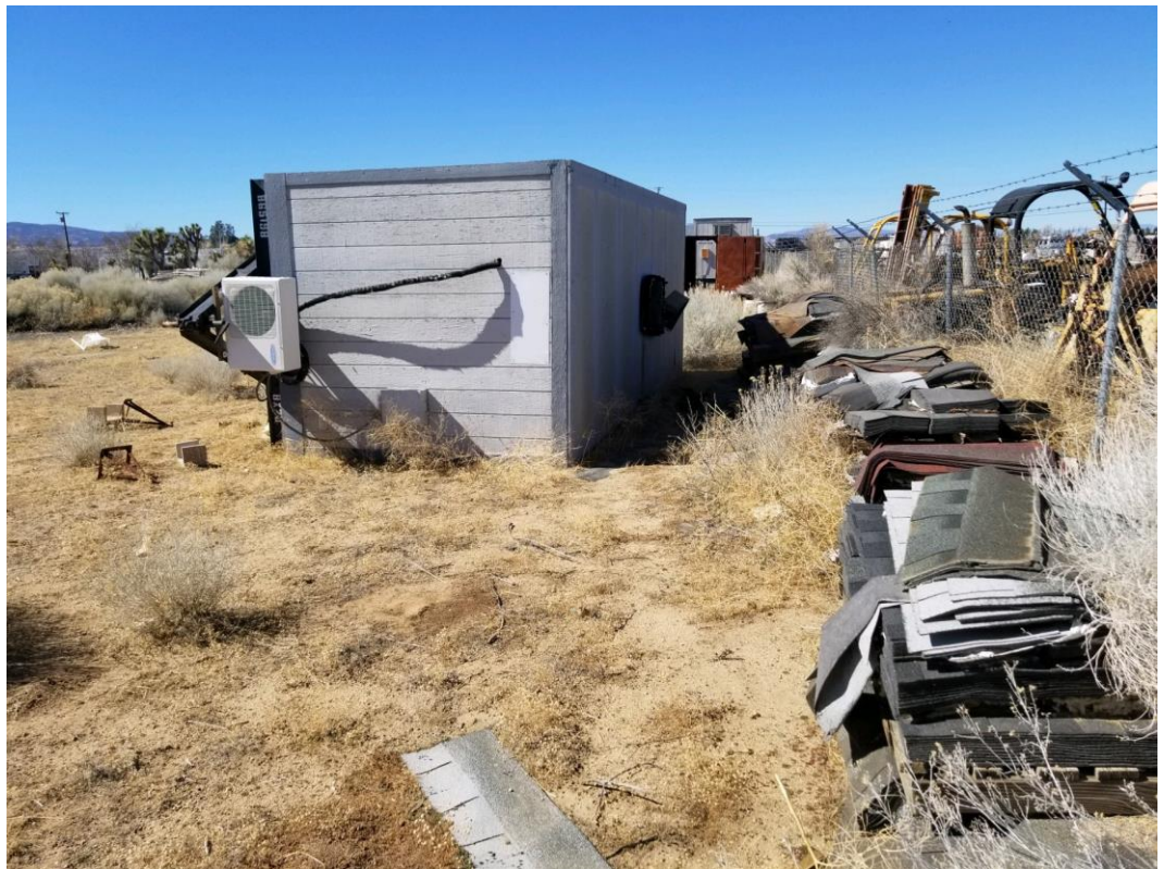
12. View looking west from the northeast corner, viewing an office trailer on its side and debris.
