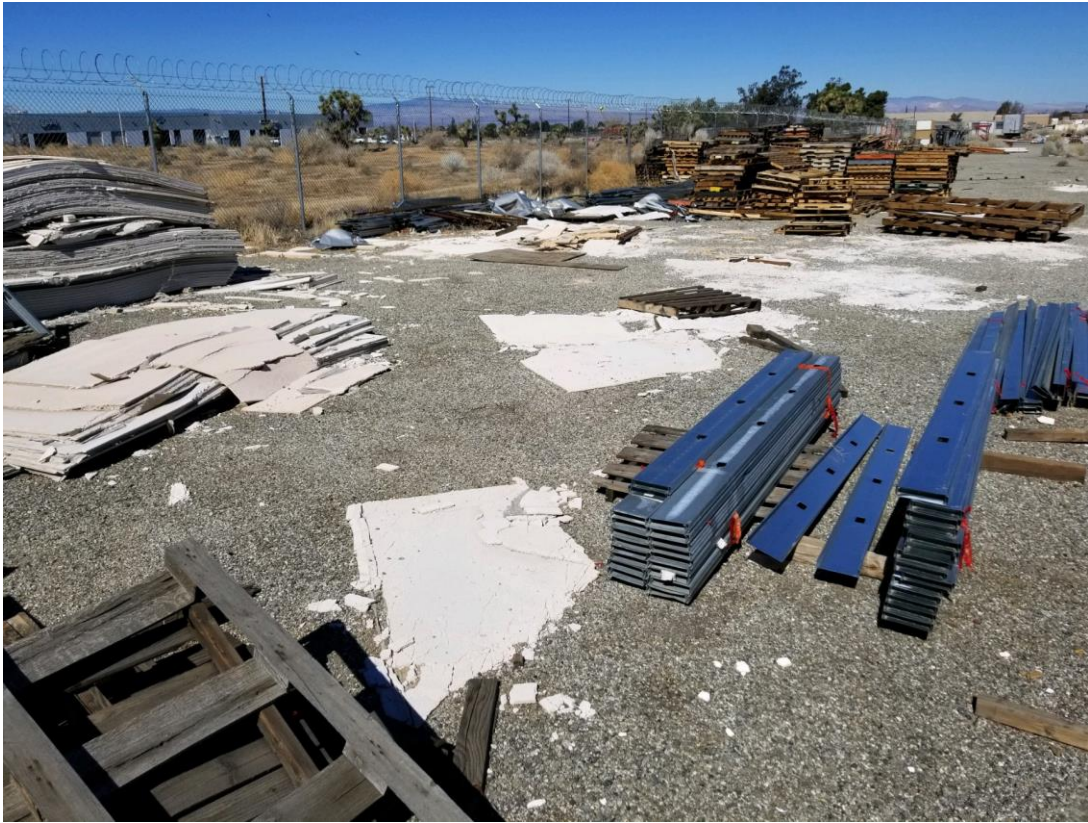
3. Leftover construction related debris located on the west side of the Site.
