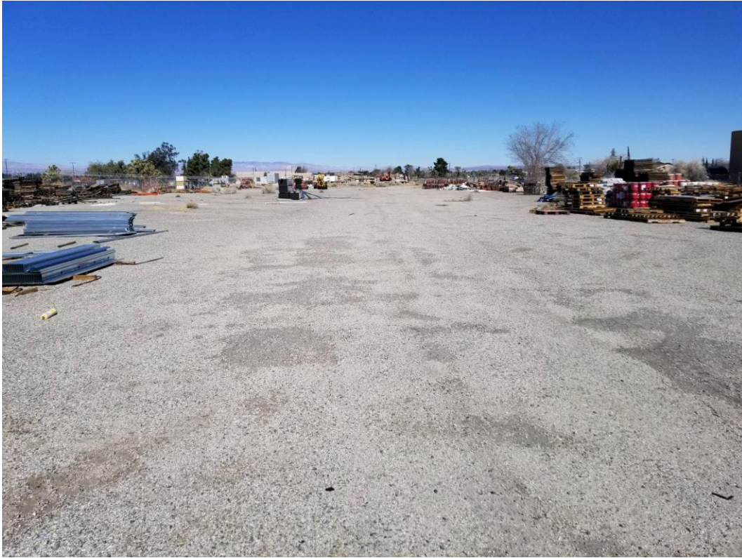
1. View looking north from just inside the entrance on the south side of the Site, adjacent to Avenue L-12.
