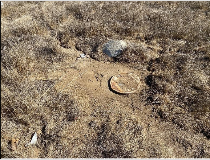
19. View of an apparent groundwater monitoring well on Parcel B along Redlands Avenue
