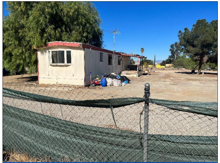
10. View of the mobile home, concrete pad from demolished shed, and trash
