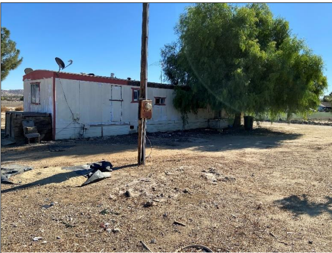
3. View of mobile home facing southeast from Redlands Avenue
