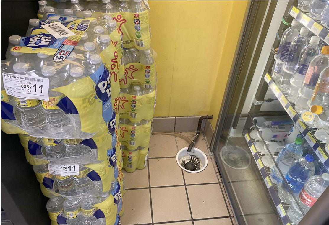
Photo No. 5 Typical floor drain in convenience store
