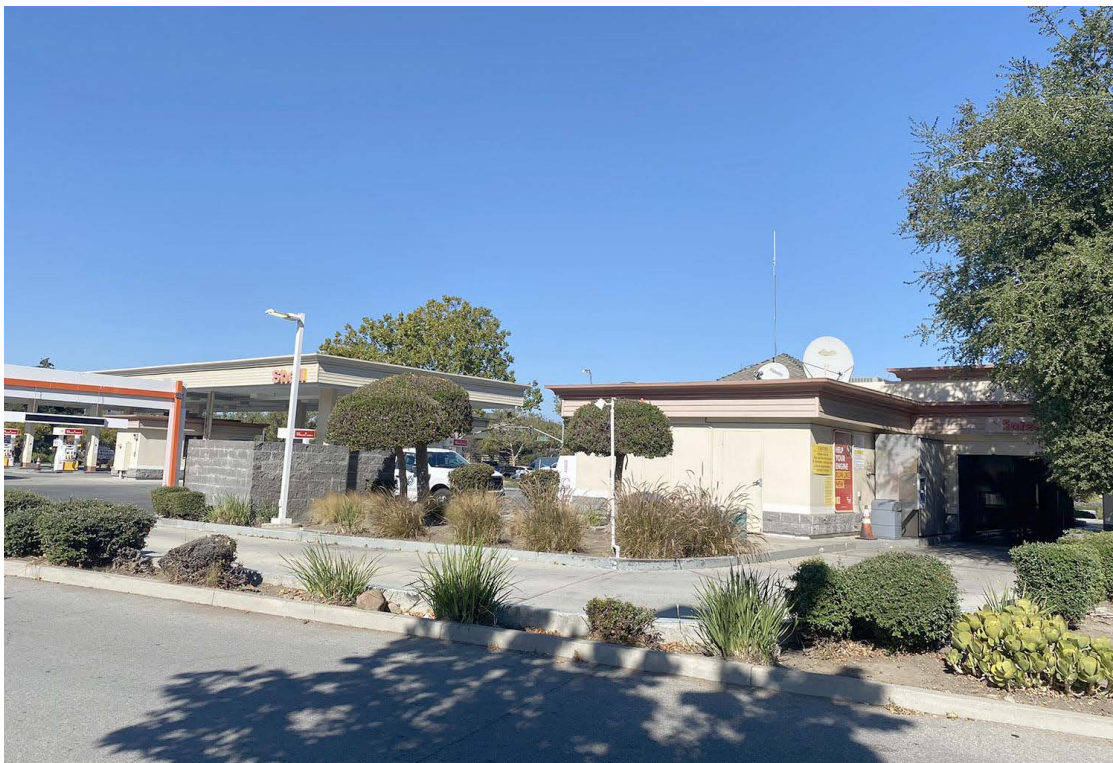
Photo No. 10 View to the northwest of car wash entrance
