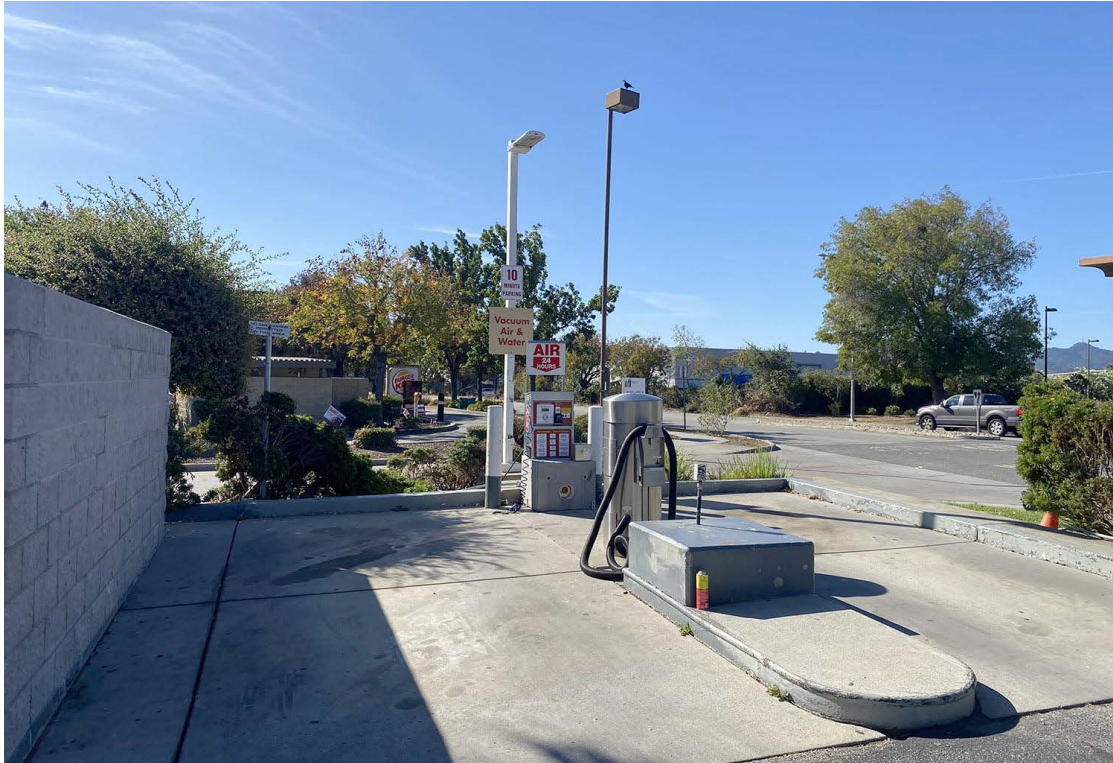
Photo No. 19 Coin/card-operated vacuum, air, and water station in southwestern portion of Site
