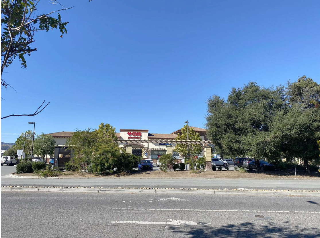
Photo No. 29 View to the west across Walnut Grove Drive of CVS Pharmacy
