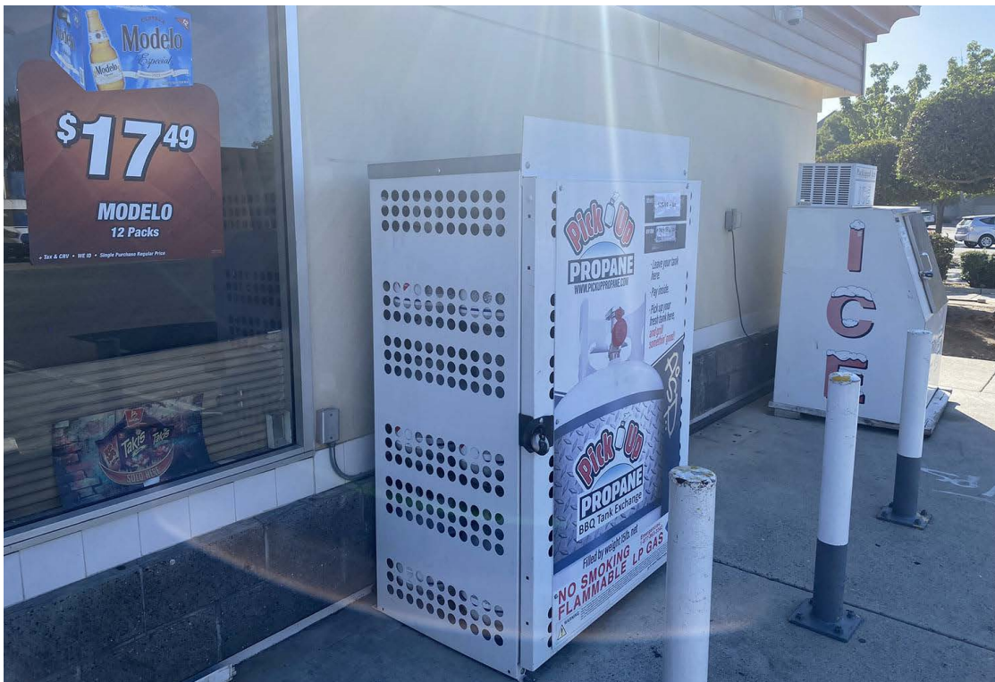
Photo No. 18 Propane tank and ice storage along western side of convenience store
