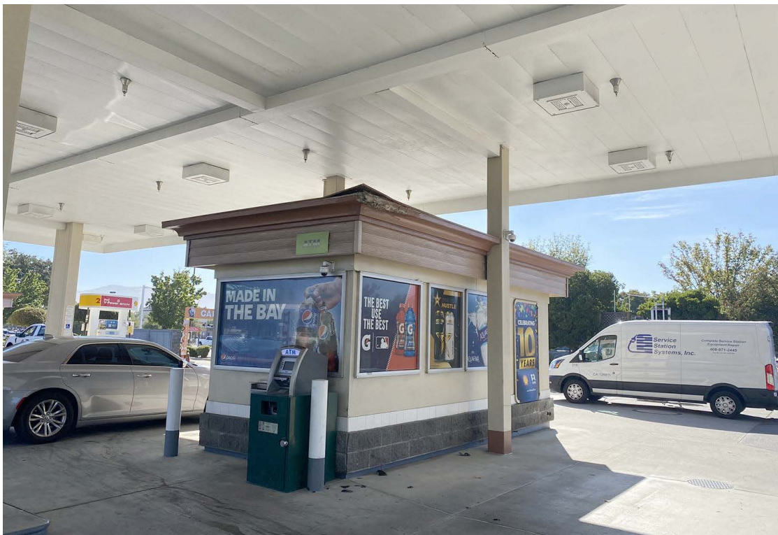
Photo No. 2 Fuel pump building
