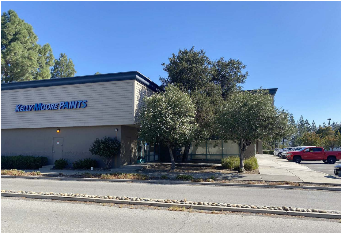
Photo No. 26 View to the east of Kelly-Moore Paints
