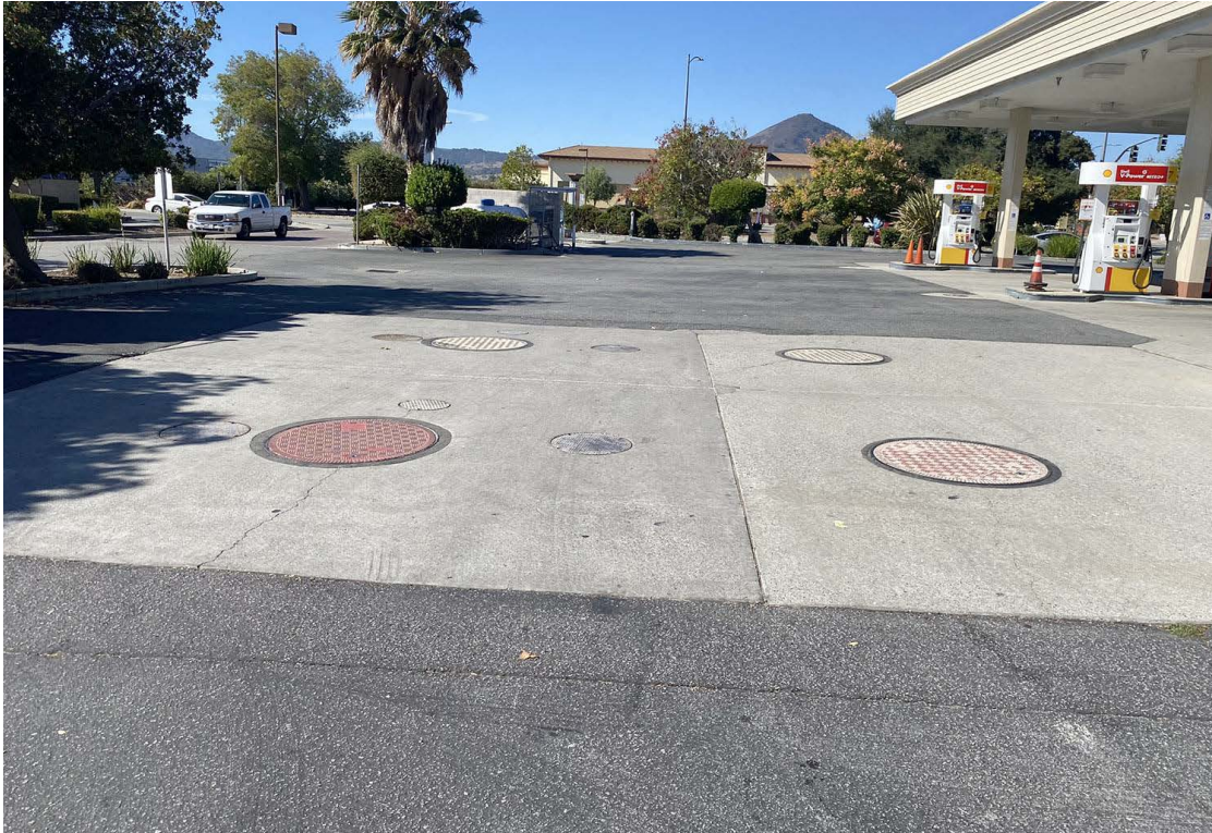
Photo No. 15 Gasoline UST access/fill ports in south central portion of the Site
