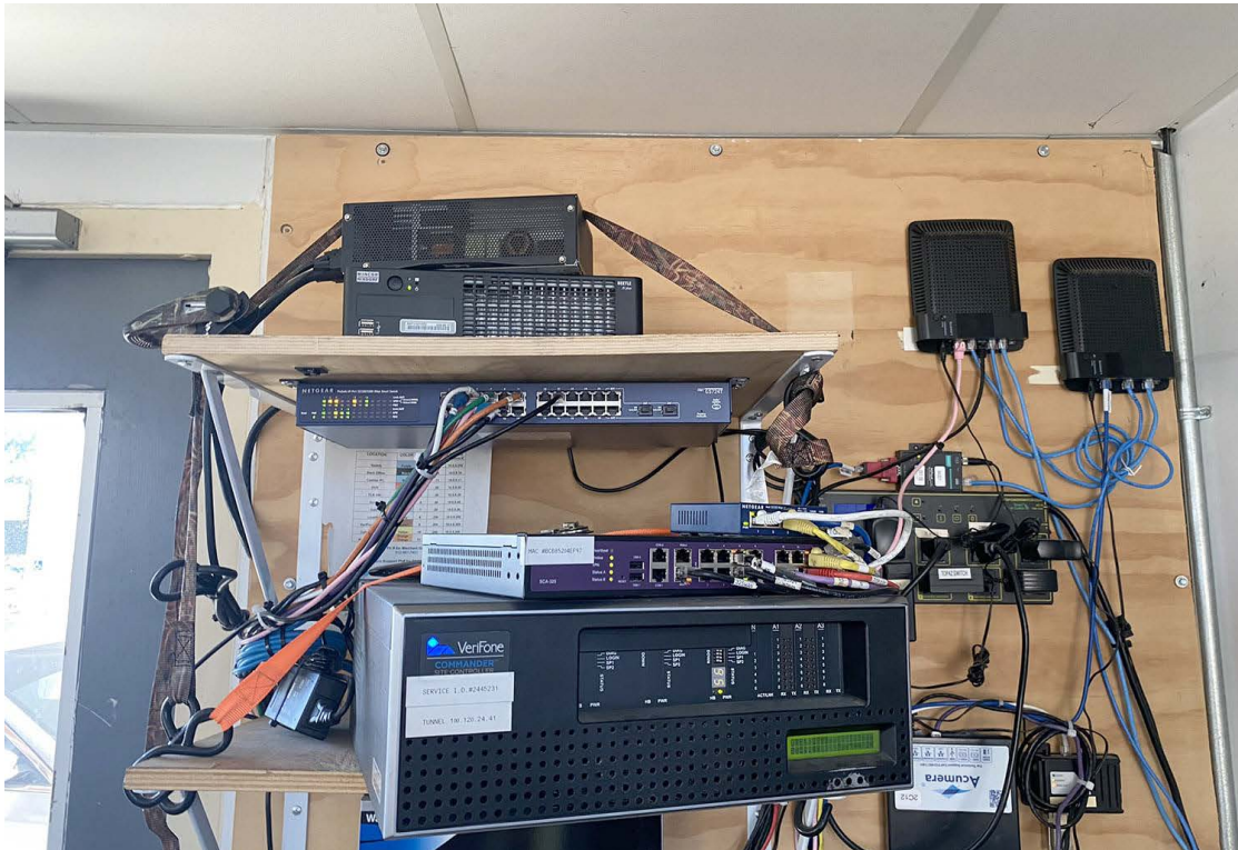
Photo No. 13 Computer systems for leak detection systems in small Site building
