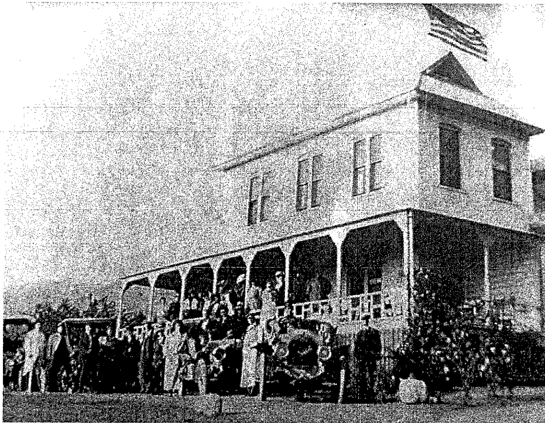
Atwood house (Feature 1), painted white circa 1910, before second-story porch was added. Front (west) and south elevations. View to northeast. (Photo courtesy of Yucaipa Valley Historical Society Museum)
