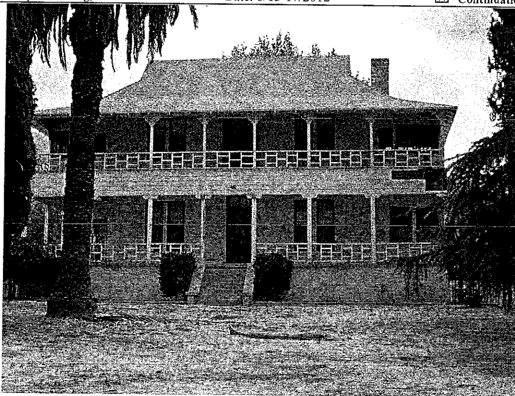
Casa Blanca Ranch house (Feature 1), front (west) elevation. View to east, 8/17/2012.
