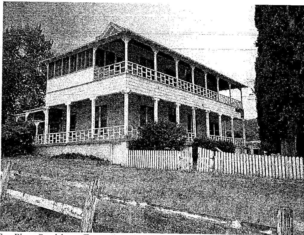
Casa Blanca Ranch house (Feature 1), north and front (west) elevations. View to southeast, 8/17/2012.
