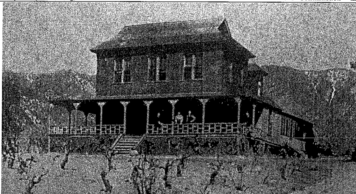
Dunlap house (Feature 1) circa 1900, front (west) and south elevations. View to northeast. (Photo courtesy of Yucaipa Valley Historical Society Museum)
