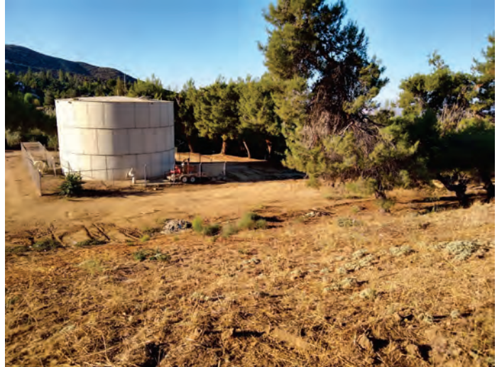
Photo 6: View of the existing tank facing south.
