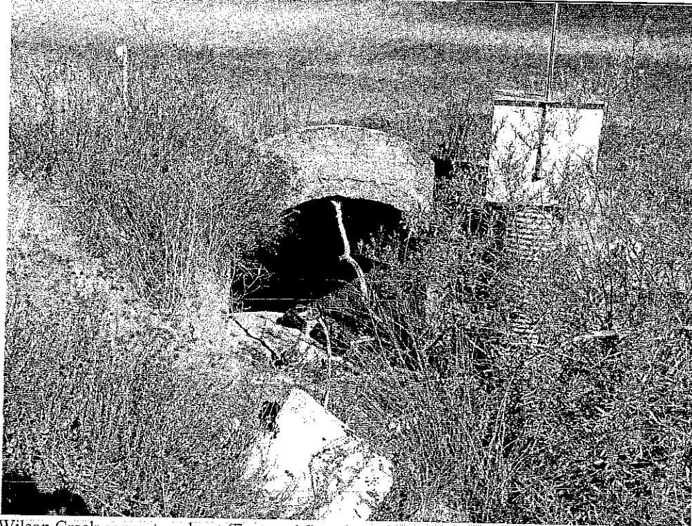
Wilson Creek concrete culvert (Feature 16) under Jefferson Street. View to west, 8/15/2012.
