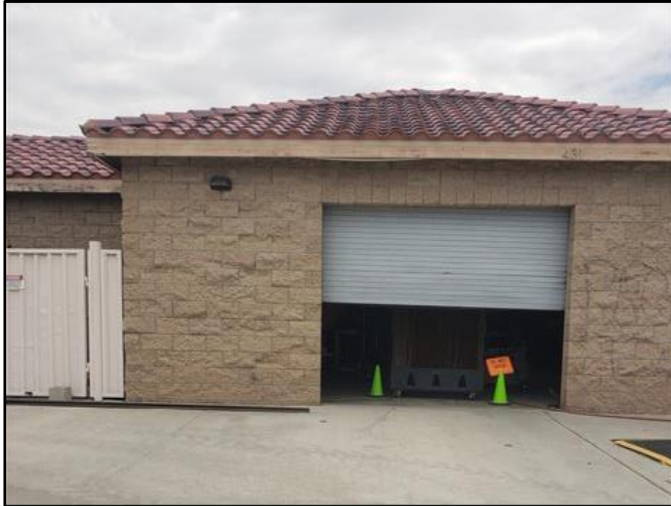
Photo 8. View of west building of the subject property, facing north.
