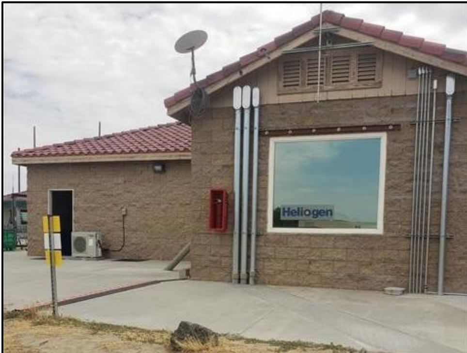
Photo 7. View of west building of the subject property, facing east.
