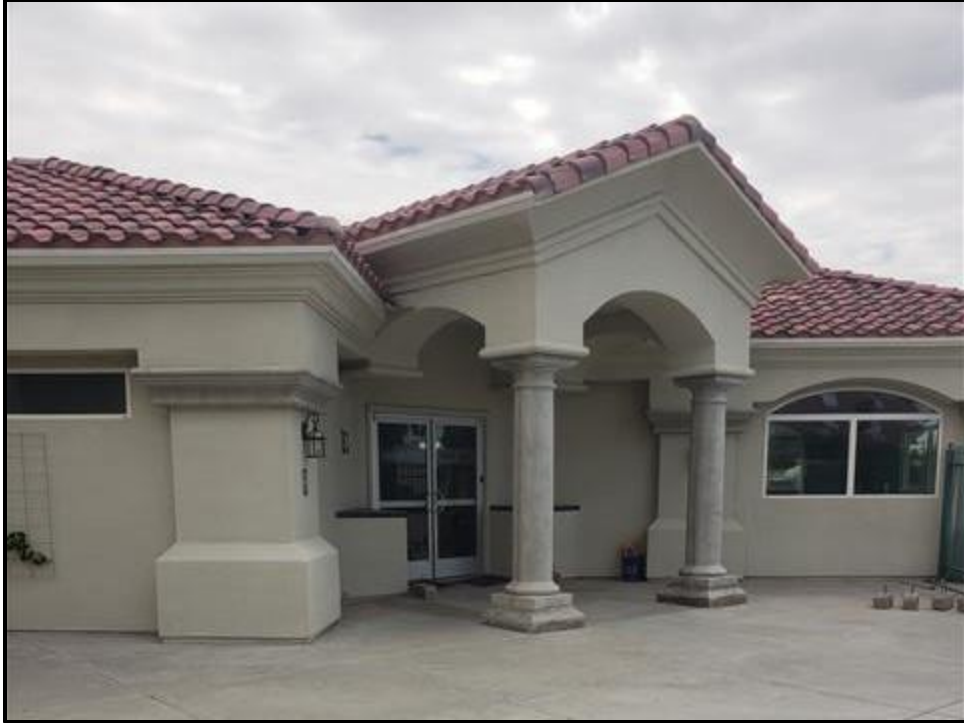
Photo 14. West side of northeast building.
