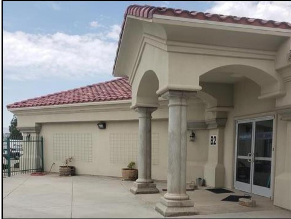
Photo 10. East side of the northeastern building.
