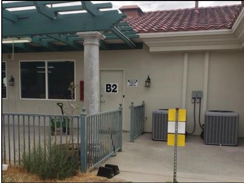
Photo 12. North side of the northeast building.
