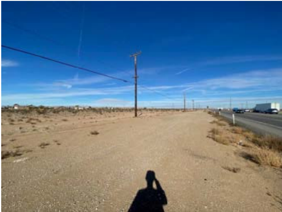
Site overview. View to northwest.
