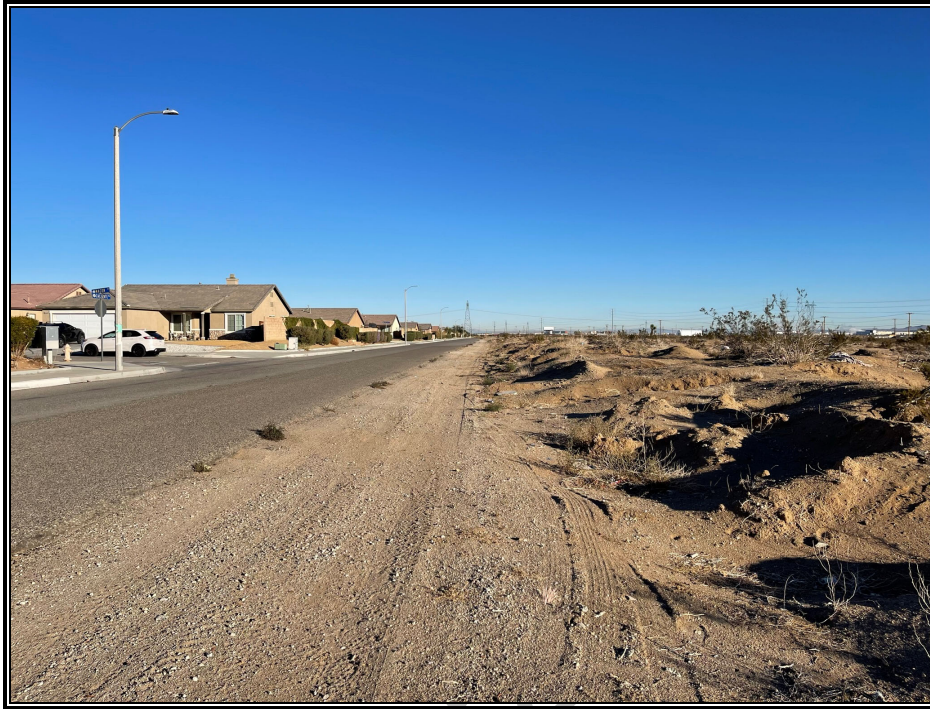
View north along Caliente Road, west of subject property.
