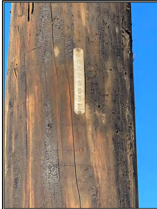
Existing utility pole on HWY 395 for AT&T proposed POC.
