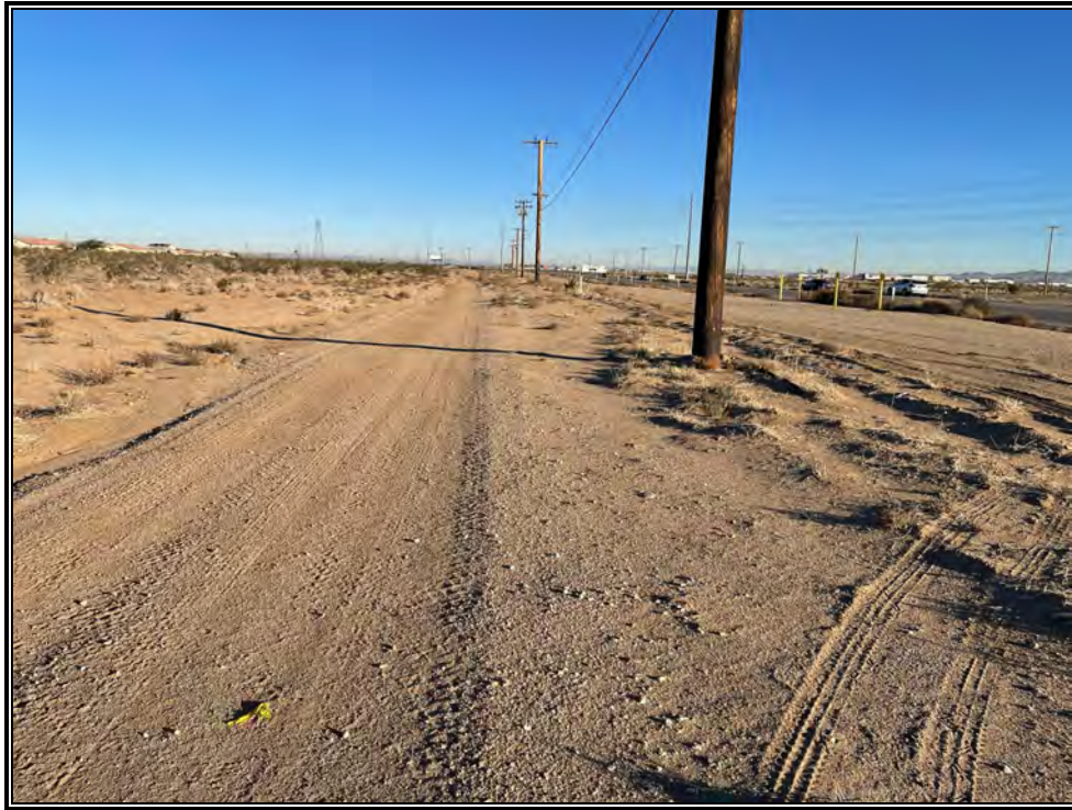
View north from utility trench route at HWY 395.
