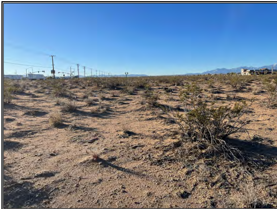
View south from proposed utility trench route.
