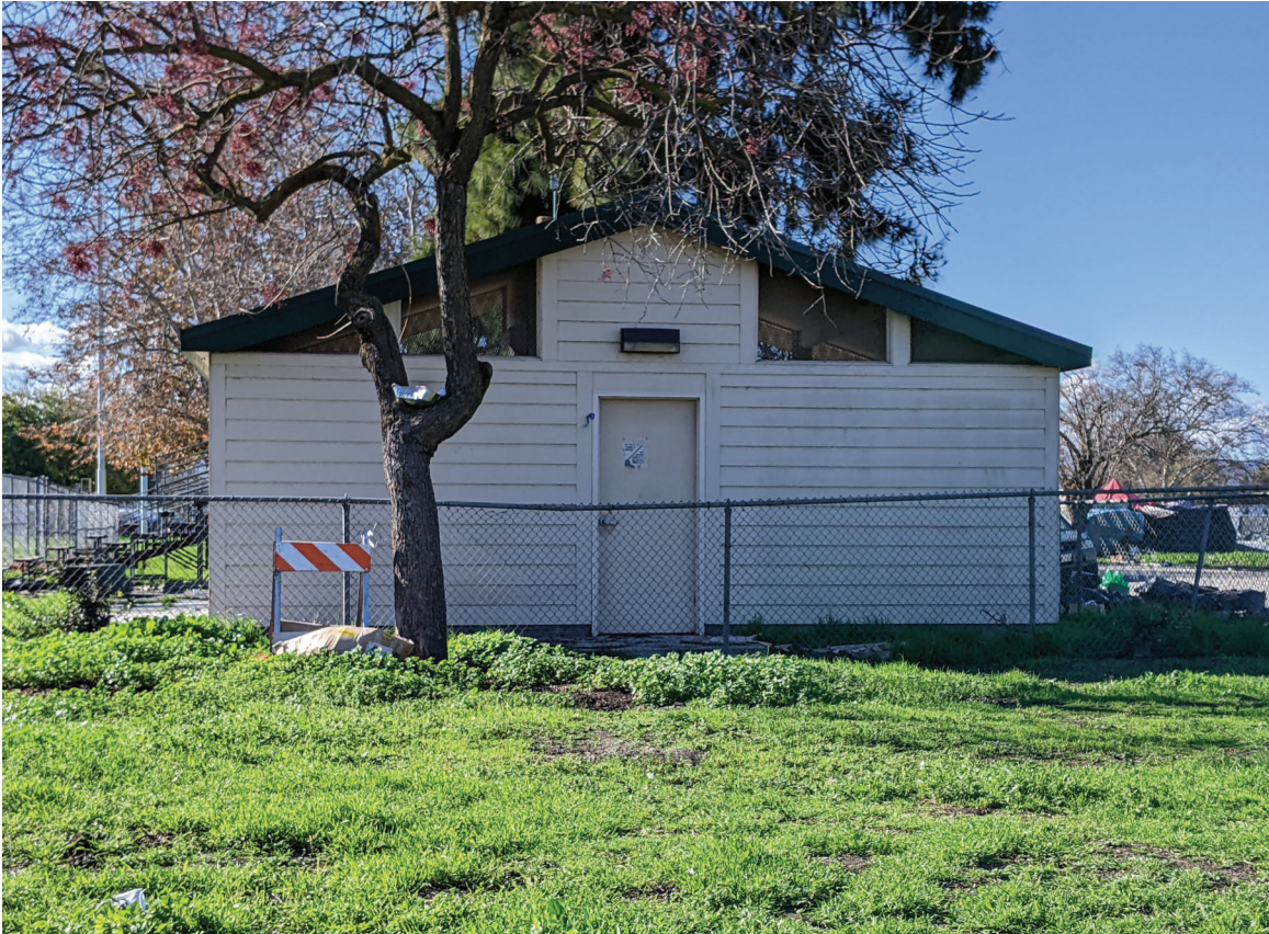
Photo 3: View of existing restroom building looking west from Irene Street.
