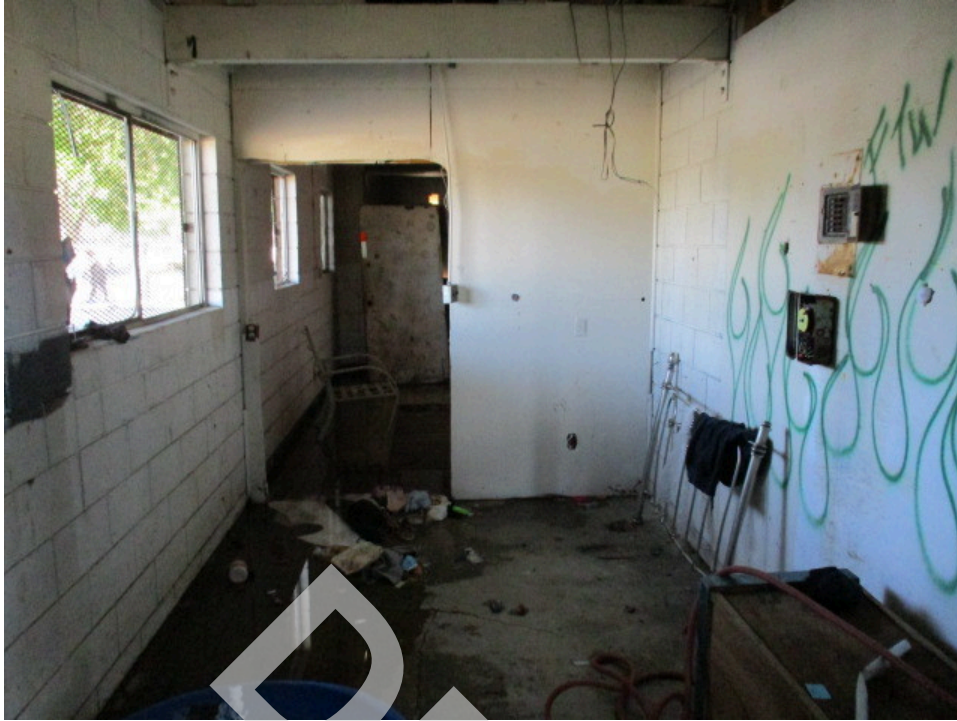
19. Restroom/equipment building on the southwestern side of the subject property
