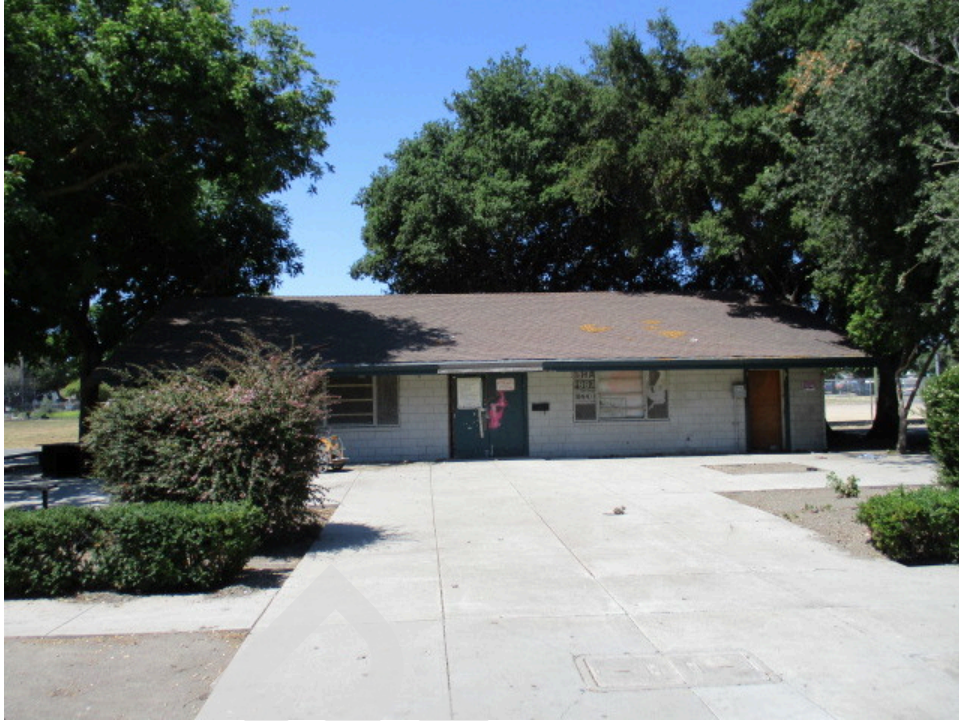
11. Restroom/equipment building on the southwestern side of the subject property
