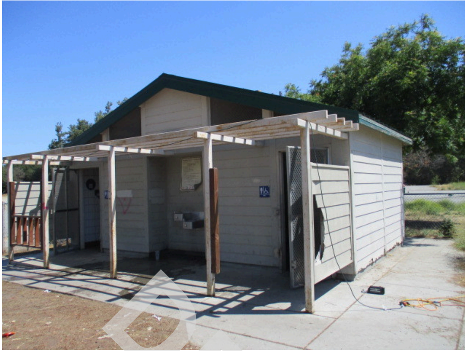
1. Restroom building on the northeastern side of the subject property
