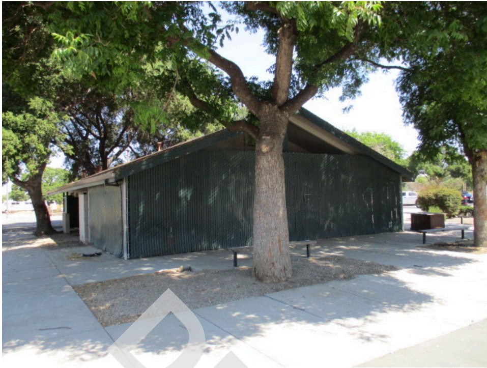
15. Restroom/equipment building on the southwestern side of the subject property
