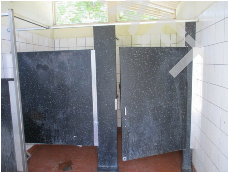
2. Restroom building on the northeastern side of the subject property
