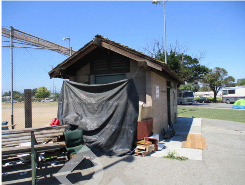
21. Equipment building on the southwestern side of the subject property
