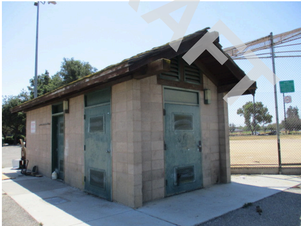
22. Equipment building on the southwestern side of the subject property
