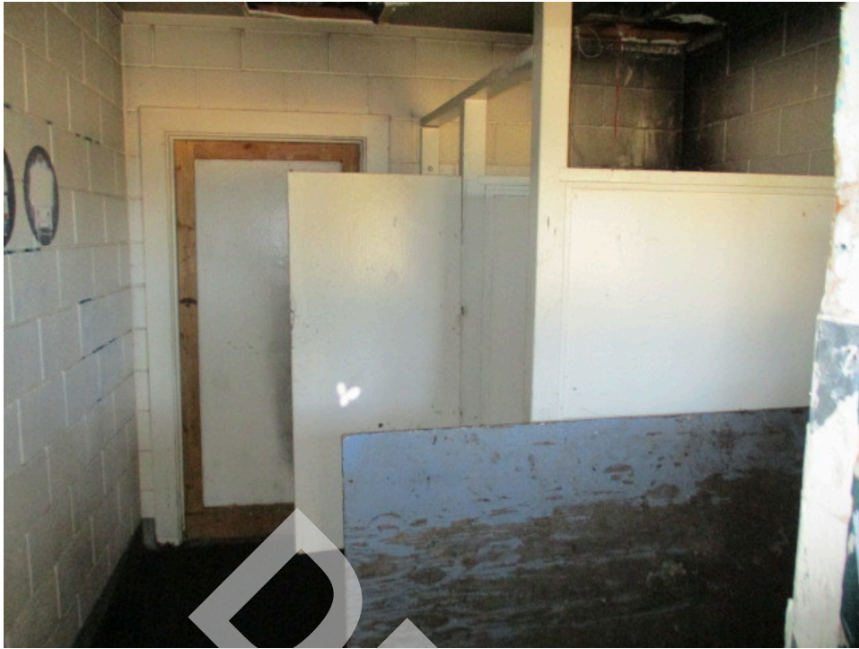
17. Restroom/equipment building on the southwestern side of the subject property
