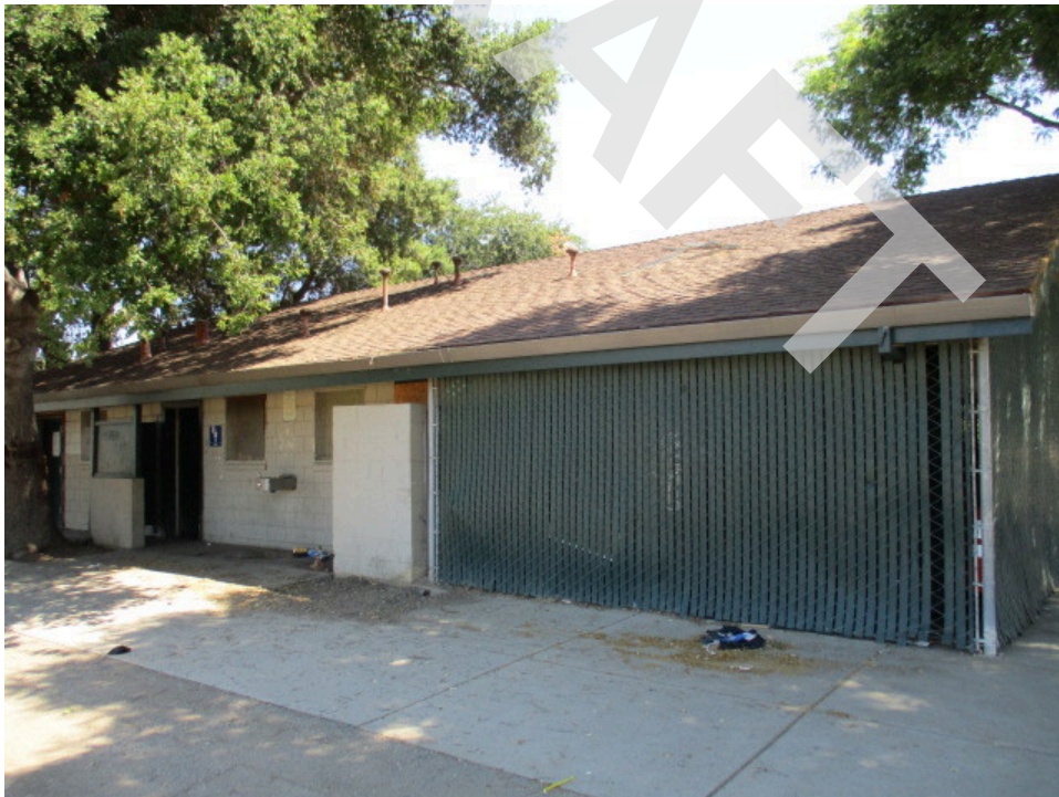
16. Restroom/equipment building on the southwestern side of the subject property
