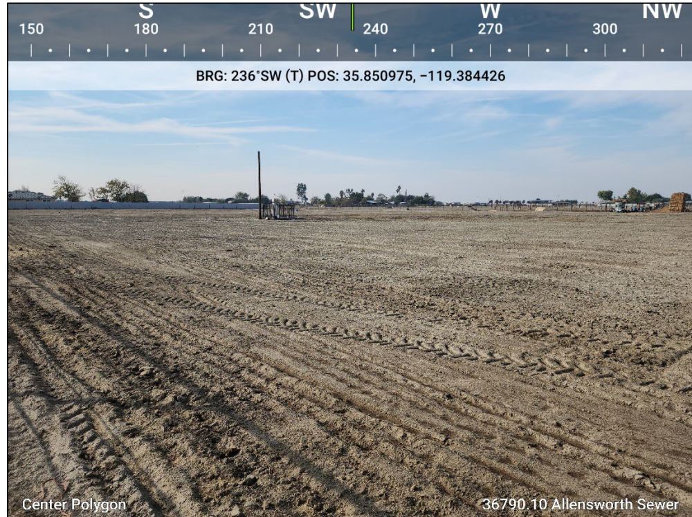
Figure 3. Central pumping station location, looking southwest.
