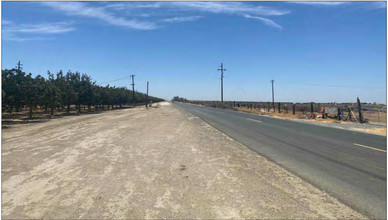
Figure 7. Photograph of a sewer line pathway along Avenue 24, showing orchard (left) and barren road shoulder.
