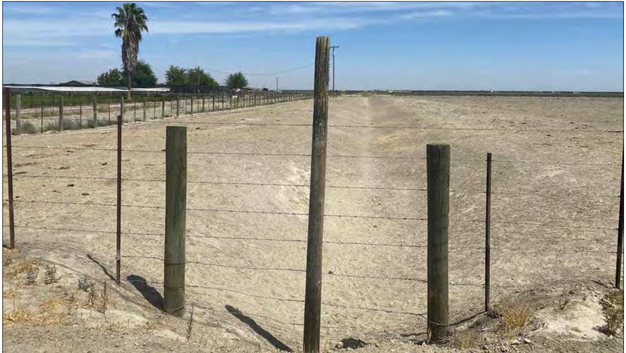
Figure 11. Photograph of a drainage ditch, oriented east-west, crossing Road 84 and the proposed sewer line pathway between Avenue 24 and Avenue 32.
