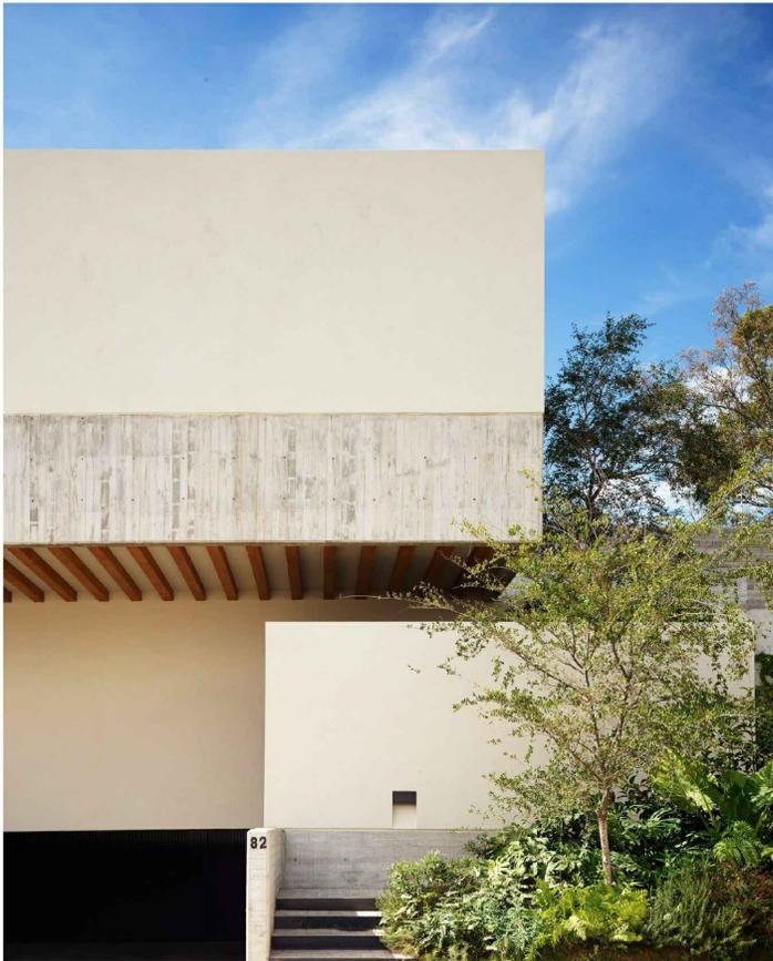
1. Smooth plaster, board-scored plaster, stained wood beams. Board-formed concrete, metal panels, metal fascia, metal roofing.
