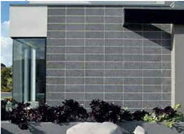
4. Concrete masonry unit blocks, tube steel, smooth plaster.
