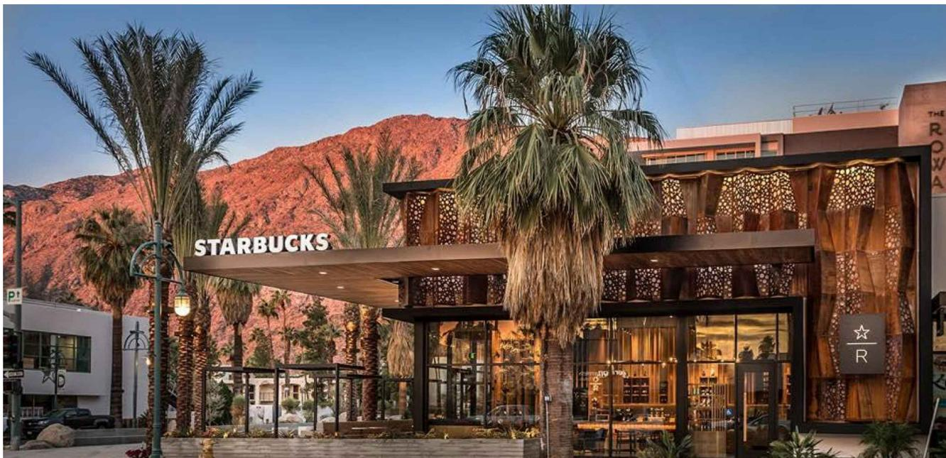
1. Board-formed concrete, metal panels, metal fascia, metal roofing.
