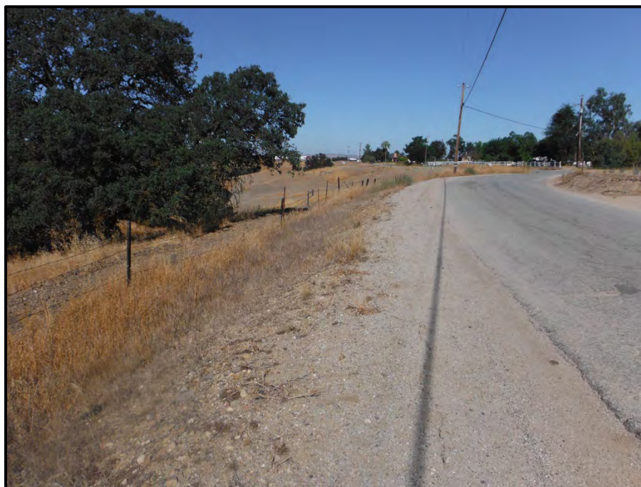
Figure 5-4. Overview of Dry Creek Road waterline route, facing west
