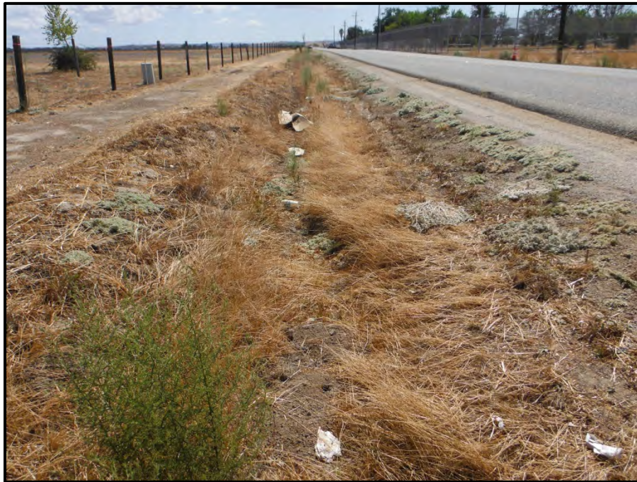
Figure 5-3. Overview of Airport Road sewer line route, facing south
