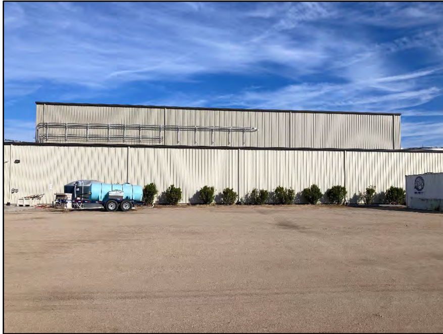
Photo 3. View north of disturbed land within survey area (November 11, 2022).
