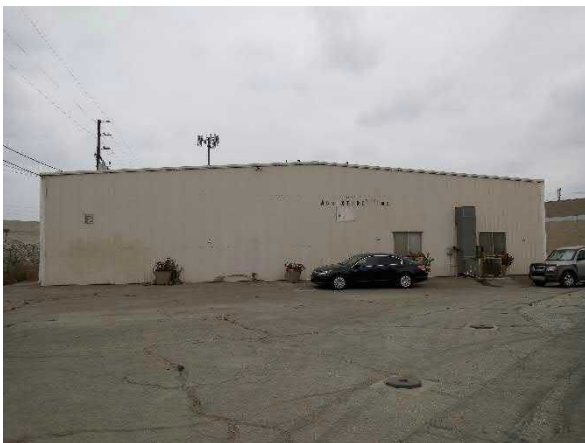
Photo #51 View of the Admixtures facility from Live Oak Lane.
