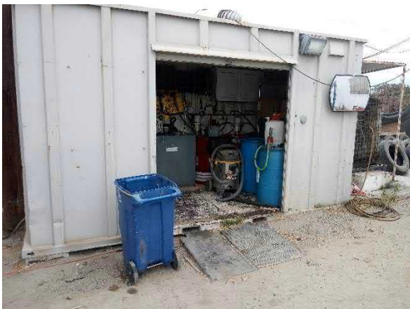
Photo #11 View of the hazardous material storage shed located on Lot 35.
