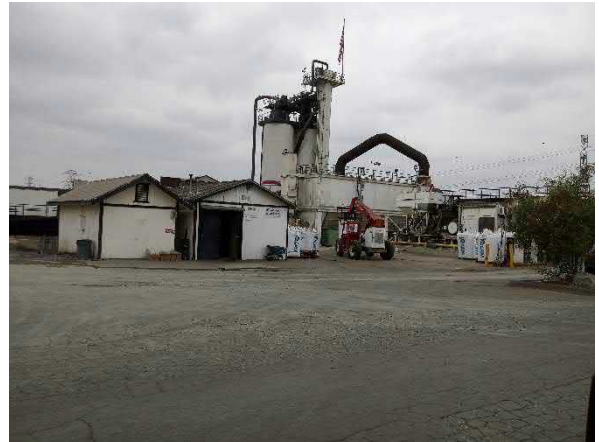
Photo #50 View of the American Asphalt facility from Live Oak Lane.
