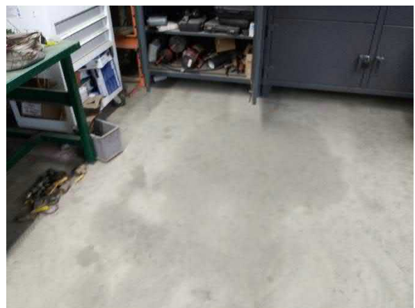
Photo #18 De minimis concrete staining located inside the maintenance garage on Lot 35.
