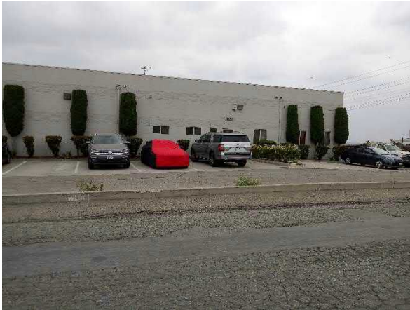
Photo #49 South facing view of the Capital Rebar facility from Live Oak Lane.
