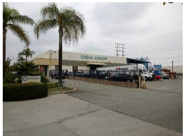
Photo #54 View of the Chem Arrow facility from Live Oak Lane.
