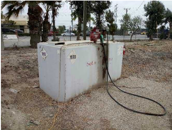
Photo #37 1000-gallon capacity AST containing diesel fuel located near the landfill entrance.
