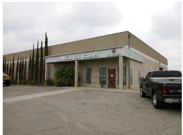
Photo #52 View of the Jonell Oil Corp. facility from Live Oak Lane.
