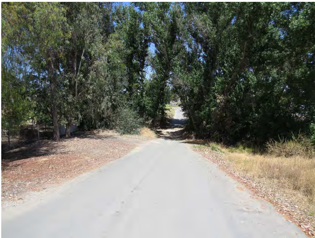
Photograph 28: Looking at the low water crossing associated with Monroe Avenue.
