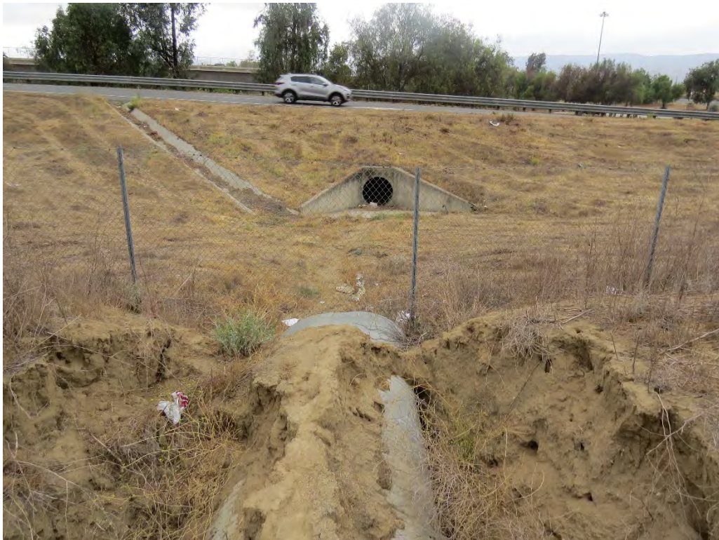
Photograph 18: Looking at the culvert that receives water flows from Drainage 2 and conveys water under Interstate 15.
