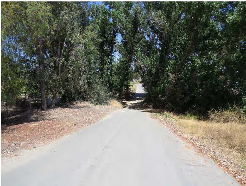
Photograph 18: Looking at the low water crossing associated with Monroe Avenue.
