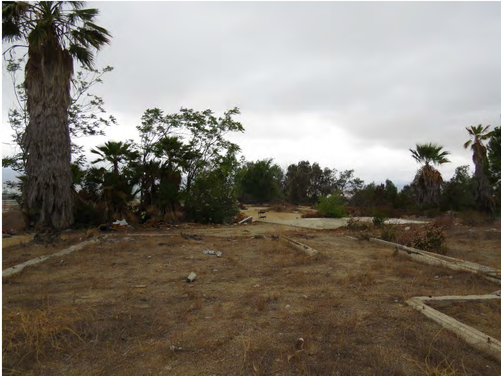
Photograph 3: Existing residential foundations on the northern portion of the site.
