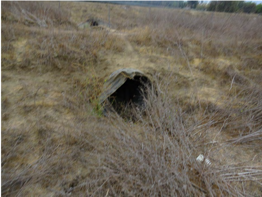
Photograph 17: 36-inch culvert that Drainage 2 flows into on the western boundary of the site.
