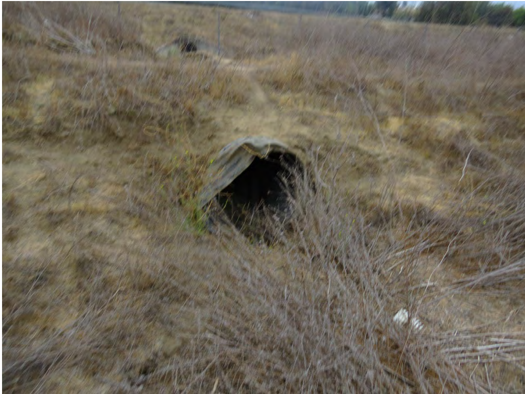
Photograph 8: 36-inch culvert that Drainage 2 flows into on the western boundary of the site.
