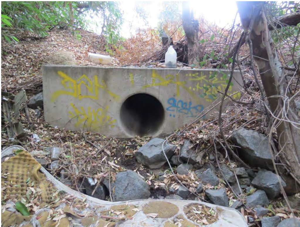
Photograph 21: One of the culverts that conveys flows into Drainage 1 on the southeast corner of the site.
