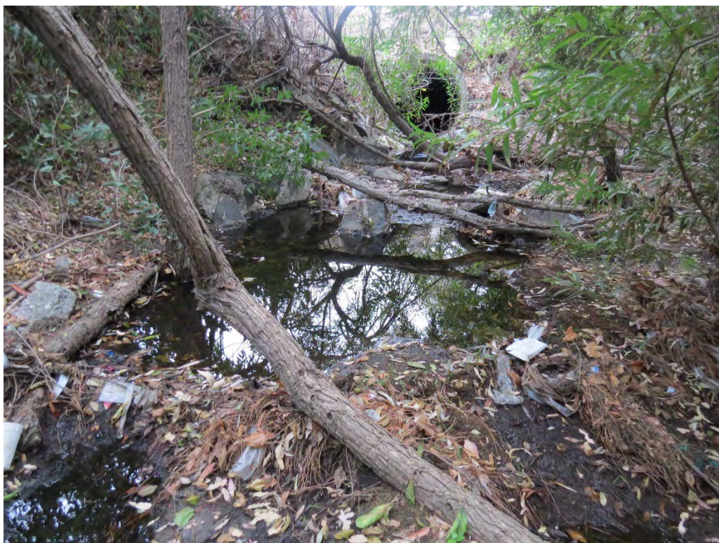
Photograph 20: From the eastern boundary of Drainage 1, looking at the area that is subject to urban runoff.
