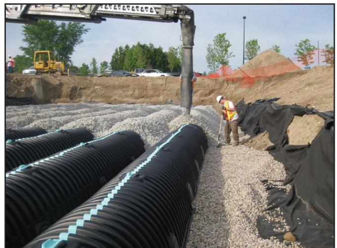
Do not allow equipment to drive over the chambers unless the minimum cover as shown in Table 6, page 20 is in place. Use a warning tape (available from CULTEC) to restrict access.
