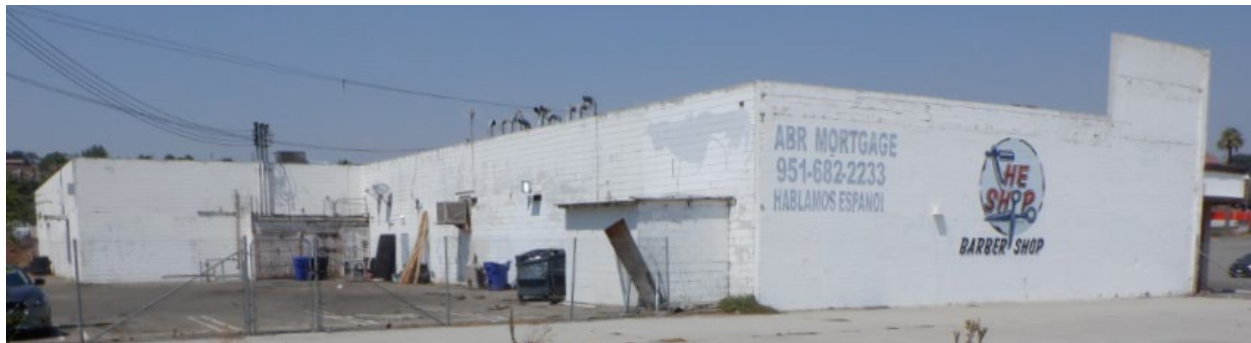
Photo 9. East and south elevations. View northwest. (Michael Baker International 9/7/2022)
