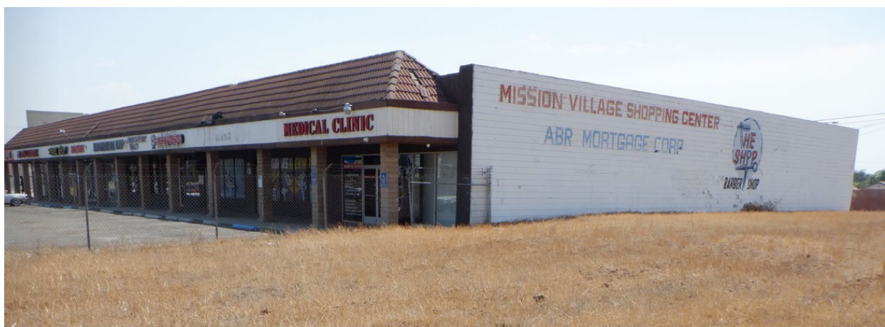
Photo 13. North and west elevations. View southeast. (Michael Baker International 9/7/2022)
