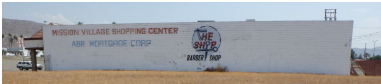
Photo 12. West elevation. View east. (Michael Baker International 9/7/2022)
