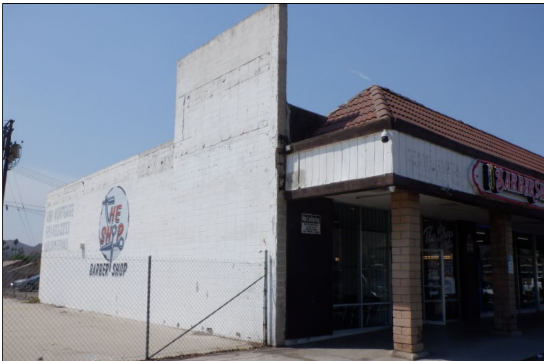
Photo 3. North and east elevations. View southwest. (Michael Baker International 9/7/2022)
