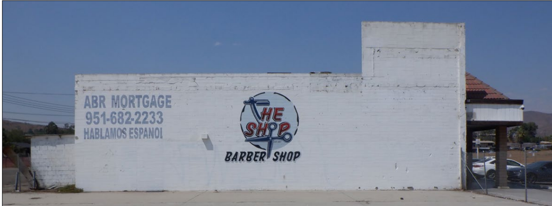
Photo 8. East elevation. View west. (Michael Baker International 9/7/2022)
