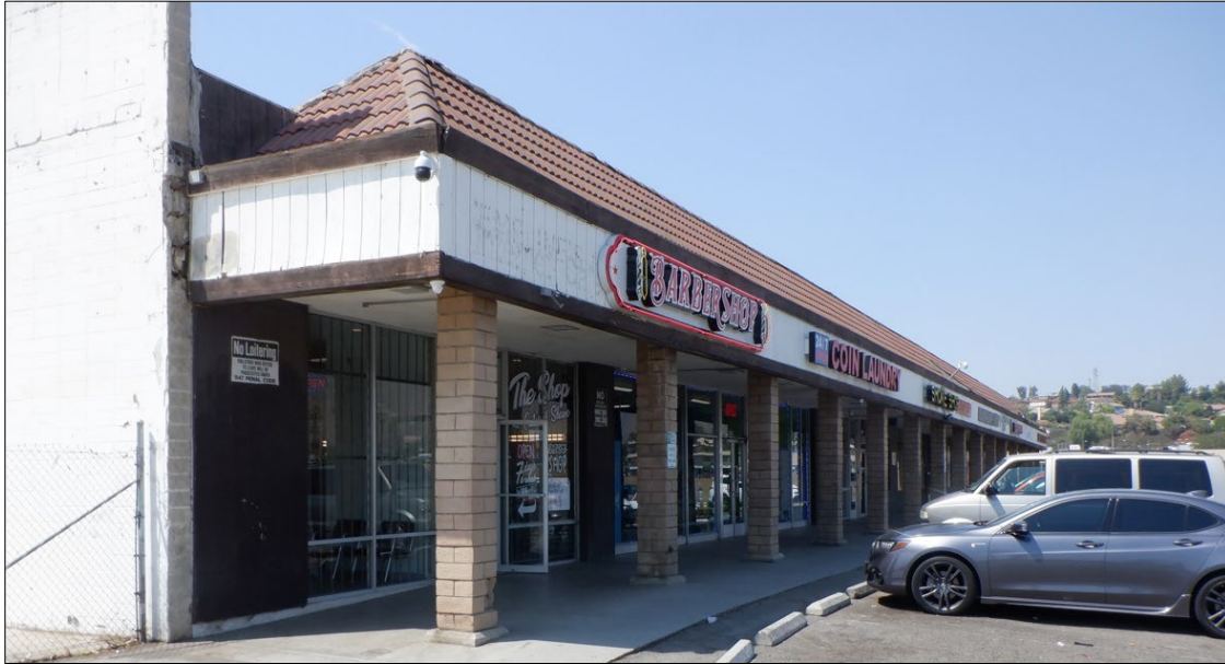
Photo 4. North and east elevations. View southwest. (Michael Baker International 9/7/2022)
