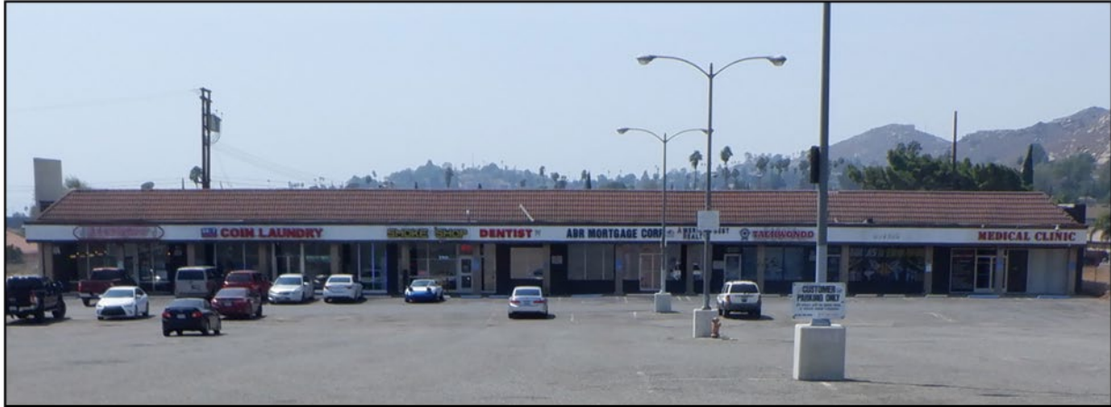
FIGURE 3 OVERVIEW OF 6322-6328 MISSION BOULEVARD STRIP MALL (FACING SOUTH)
