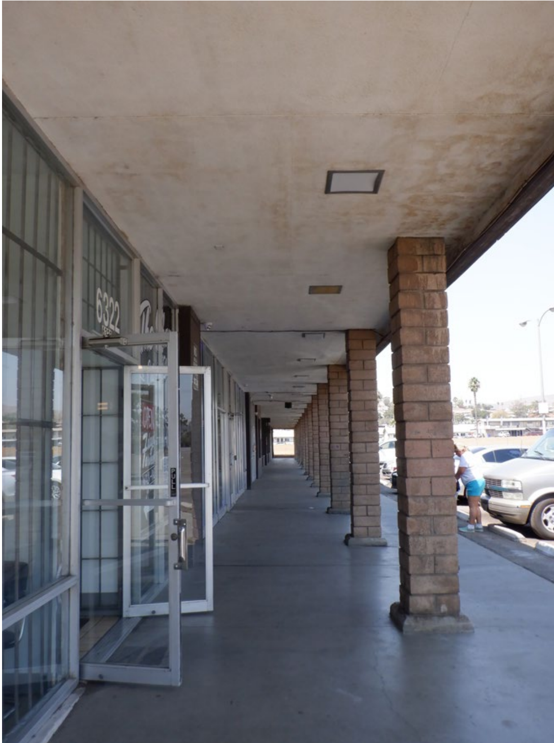
Photo 6. North elevation. View east. (Michael Baker International 9/7/2022)
