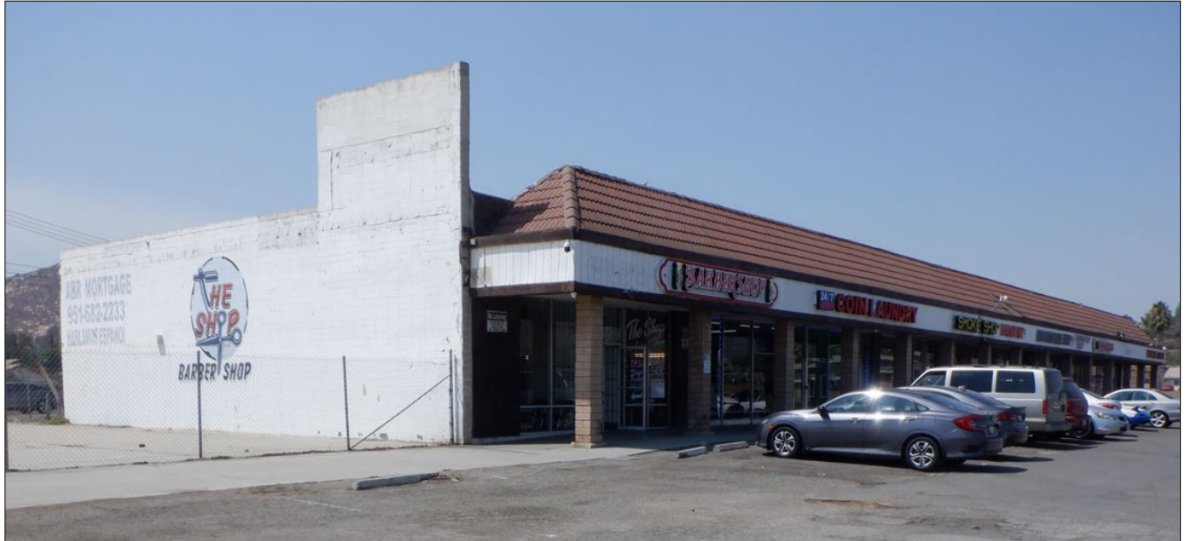
Photo 2. North and east elevations. View southwest. (Michael Baker International 9/7/2022)
