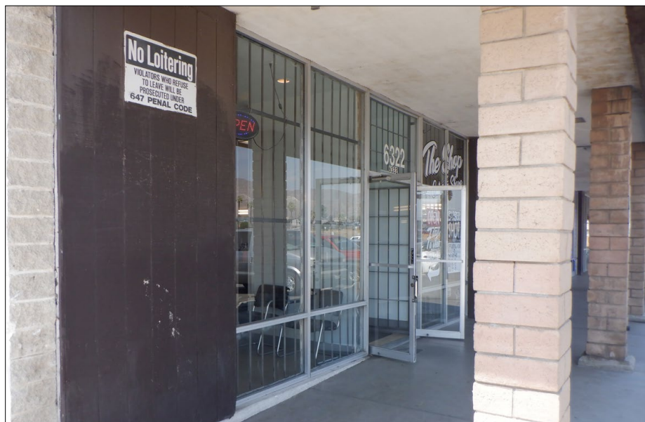
Photo 5. North elevation. View southwest. (Michael Baker International 9/7/2022)
