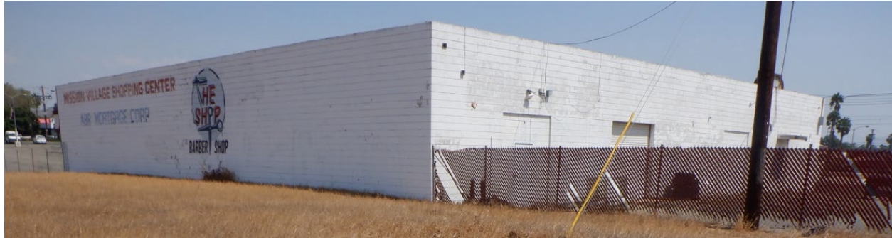
Photo 11. South and west elevations. View northeast. (Michael Baker International 9/7/2022)
