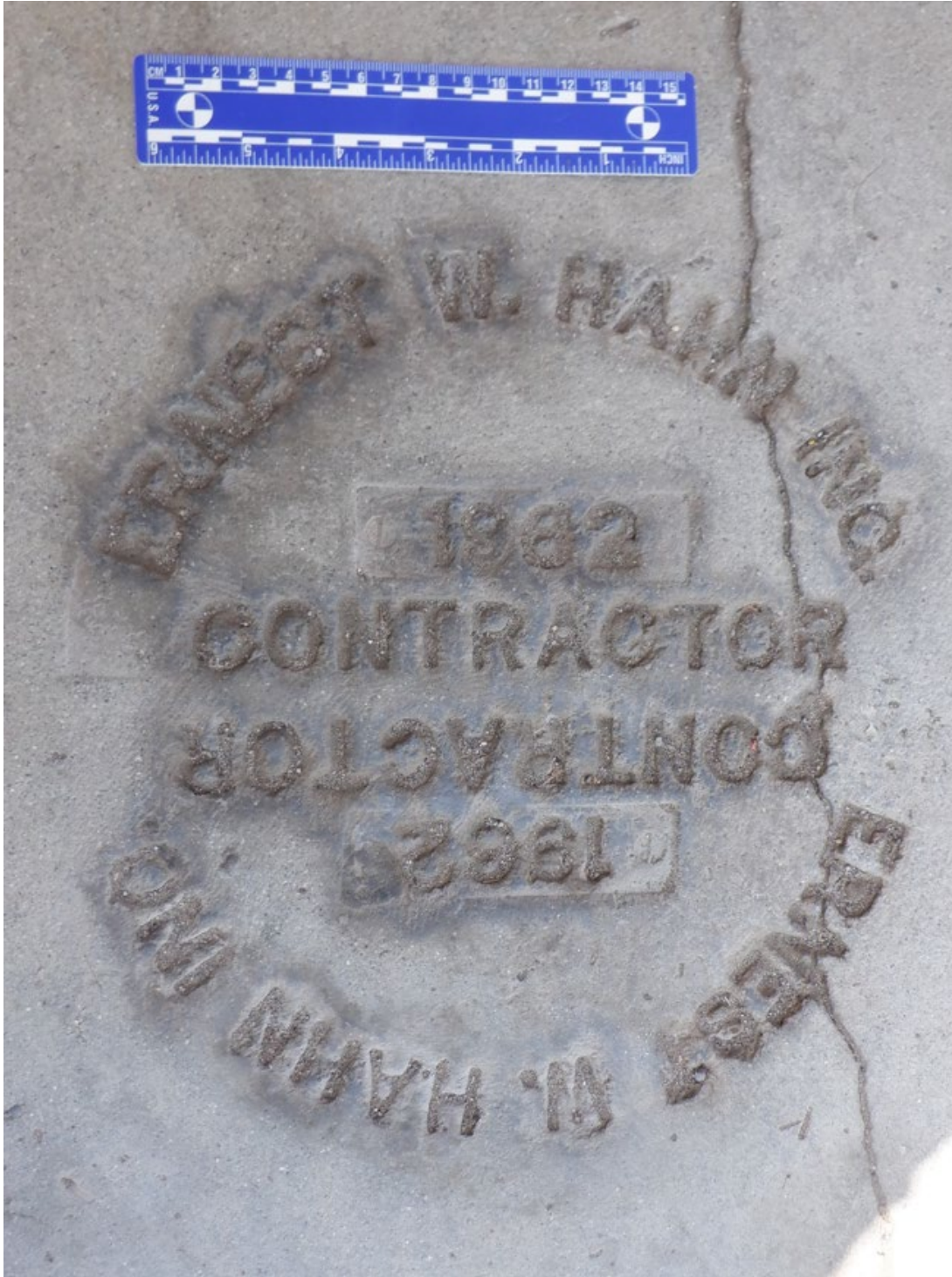
Photo 7. Contractor's stamp near northeast corner of the building. (Michael Baker International 9/7/2022)
