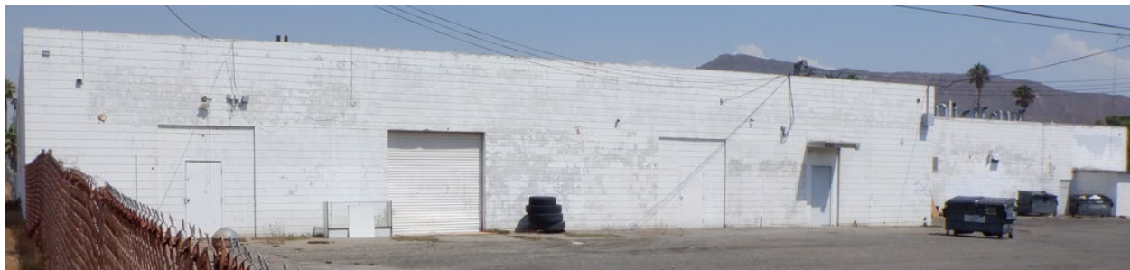
Photo 10. South elevation. View north. (Michael Baker International 9/7/2022)
