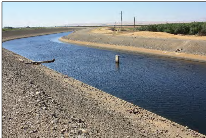
Photograph 304: View of Segment 15, showing a well discharge and remnants of a deleted pipe crossing at M.P. 78.31; camera facing downstream from left bank, June 14, 2022 (C0267).
