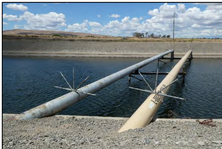
Photograph 99: Two oil utility crossings at M.P. 16.78; camera facing right bank from left bank, May 10, 2022 (B00009).
