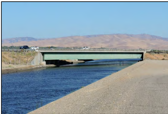
Photograph 301: Bridge at M.P. 72.80; camera facing upstream from left bank, June 14, 2022 (D0206).
