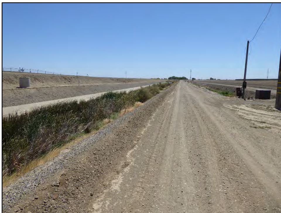
Photograph 7: Upstream view of Drain U-121.2 (right), San Luis Drain (left), and manhole tube (far left); camera facing southeast, July 20, 2022.
