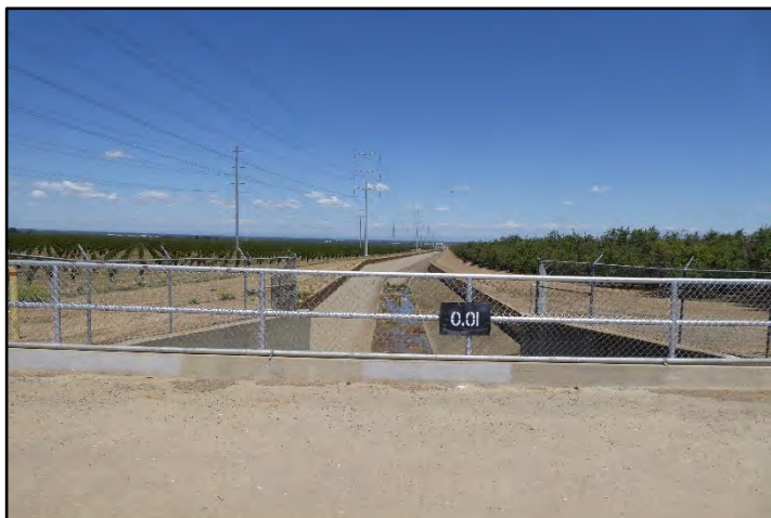
Photograph 190: View of beginning of concrete-lined chute of Westley Wasteway from inlet at M.P. 34.32; camera facing east from left bank, May 11, 2022 (A00710).
