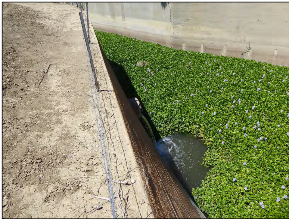
Photograph 6: Downstream view of Drain U-121.2 discharge point at Firebaugh Wasteway; camera facing southwest, July 20, 2022.
