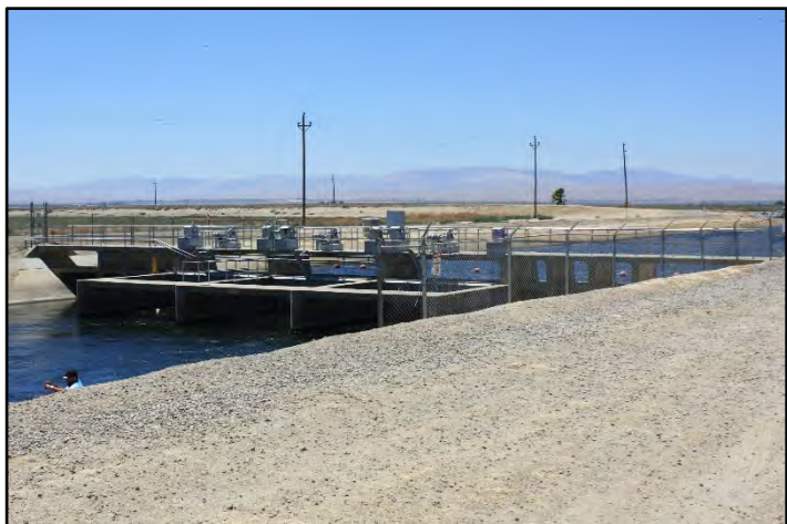
Photograph 344: Check No. 18; camera facing upstream from left bank, June 14, 2022 (C0412).
