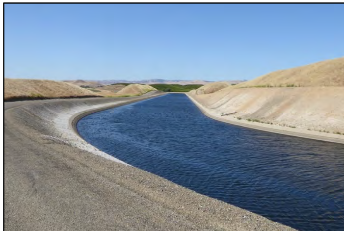
Photograph 247: View of deep excavations on the right bank of the DMC from approximately M.P. 50.00; camera facing downstream from left bank, May 13, 2022 (C20400).
