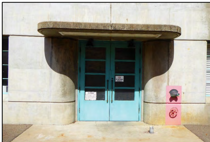
Photograph 119: Detail view of personnel door on east side of Pumping Station; camera facing west, May 9, 2022. (A00104)
