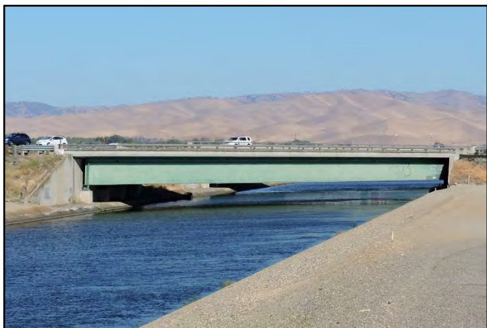
Photograph 90: View of non-original (post-1958) State Highway Bridge at M.P. 72.8, along Interstate 5 Westbound, 39-foot-8-inch-wide concrete deck on steel stringer strung directly between abutments; camera facing upstream from left bank, June 15, 2022 (D2206).
