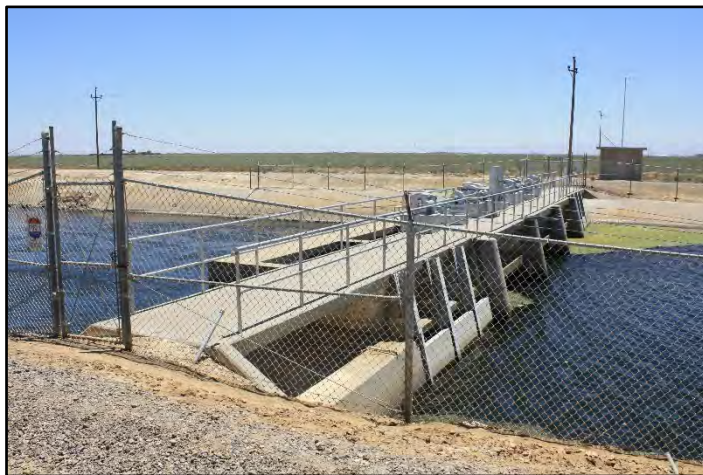
Photograph 343: Check No. 18; camera facing right bank from left bank, June 14, 2022 (C0413).
