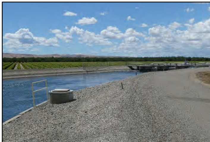
Photograph 167: View of stilling well, M.P. 20.69, and Check No. 3 outlet transition; camera facing upstream from left bank, May 10, 2020 (B00096.)
