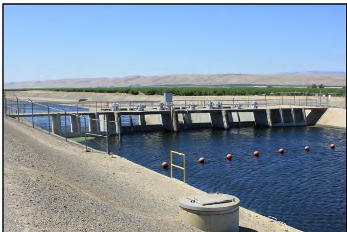
Photograph 328: Check No. 16 at M.P. 85.09; camera facing downstream from left bank, June 14, 2022 (C0333).
