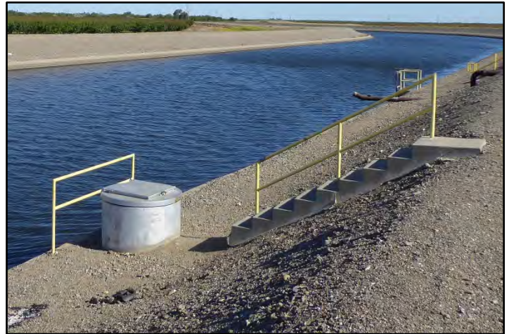
Photograph 30: View of stilling well, access hatch, and stairs to access the stilling well from the road; camera facing upstream from left bank, May 11, 2022 (A00482).
