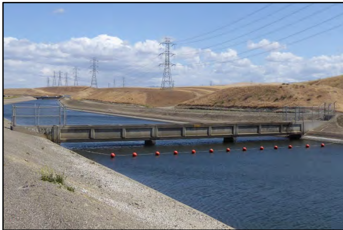
Photograph 41: Concrete overchute at M.P. 7.25 looking downstream; camera facing downstream from left bank, May 9, 2022 (A00253).
