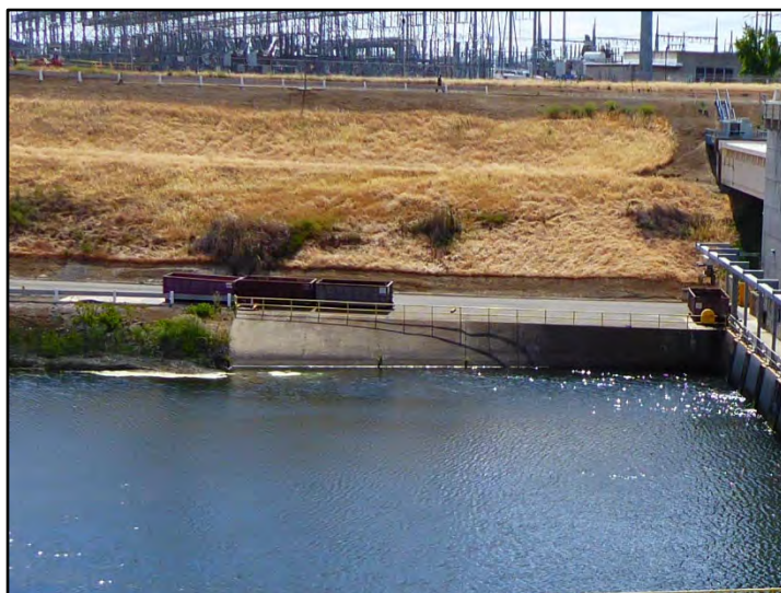
Photograph 5: End of earth lined Section No. 2 at the beginning of the Pumping Station inlet transition, at M.P. 2.52, which marks the end of the Intake Canal; camera facing left bank from right bank, May 9, 2022. (A00089)
