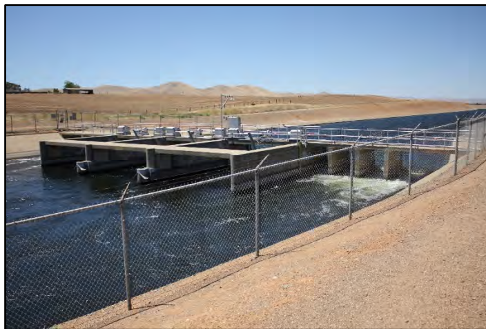
Photograph 286: Check No. 12; camera facing upstream from left bank, June 13, 2022 (C0147).
