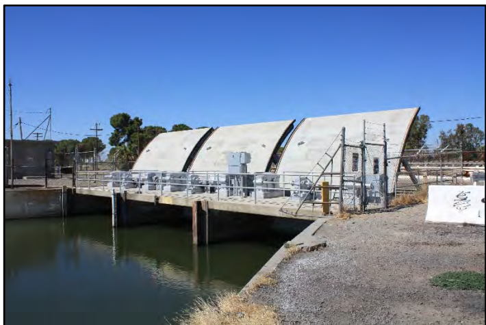
Photograph 370: Check No. 21, showing the radial gates fully open; camera facing upstream from left bank, June 15, 2022 (C0555).
