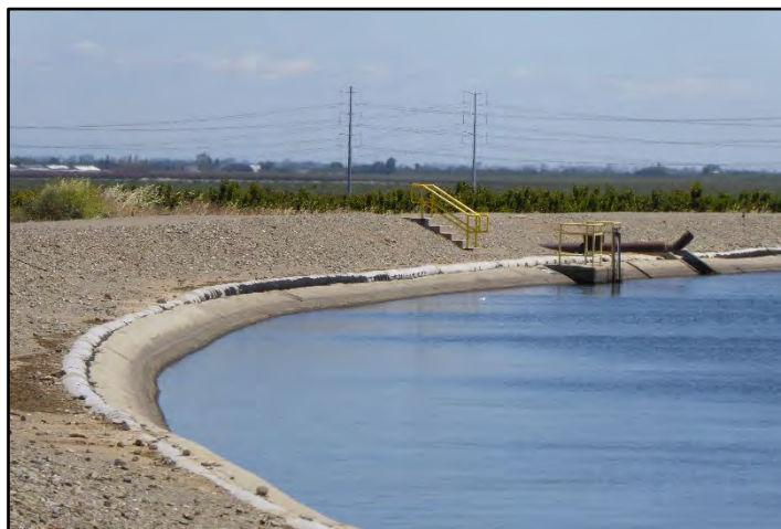
Photograph 201: View of sandbags lining the top of the concrete wall around features at M.P. 33.71; camera facing downstream from left bank, May 11, 2022 (A00694)
