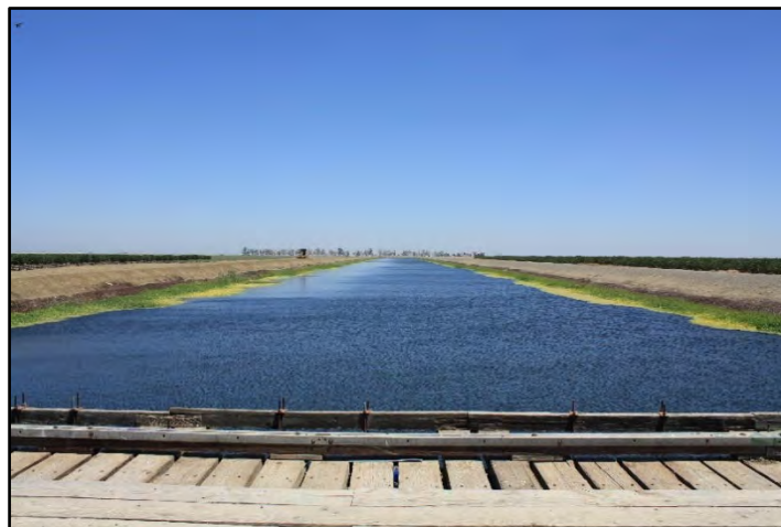
Photograph 11: View of compact-earth lined Section No. 10; camera facing downstream from Farm Bridge at M.P. 99.82, June 14, 2022 (C0430).
