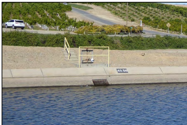
Photograph 33: Concrete pipe turnout along the right bank at M.P. 49.56, showing the original, manual gate-hoisting equipment; camera facing from left bank, May 13, 2022 (A00911).
