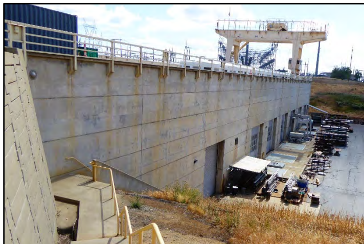
Photograph 111: South elevation of Pumping Station; camera facing east, May 9, 2022. (A00095)
