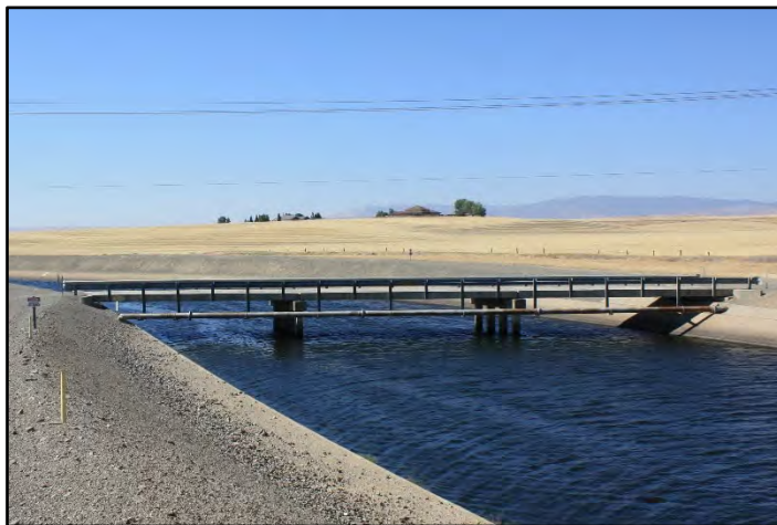
Photograph 312: Bridge at M.P. 77.20; camera facing downstream from left bank, June 14, 2022 (C0259).
