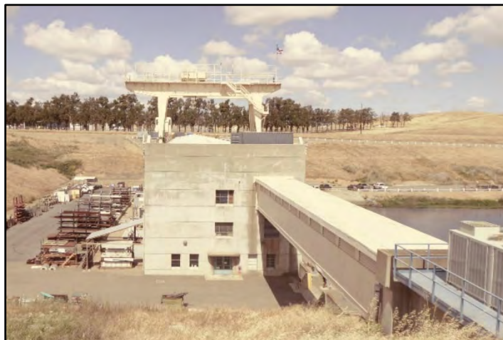
Photograph 113: East elevation of Pumping Station; camera facing west, May 9, 2022. (A00145)
