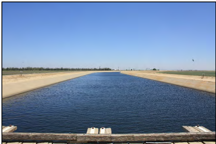
Photograph 333: View of Segment 18 from the deck of a farm bridge at M.P. 95.45; camera facing downstream, June 14, 2022 (C0398).
