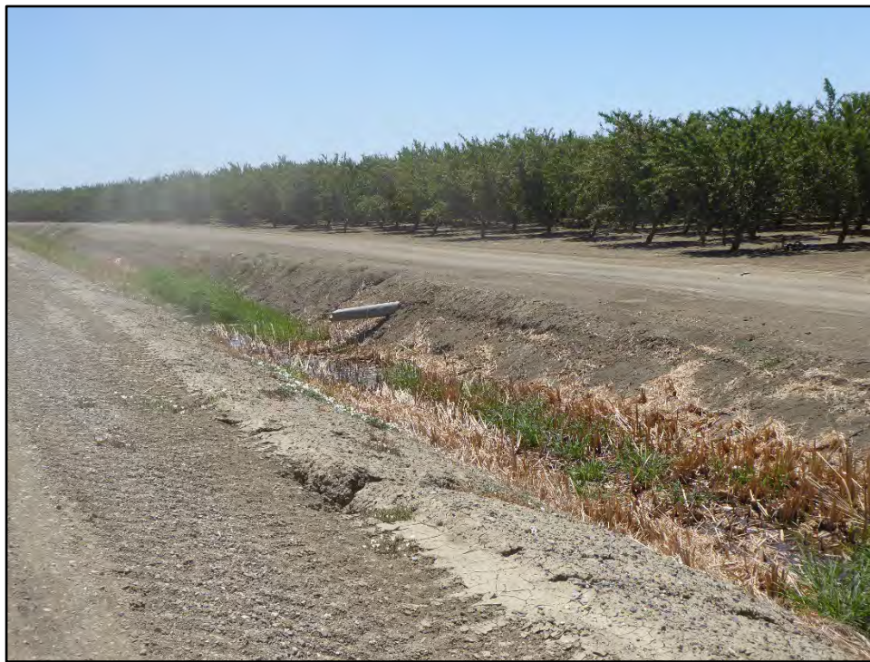
Photograph 10: Upstream view of Drain U-121.2 with extended subsurface inlet drain pipe; camera facing southeast, July 20, 2022.
