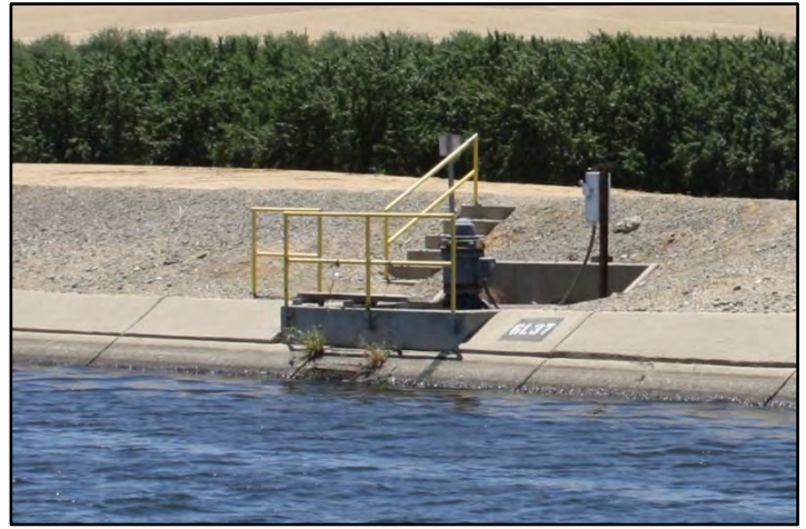
Photograph 36: Concrete pipe turnout altered by the addition of an automatic, electronic gate-operating system along the right bank at M.P. 61.37; camera facing from left bank, June 13, 2022 (C0118).
