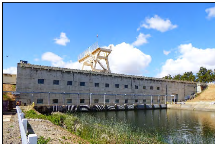
Photograph 109: View of water intake (north side) at C.W. Bill Jones Pumping Station; camera facing downstream from left bank, May 9, 2022. (A00106)
