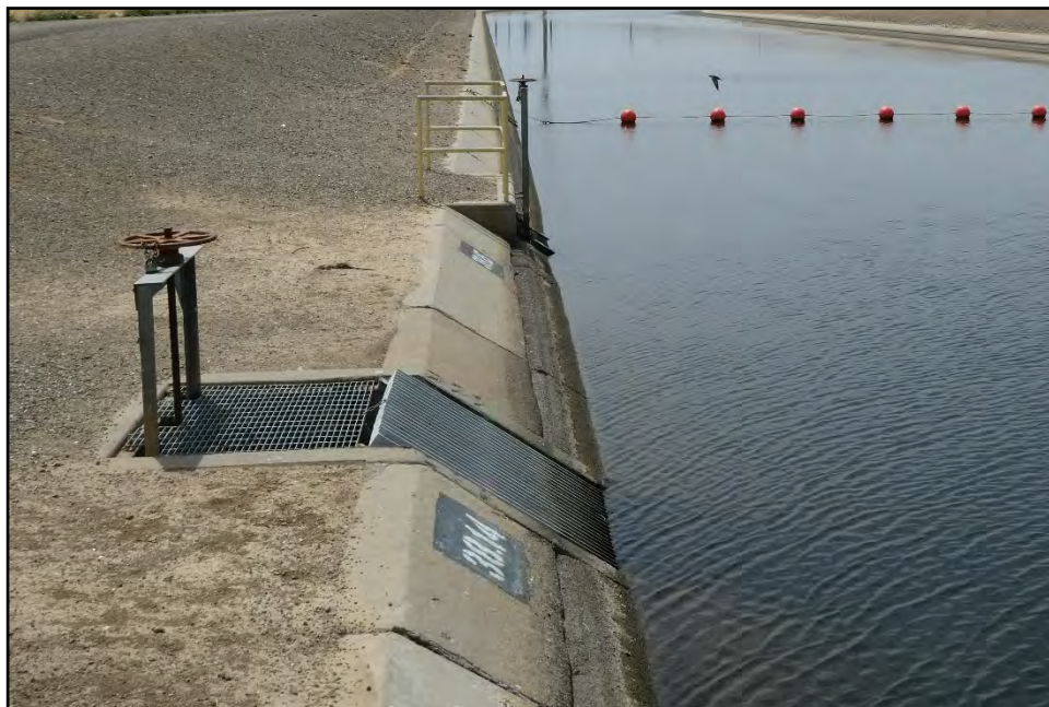
Figure 33: Two turnouts at M.P. 38.14; camera facing downstream from left bank, May 12, 2022.
