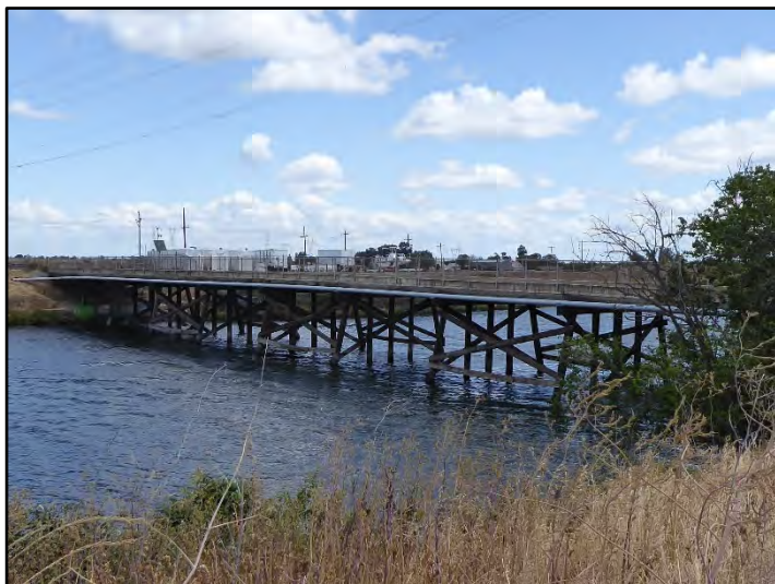
Photograph 64: View of County Highway Bridge with concrete deck supported by timber bents, at M.P. 0.33 along Lindemann Road, next to the Tracy Fish Facility; camera facing upstream from left bank, May 9, 2022 (A00158).
