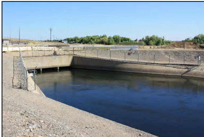
Photograph 19: 3-barrel siphon outlet at M.P. 79.72; camera facing upstream from right bank, June 14, 2022 (C0293).
