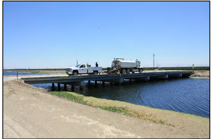
Photograph 73: View of 30-foot-wide Farm Bridge at M.P. 98.74, with replacement concrete deck supported by five replacement concrete bents, with no handrails; camera facing downstream from left bank, June 14, 2022 (C0422).
