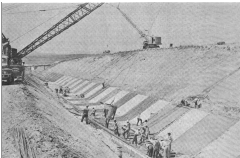
Figure 10: Placing alternate panels of reinforced concrete in Newman wasteway, April 1951. 75
