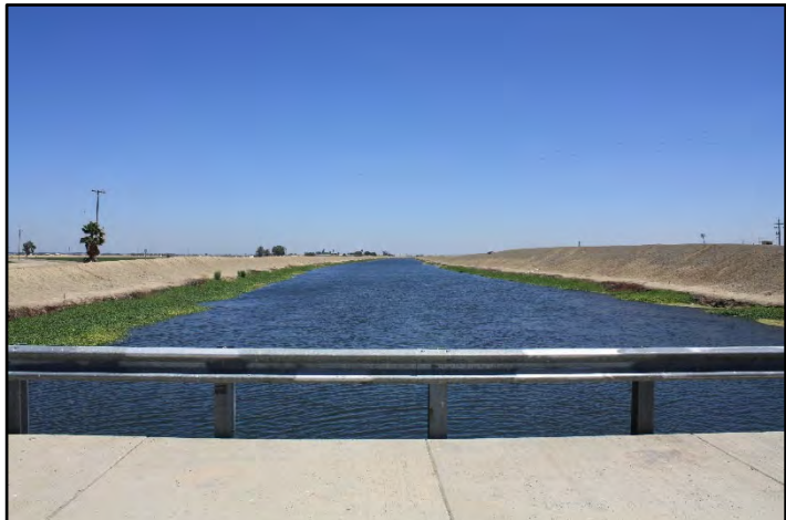
Photograph 347: View of Segment 20 from the deck of the bridge at M.P. 106.58 Check No. 19; camera facing downstream, June 14, 2022 (C0462).
