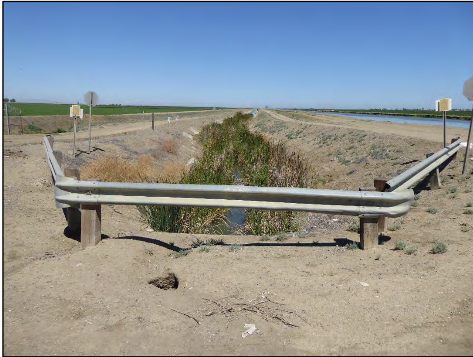
Photograph 3: Downstream view of San Luis Drain from north side of W. Nees Ave.; camera facing northwest, July 20, 2022.
