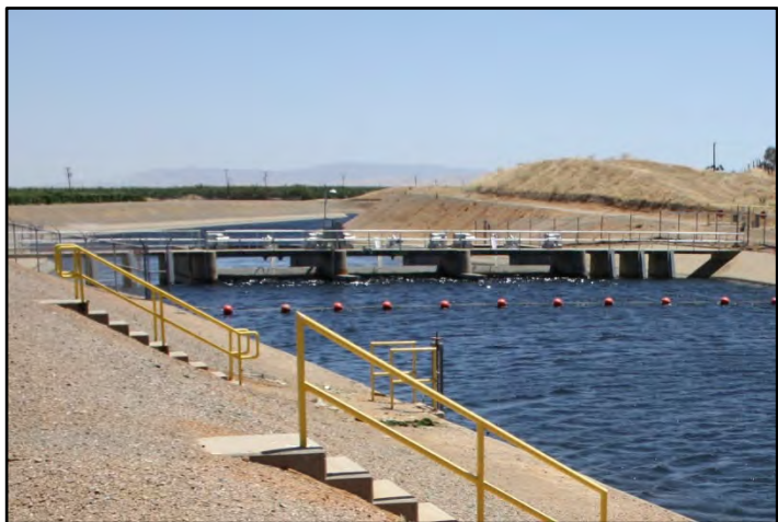
Photograph 285: Check No. 12, with a turnout at M.P. 63.96 visible in the foreground; camera facing downstream from left bank, June 13, 2022 (C0142).
