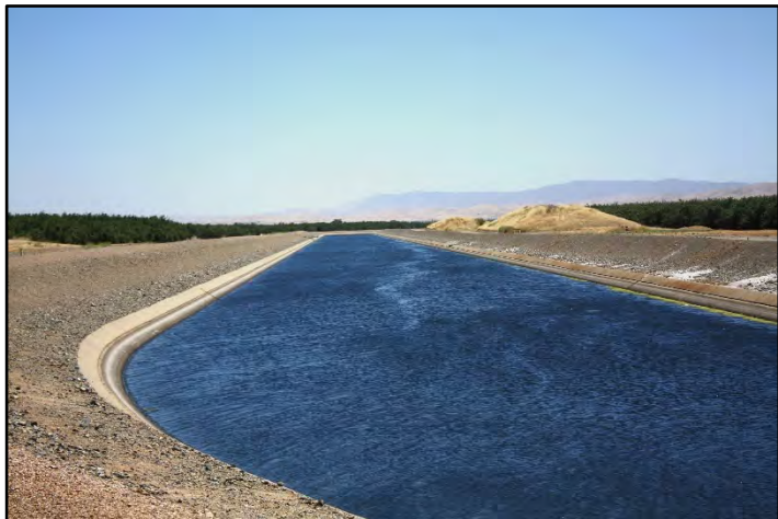
Photograph 283: View of Segment 13 from approximately M.P. 64.44, with spoils piles along the right bank; camera facing downstream from left bank, June 13, 2022 (C0158).
