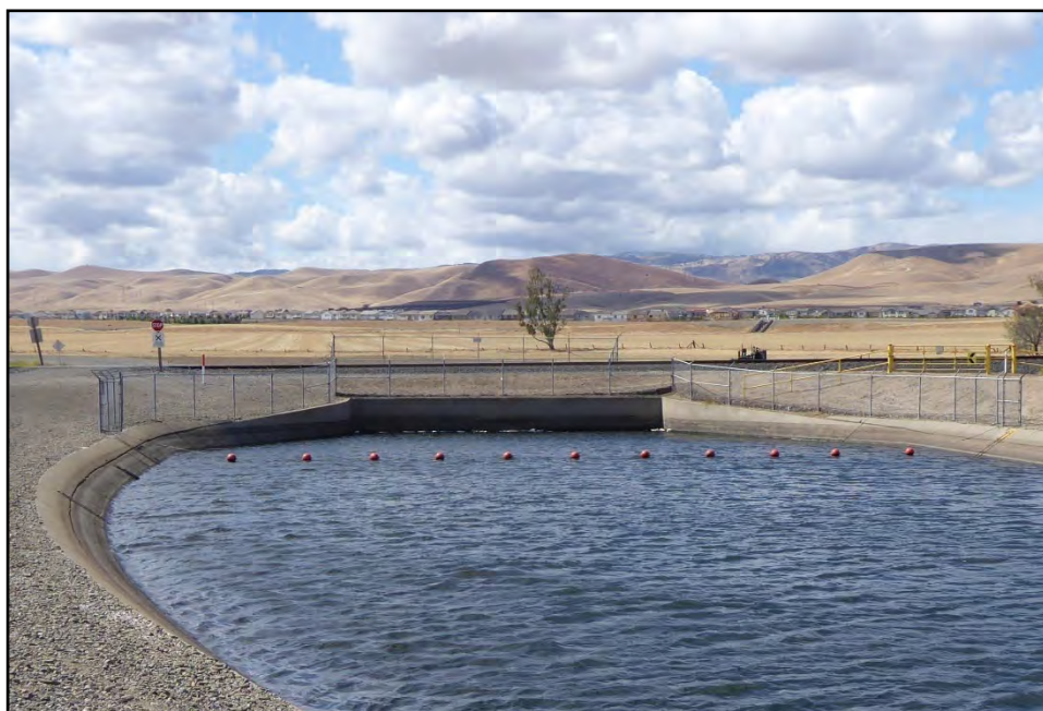
Figure 26: Three-barrel siphon inlet headwall at M.P. 13.67; camera facing downstream from left bank, May 10, 2022.
