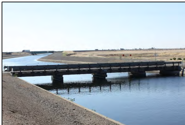
Photograph 61: View of County Highway Bridge with timber deck supported by three concrete piers at M.P. 72.33 along Hilldale Avenue; camera facing downstream from left bank, June 14, 2022 (C0243).
