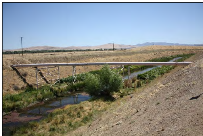
Photograph 291: View of Volta Wasteway with a pipe crossing at approximately M.P. 1.5; camera facing upstream from wasteway's left bank, June 13, 2022 (C0225).
