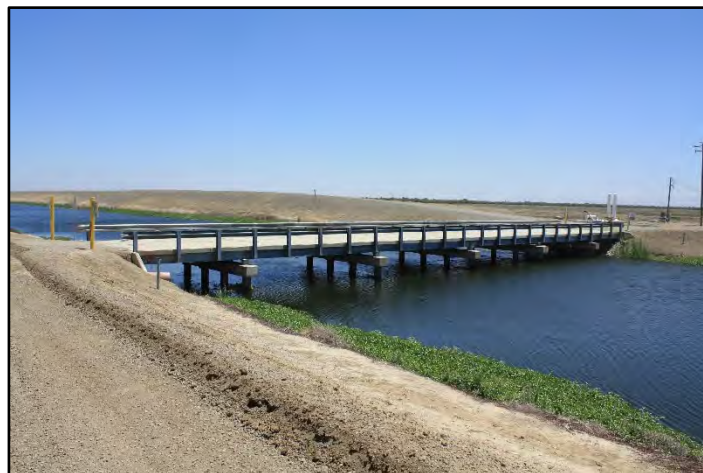
Photograph 345: Bridge at M.P. 102.03; camera facing downstream from left bank, June 14, 2022 (C0440).
