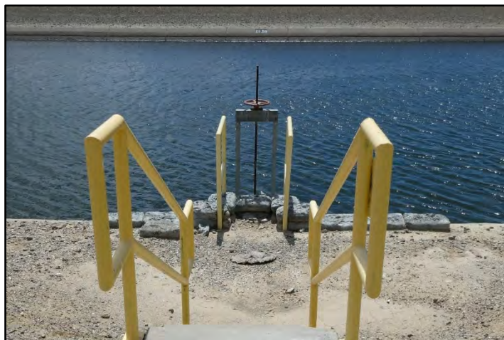
Photograph 160: View of sandbags lining the top of the canal wall at a turnout on the left bank at M.P. 20.59; camera facing right bank from left bank, May 10, 2022. (B00085)
