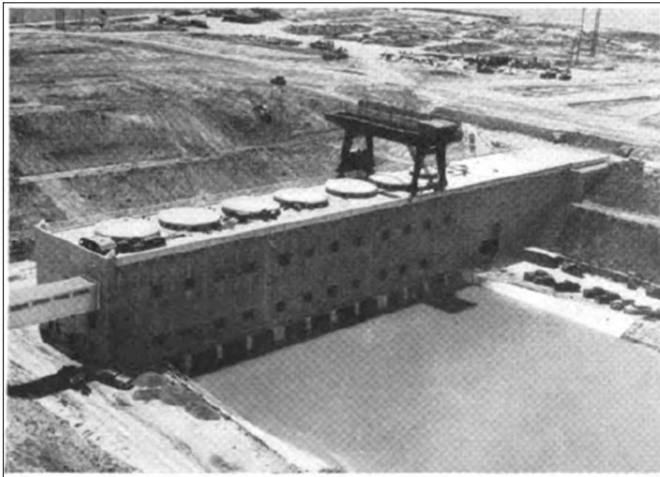
Figure 6: Tracy Pumping Plant, January 1951. 69
