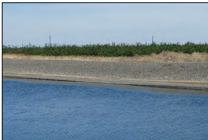
Photograph 233: Subsidence on right bank around M.P. 42.30; camera facing right bank from left bank, May 12, 2022 (B00417).
