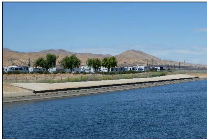
Photograph 227: Concrete overspill apron wasteway at M.P. 39.32/39.42 on the right bank, the only one of its type on the DMC; camera facing upstream from left bank; May 12, 2022 (B00342).
