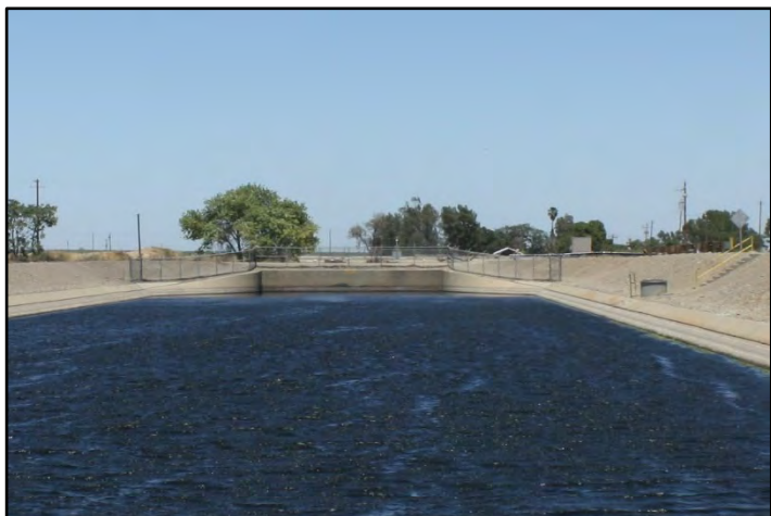
Photograph 279: Garzas Creek Siphon's outlet headwall from the deck of Gravel Pit Road bridge at M.P. 58.46; camera facing upstream, June 13, 2022 (C0080).
