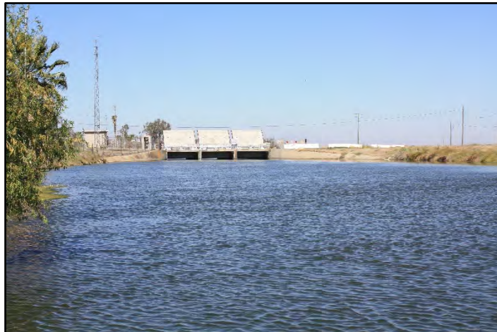
Photograph 369: View of Segment 22 from approximately M.P. 116.55, with Check No. 21 in the background; camera facing upstream from right bank, June 15, 2022 (C0538).
