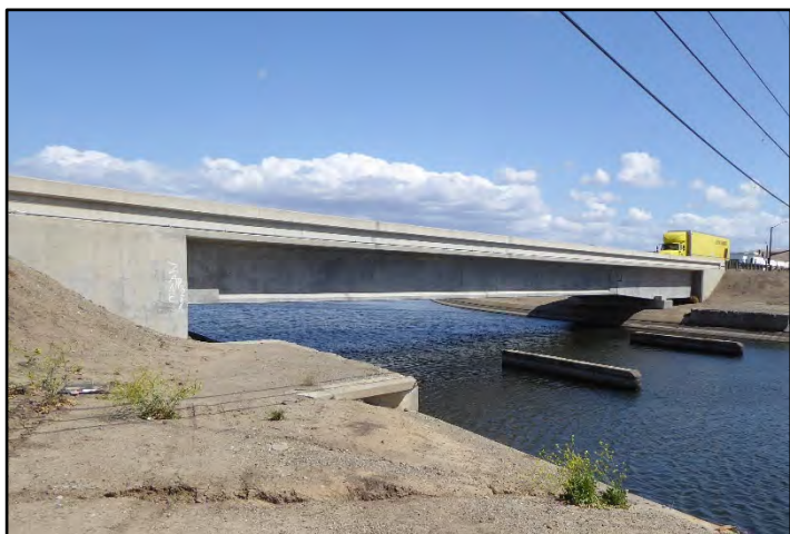
Photograph 86: View of replacement County Highway Bridge at M.P. 9.29, along International Parkway, with 30-foot-wide concrete deck, original piers and abutments visible just upstream of current bridge; camera facing downstream from left bank, May 9, 2022 (A00287).
