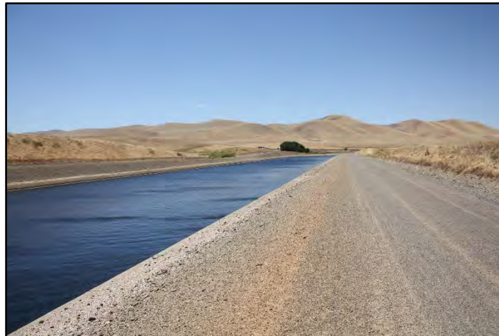
Photograph 274: View of Segment 12 from approximately M.P. 63.34; camera facing upstream from left bank, June 13, 2022 (C0135).
