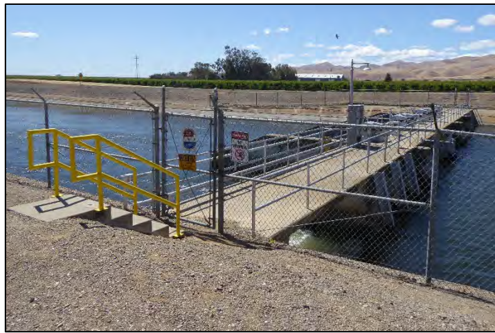
Photograph 185: Detail view of Check No. 5 deck, camera facing right bank from left bank, May 11, 2022 (A00606).
