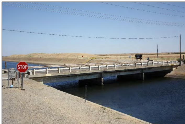
Photograph 83: View of State Highway Bridge at M.P. 71.31 along Jensen Road / State Route 207, with original steel guard-railing; camera facing downstream from left bank, June 13, 2022 (C0210).
