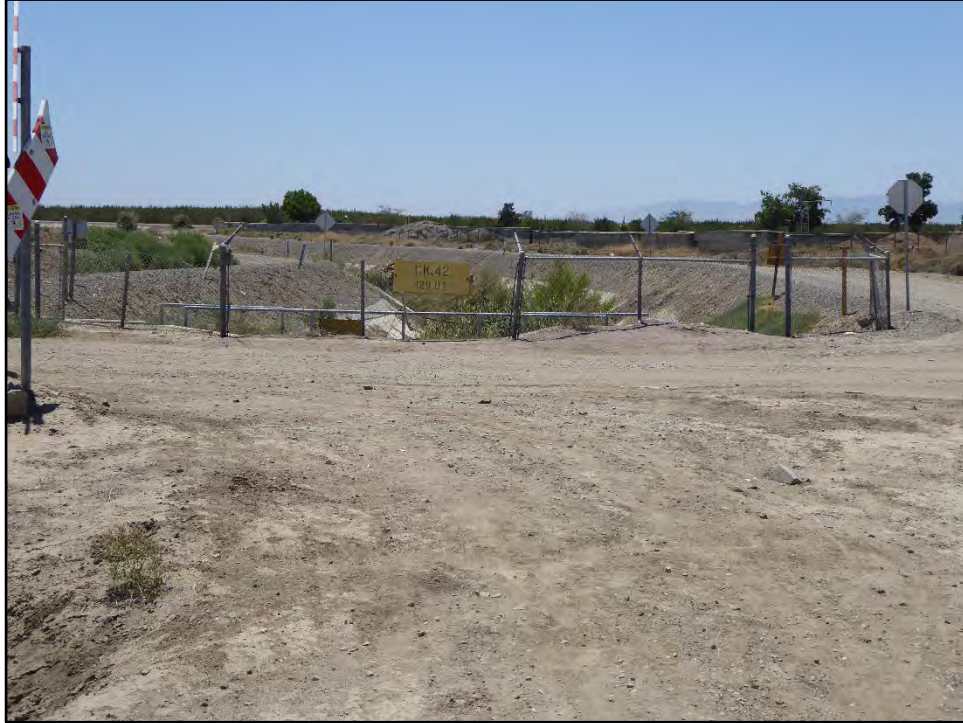
Photograph 14: Upstream view of San Luis Drain from south side of West Belmont Avenue, with Check Structure 42 (M.P. 129.07); camera facing south, July 20, 2022.
