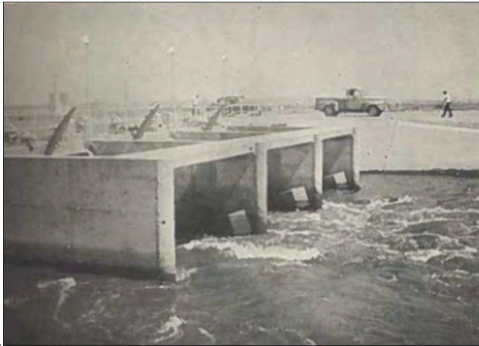
Figure 18: Note rough silty water below gates at Check No. 19, May 16, 1970. 100
