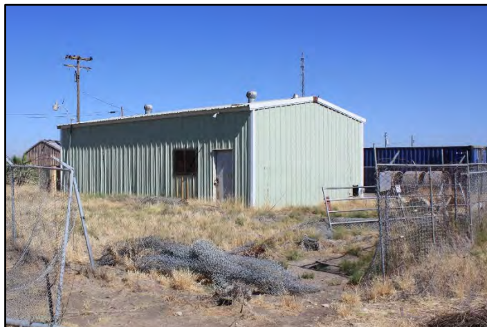
Photograph 375: South and east sides of storage building; camera facing northwest, June 15, 2022 (C0545).
