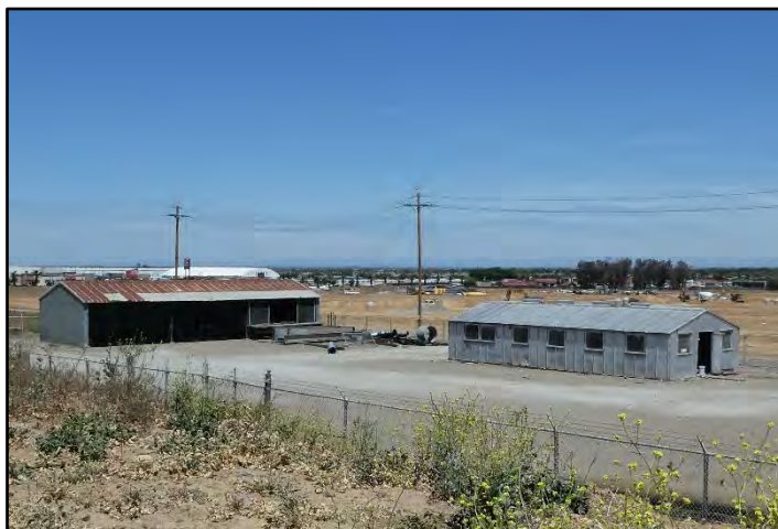
Photograph 225: Patterson O&M storage yard at M.P. 40.00 where buildings are no longer in use and have suffered heavy deterioration; camera facing southwest, May 12, 2022 (B00368).
