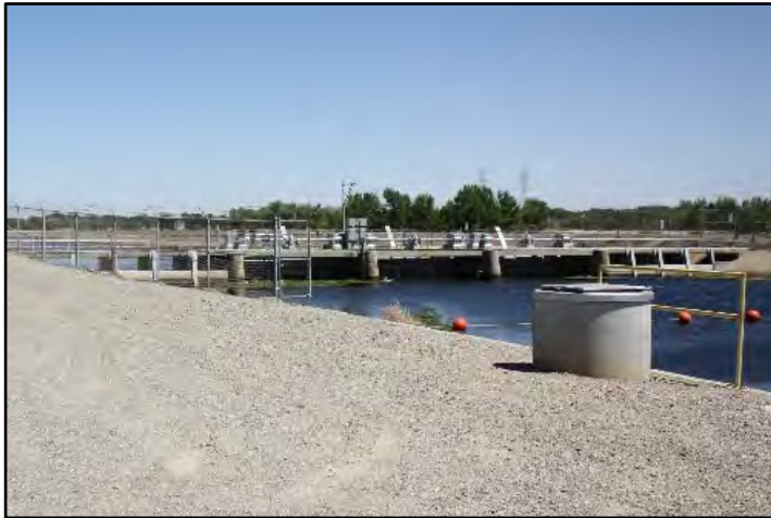
Photograph 29: View of stilling well upstream of Check No; camera facing downstream from left bank June 13, 2022 (C0200).
