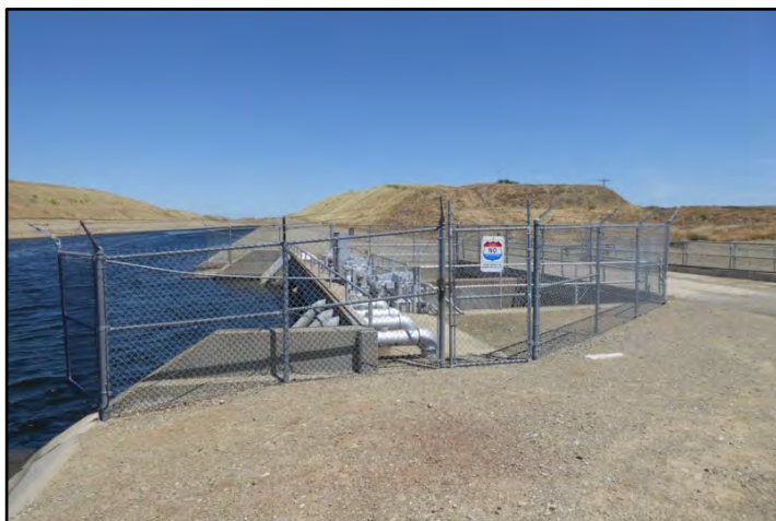
Photograph 256: View of Newman Wasteway inlet structure, looking upstream; camera facing downstream from left bank, May 13, 2022 (A00994).
