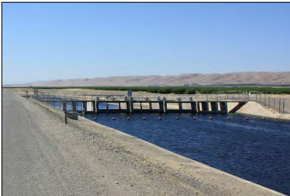
Figure 28: Check No. 16 at M.P. 85.09; camera facing downstream from left bank, June 14, 2022.
