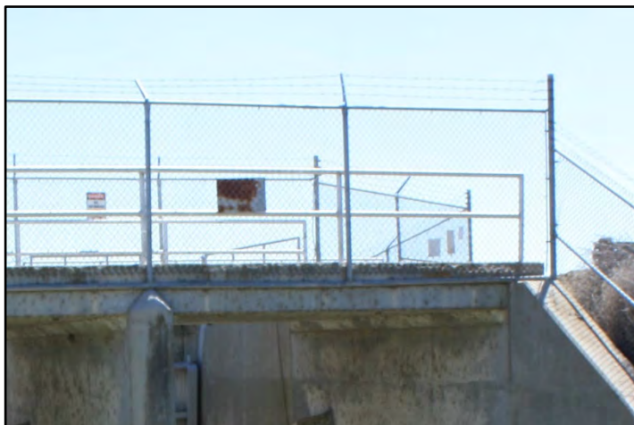
Photograph 60: View of chain-link fence and metal-pipe handrails on Firebaugh Wasteway bridge at M.P. 111.22, as well as central pier and left abutment/wall of forebay; camera facing southwest, June 14, 2022 (C0485).
