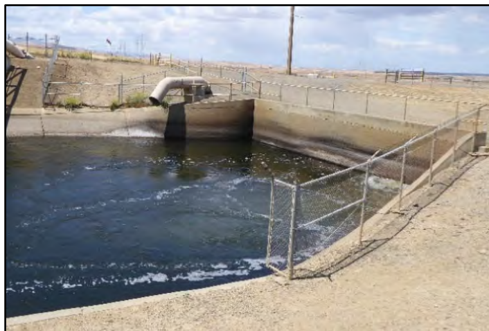
Photograph 7: Beginning of concrete-lined Section No. 3 at discharge pipes inlet to DMC at M.P. 3.50, raised lining visible at top of canal walls; camera facing west from left bank, May 9, 2022 (A00199).
