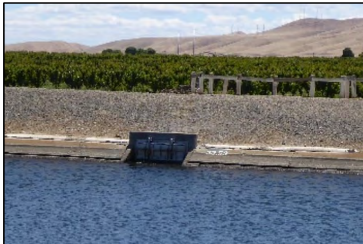
Photograph 199: View of sandbags lining the top of the concrete wall around turnout at M.P. 33.53; camera facing right bank from left bank, May 11, 2022 (A00690).
