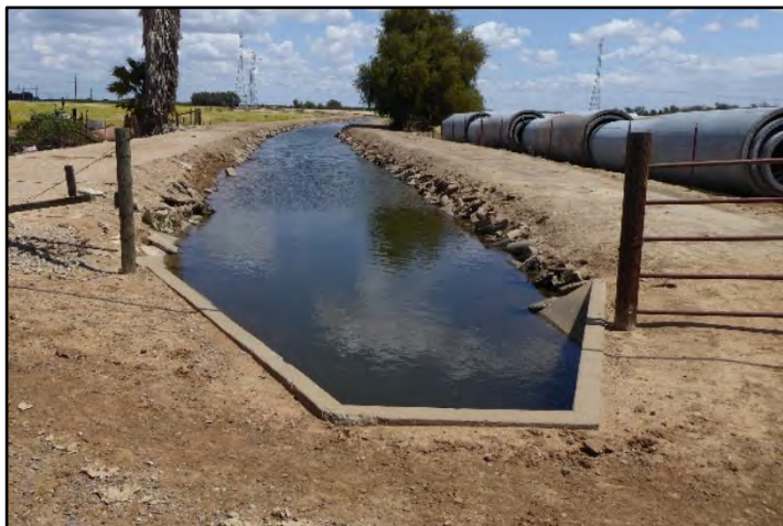
Photograph 120: View of irrigation canal at M.P. 2.92; camera facing east, May 9, 2022. (A00176)
