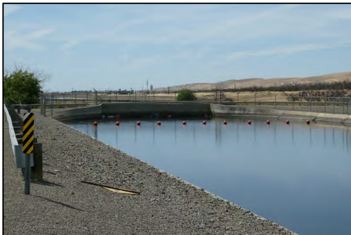
Photograph 213: Downstream view of siphon inlet headwall at M.P. 37.31; camera facing downstream from left bank, May 12, 2022 (B00234).
