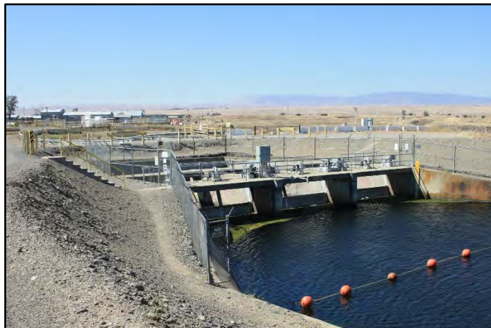
Photograph 317: Check No. 15, showing where it transitions into the Los Banos Creek Siphon inlet; camera facing downstream from left bank, June 14, 2022 (C0280).
