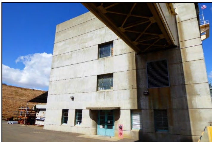
Photograph 118: Detail view of east elevation and trusses on underside of suspended walkway; camera facing southwest, May 9, 2022. (A00102)
