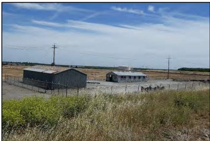
Photograph 224: Patterson O&M storage yard on the east side of the O&M road, at M.P. 40.00 containing two deteriorated and unused buildings; camera facing southeast, May 12, 2022 (B00364).
