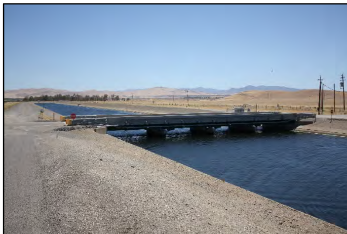
Photograph 295: Bridge at M.P. 68.03; camera facing downstream from left bank, June 13, 2022 (C0178).
