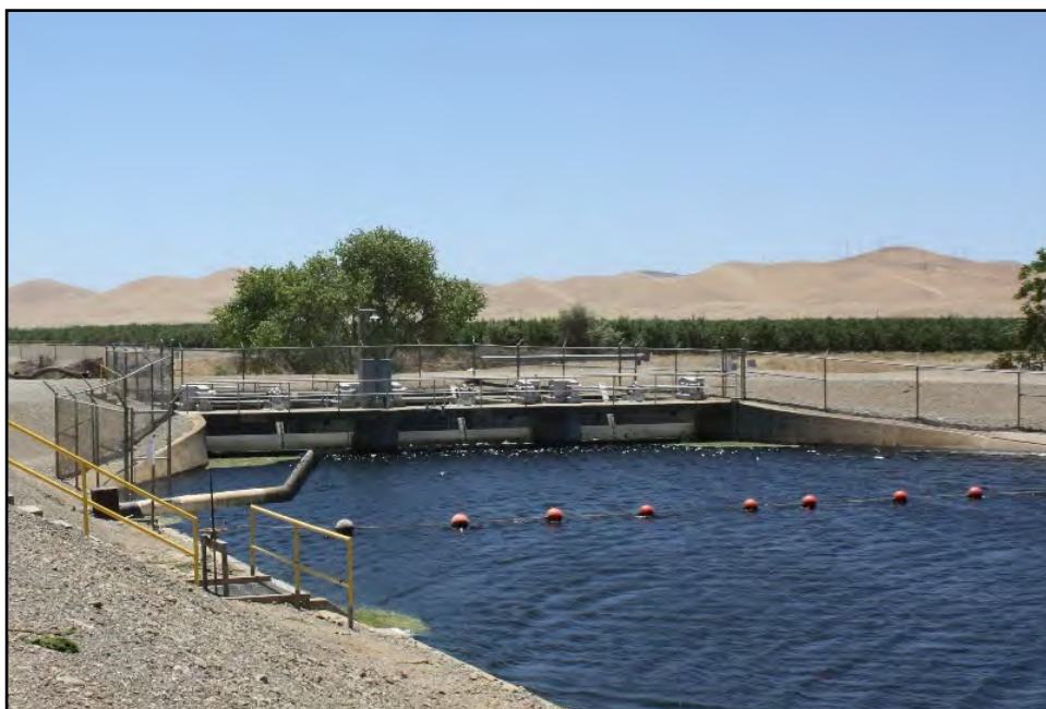
Figure 29: Check No. 11 at M.P. 58.28; camera facing downstream from left bank, June 13, 2022.
