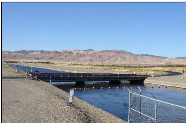
Photograph 54: View of 20-foot-wide County Highway Bridge with concrete deck and solid-type concrete pier supports at M.P. 24.48 along Koster Road; camera facing downstream from left bank, May 11, 2022 (A00490).
