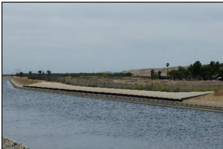
Photograph 226: Concrete overspill apron wasteway at M.P. 39.32/39.42 on the right bank is the only one of its type on the DMC; camera facing downstream from left bank; May 12, 2022 (B00338).
