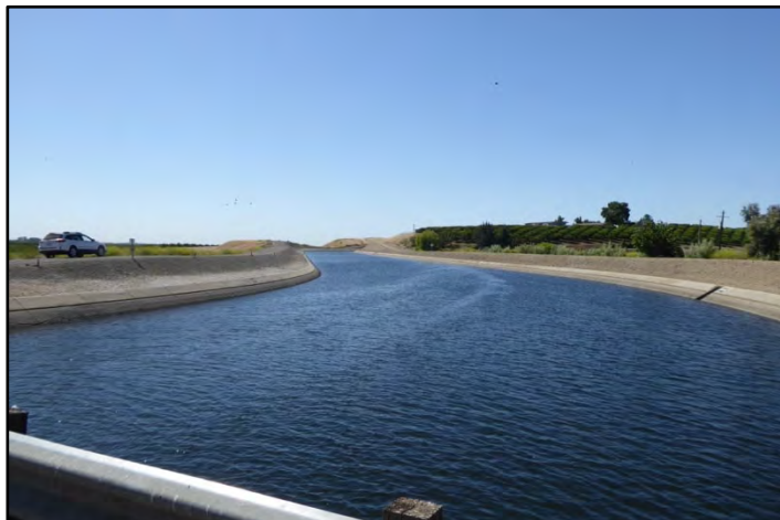
Photograph 246: Downstream view from the deck of a farm bridge at M.P. 49.55; camera facing downstream, May 13, 2022 (A00909).
