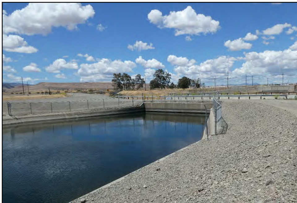
Figure 27: Four-barrel siphon outlet headwall at M.P. 16.34; camera facing upstream from left bank, May, 10, 2022.
