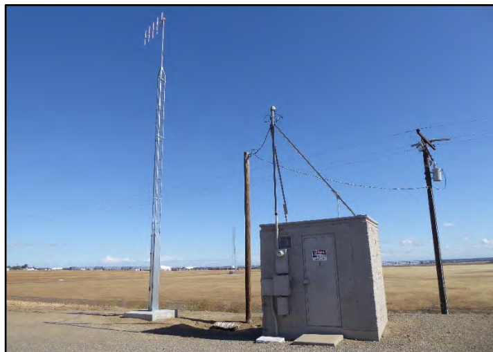
Photograph 26: Check building at Check No. 1; camera facing northwest, May 10, 2022 (A00343).
