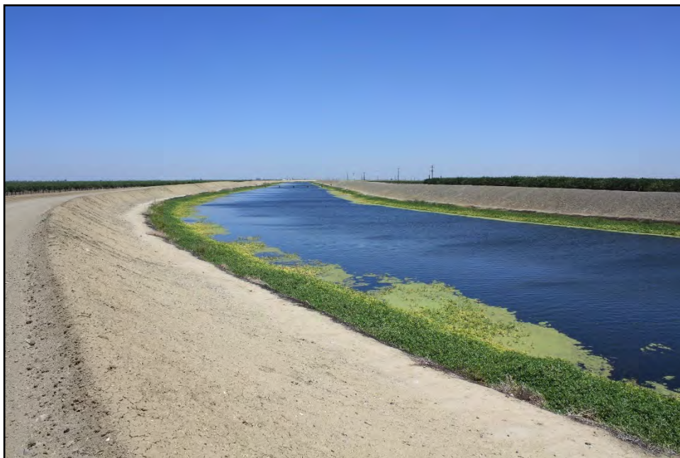
Figure 21: View of earth-lined section of canal from approximately M.P. 104.22; camera facing downstream from left bank, June 14, 2022.
