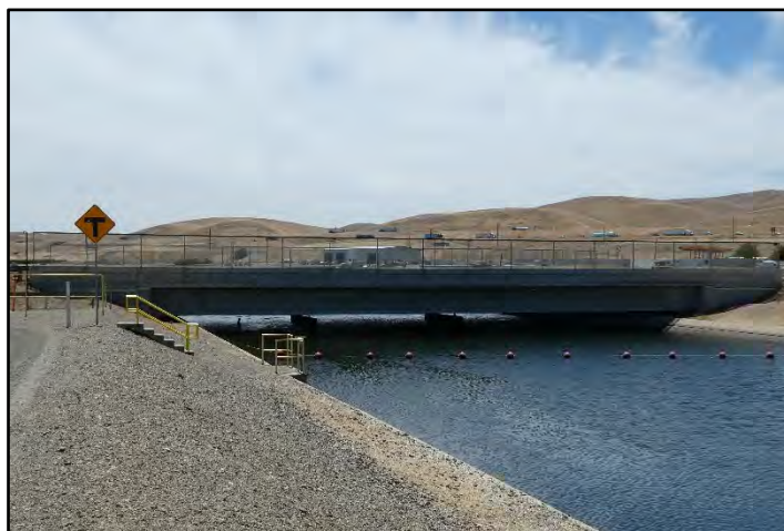
Photograph 231: Non-original replacement county highway bridge at M.P. 39.81 along Sperry Road/Hwy 130, concrete deck measuring 30 feet wide, that stretches between two large abutments with no support piers; camera facing downstream from left bank, May 12, 2022 (B00343).
