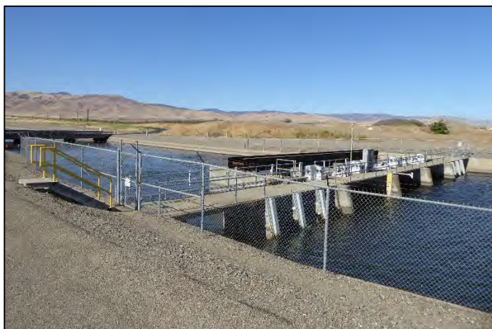
Photograph 177: Check No. 4; camera facing downstream from left bank, May 11, 2022 (A00485).
