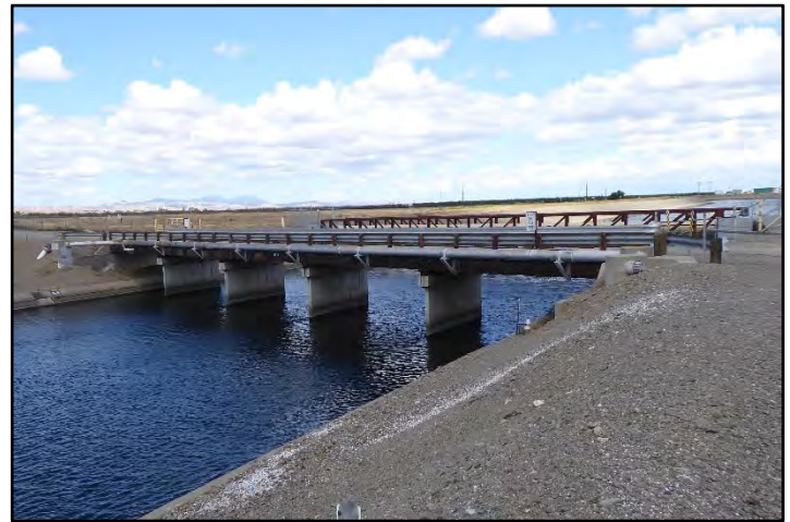
Photograph 97: Irrigation crossing attached to the downstream side of bridge at M.P. 15.10; camera facing upstream from left bank, May 10, 2022 (A00426).
