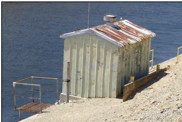
Photograph 130: View of Gage House salinity recorder house at M.P. 3.65; camera facing upstream from left bank, May 9, 2022. (A00205)
