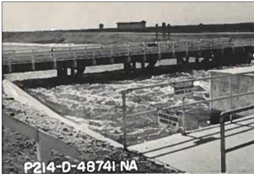
Figure 15: Bridge, Mile 90.56, scheduled for replacement. May 14, 1965. 96
