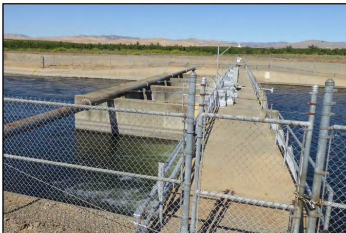
Photograph 250: Detail view of Check No. 9, showing its top deck and a pipe crossing mounted atop its support piers; camera facing right bank from left bank, May 13, 2022 (A00889).
