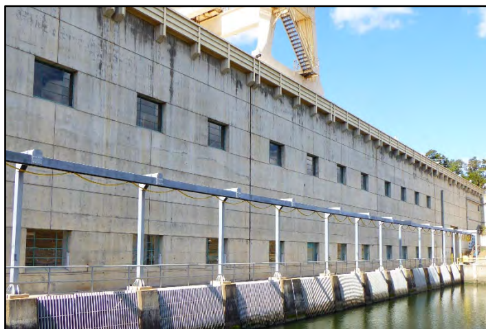
Photograph 117: View of windows on north façade of Pumping Station; camera facing west, May 9, 2022 (A00107).
