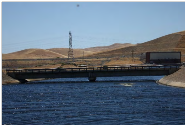
Photograph 81: View of bridge across open O'Neill forebay intake channel at M.P. 69.30; camera facing right bank from left bank, June 13, 2022 (C0190).
