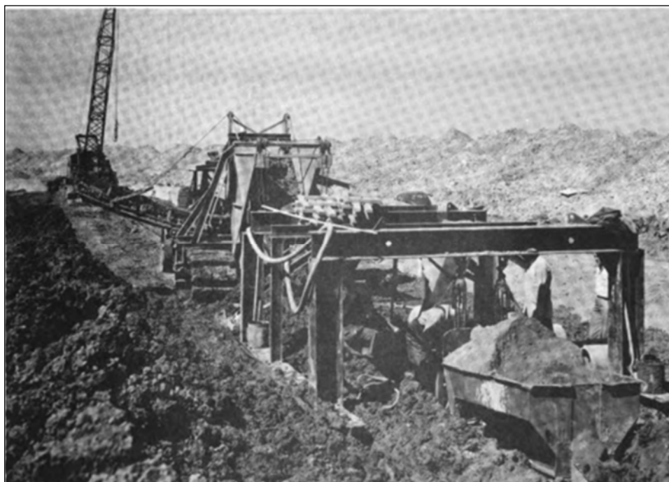
Figure 9: Converted ditcher and pipe laying machine used by United-Vinnell Co., March 1951. 73
