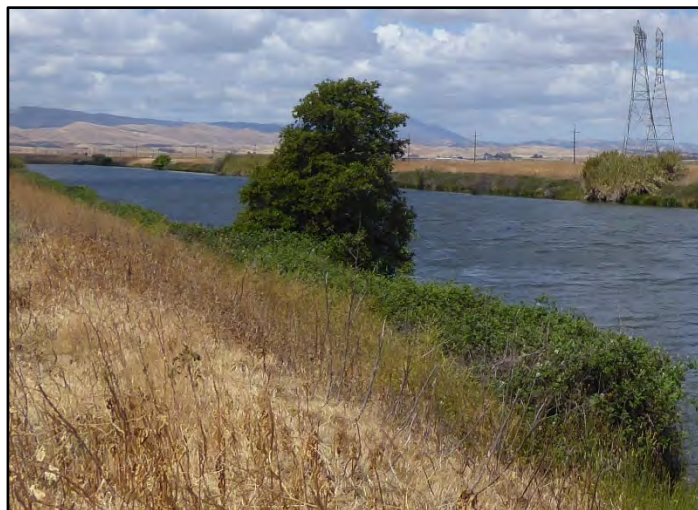
Photograph 3: View of earth lining of Intake Canal at M.P. 0.34, above Bethany-Byron Road siphon; camera facing downstream from left bank, May 9, 2022 (A00166).
