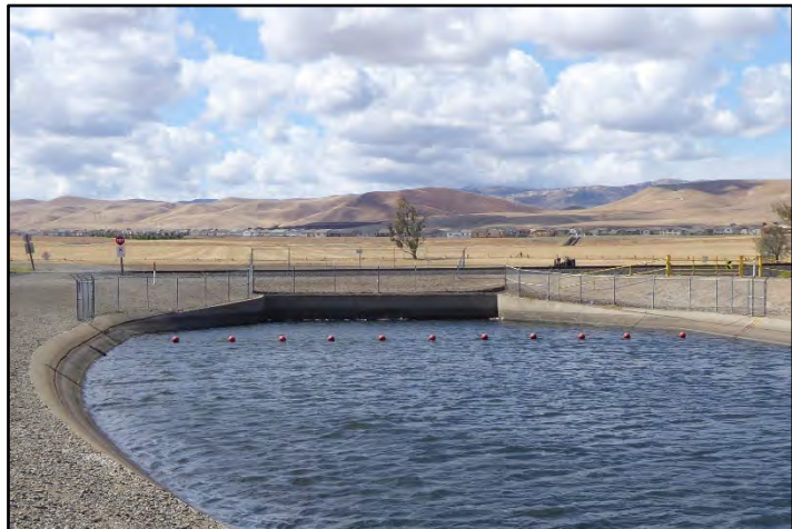
Photograph 18: 3-barrel siphon inlet at M.P. 13.69; camera facing downstream from left bank, May 10, 2022 (A0039).
