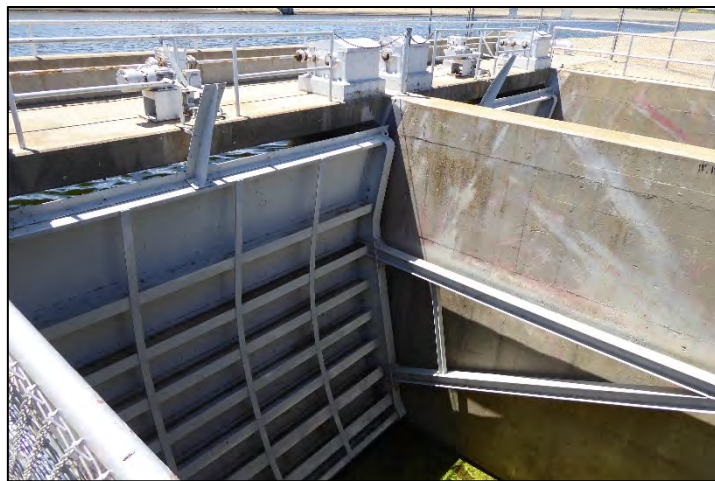
Photograph 189: Detail view of the radial gates in Westley Wasteway's inlet structure; camera facing west, May 11, 2022 (A00712).
