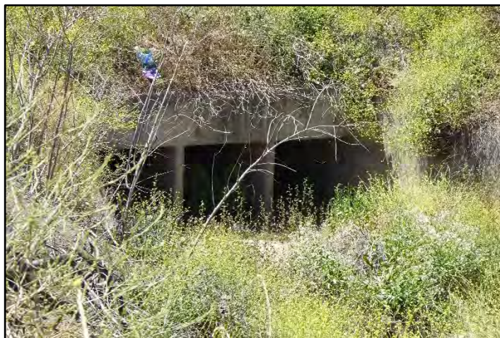
Photograph 103: Three-barrel siphon undercrossing outlet at M.P. 30.63; camera facing south, May 11, 2022 (A00633).
