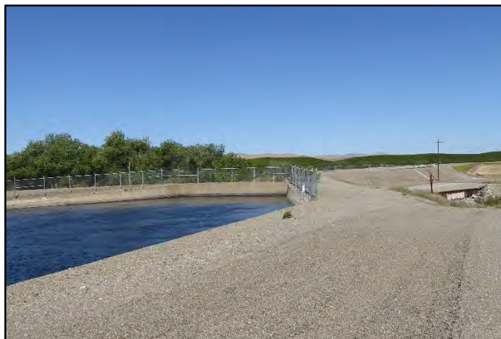
Photograph 255: Outlet headwall of Orestimba Creek siphon, at M.P. 51.27, repaired retaining wall visible in background (far right); camera facing upstream from left bank, May 13, 2022 (A00948).
