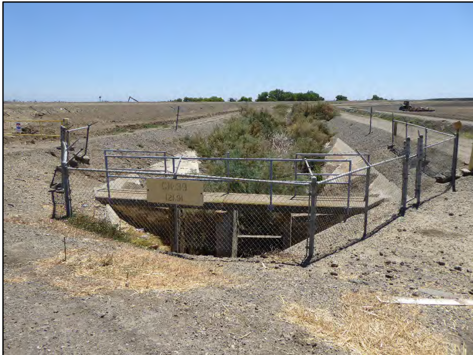
Photograph 7: Upstream view of San Luis Drain at Check Structure 39 (M.P. 121.91), with DMC (left); camera facing southeast, July 20, 2022.
