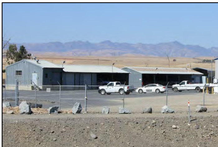
Photograph 324: Both two 5-bay garages at San Luis and Delta-Mendota Water Authority Field Office; camera facing right bank from left bank, June 14, 2022 (C0296).
