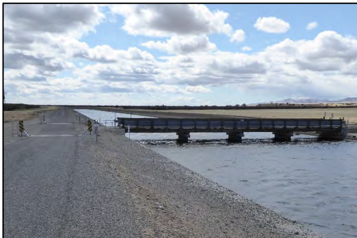
Photograph 94: View of cattle guards (left) adjacent to Farm Bridge (right) at M.P. 13.96; camera facing downstream on left bank, May 10, 2022 (A00396).
