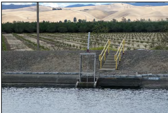
Photograph 157: View of sandbags lining the top of the canal wall at a turnout at M.P. 19.59; camera facing right bank from left bank, May 10, 2022. (B00069)
