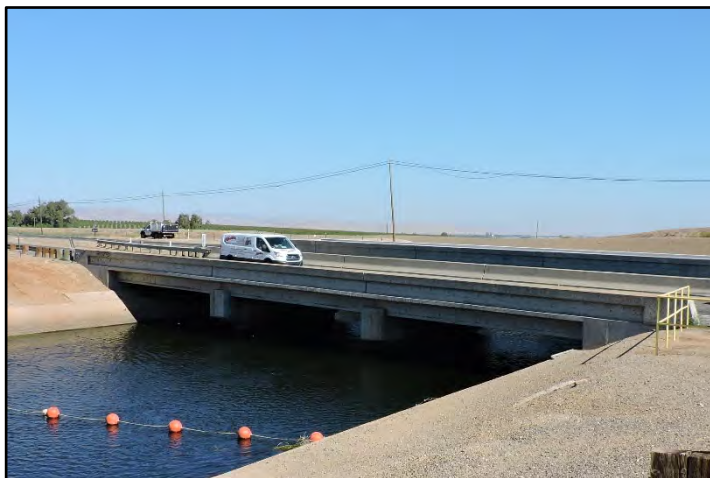
Photograph 84: View of State Highway Bridge at M.P. 75.84 along State Highway 152, with replacement concrete parapet walls; camera facing upstream from left bank, June 13, 2022 (D2237).
