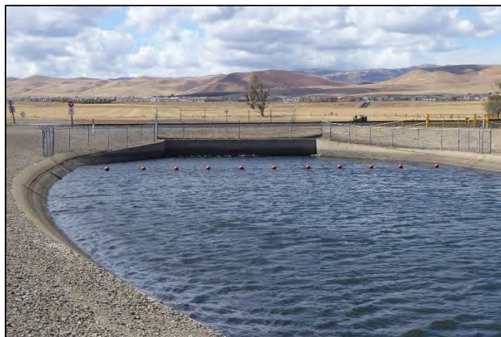
Photograph 142: Western Pacific Railroad Siphon inlet headwall at M.P. 13.67; camera facing downstream from left bank, May 10, 2022 (A00392).
