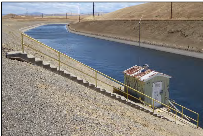
Photograph 131: View of Gage House salinity recorder house and access stairs at M.P. 3.65 and concrete canal lining; camera facing downstream from left bank, May 9, 2022. (A00206)
