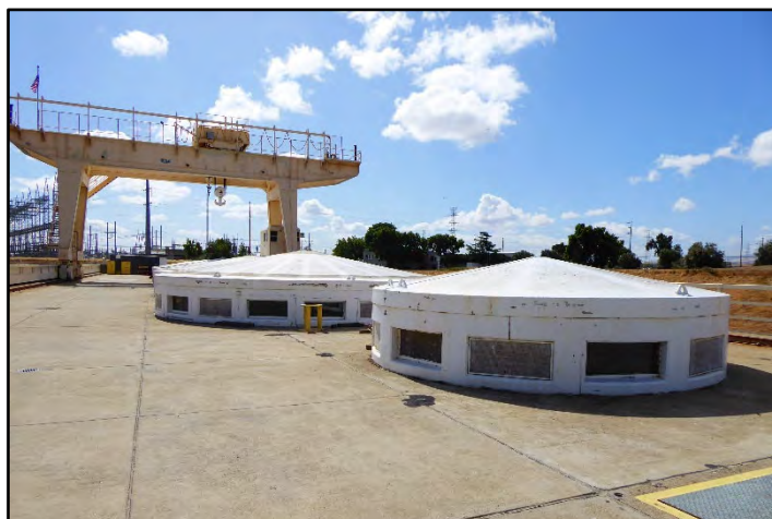
Photograph 115: Detail view of removable hatches on roof of Pumping Station with gantry in background (left); camera facing east, May 9, 2022. (A00091)
