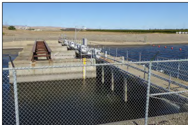
Photograph 178: Check No. 4; camera facing right bank from left bank, May 11, 2022 (A00489).
