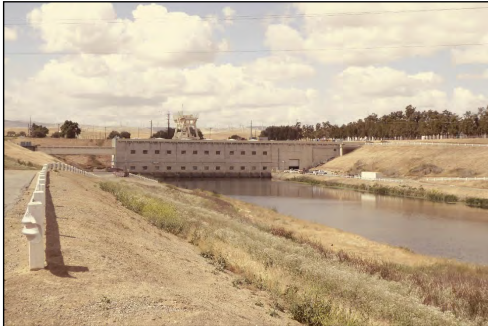
Figure 24: Tracy Pumping Plant; camera facing southwest, May 9, 2022.
