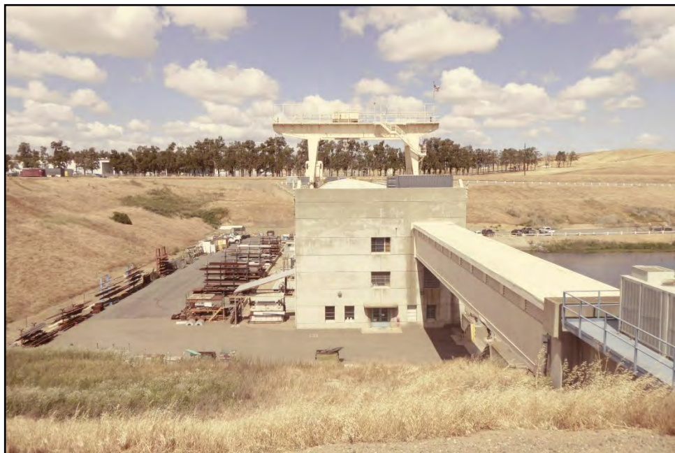
Figure 25: Tracy Pumping Plant; camera facing east, May 9, 2022.
