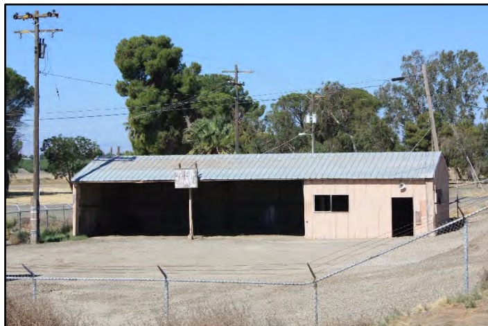
Photograph 373: Front (east) side of three-bay garage; camera facing west, June 15, 2022 (C0542).
