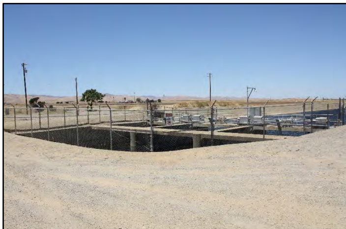
Photograph 276: Transition between Check No. 11 and Garzas Creek Siphon; camera facing right upstream from left bank, June 13, 2022 (C0087).
