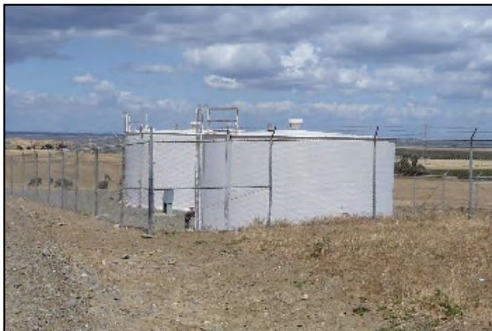
Photograph 124: View of 64-gallon water storage tanks at M.P. 3.49; camera facing north, May 9, 2022. (A00192)
