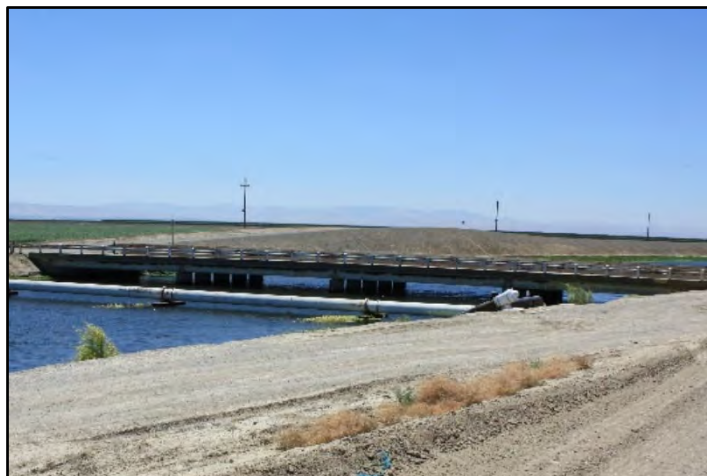
Photograph 57: View of 26-foot-wide County Highway Bridge with concrete deck supported by three (3) concrete bents at M.P. 105.03 in earth-lined section of DMC along Jerrold Avenue; camera facing upstream from left bank, June 14, 2022 (C0454).
