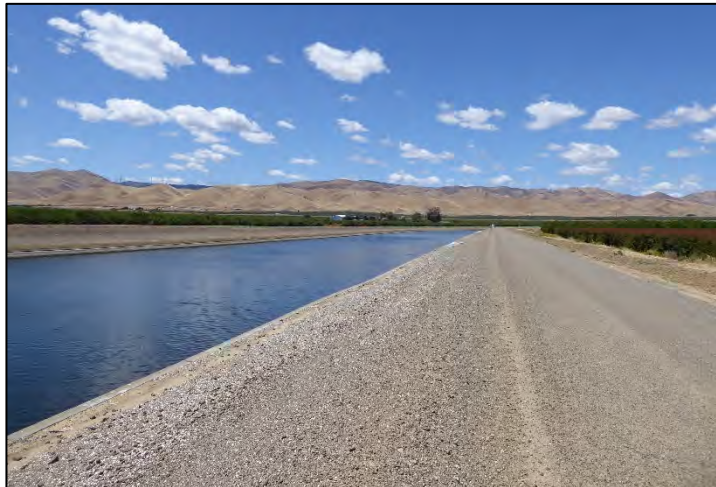
Photograph 182: Upstream view from approximately M.P. 30.33; camera facing upstream from left bank, May 11, 2022 (A00615).
