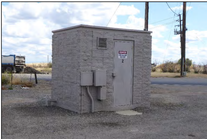
Photograph 150: Check building at Check No. 2; camera facing northeast, May 10, 2022 (A00451).
