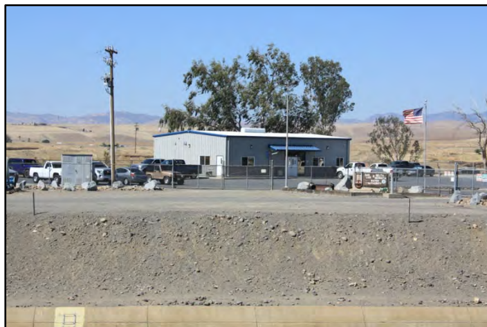
Photograph 323: Office building at San Luis and Delta-Mendota Water Authority Field Office; camera facing right bank from left bank, June 14, 2022 (C0295).
