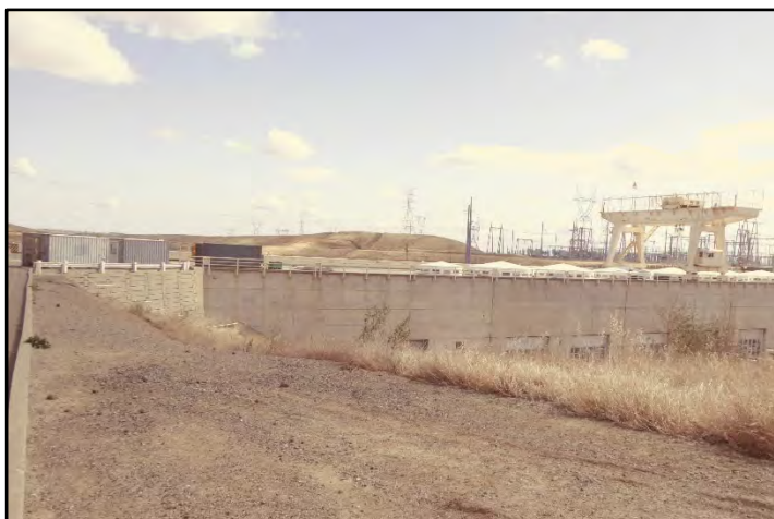
Photograph 114: Roof access to Pumping Station from Road; camera facing northeast, May 9, 2022. (A00082)
