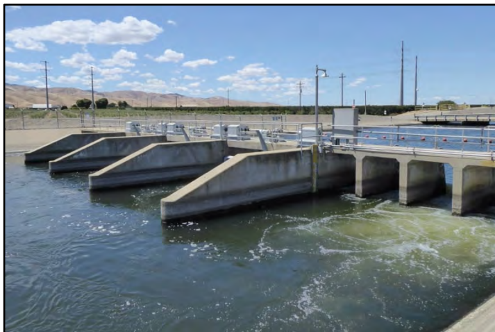
Photograph 209: Upstream view of Check No. 6; camera facing upstream from left bank, May 11, 2022 (A00723).
