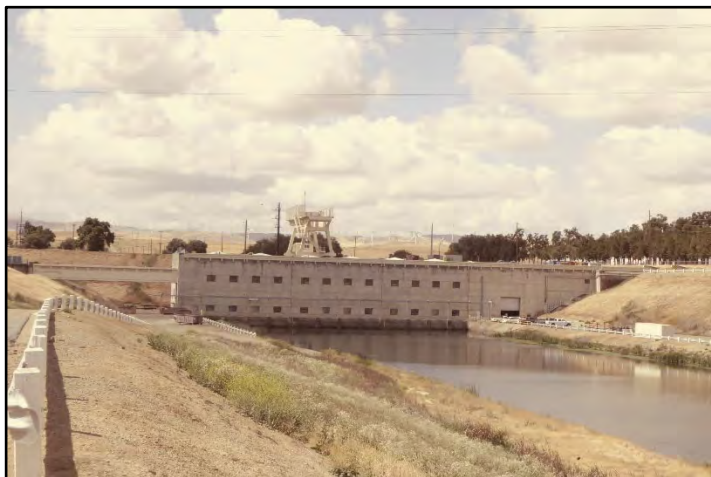
Photograph 110: North elevation of Pumping Station; camera facing south, May 9, 2022. (A00144)
