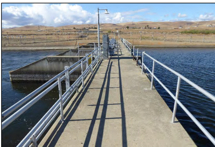
Photograph 138: Top deck of Check No. 1; camera facing right bank, May 10, 2022 (A00342).
