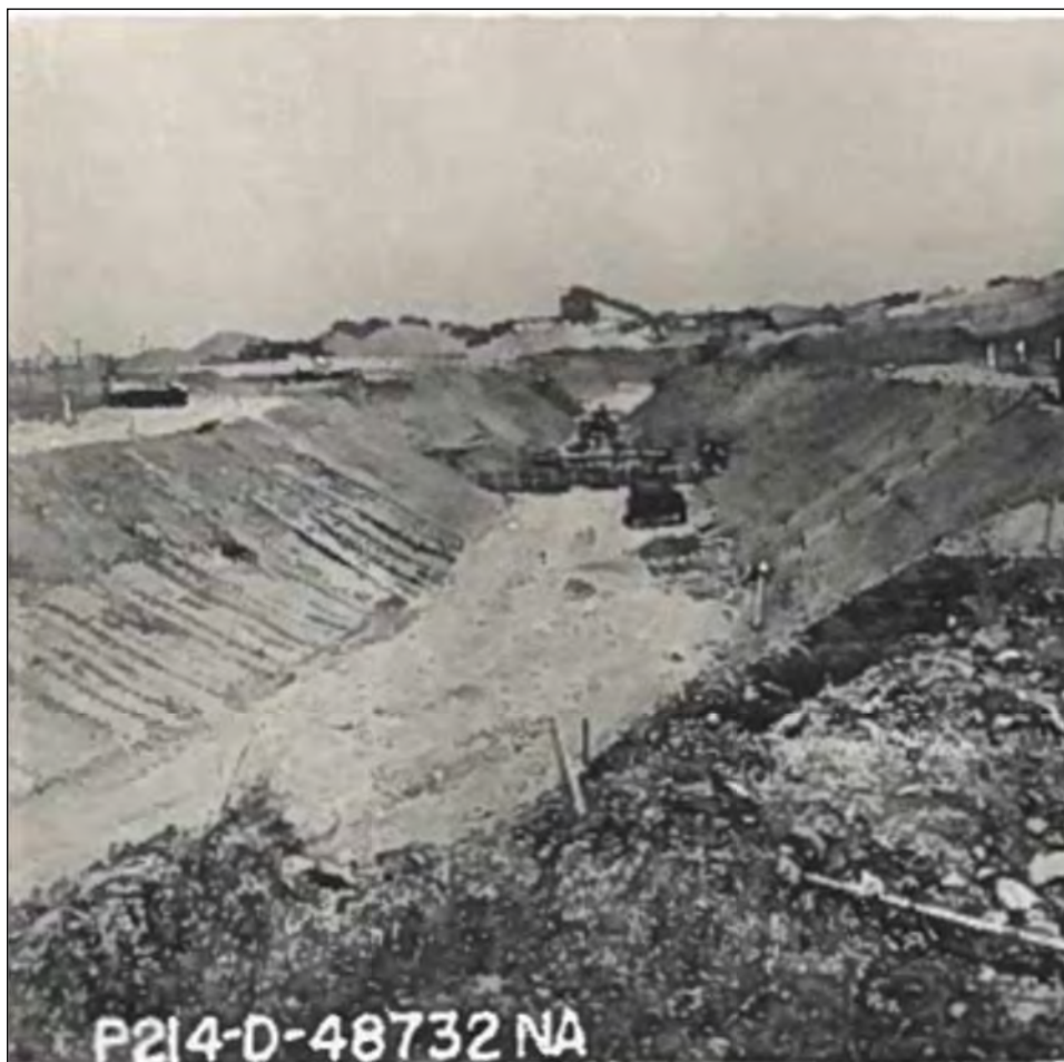
Figure 16: Baffled apron drop under construction, May 12, 1965. 97
