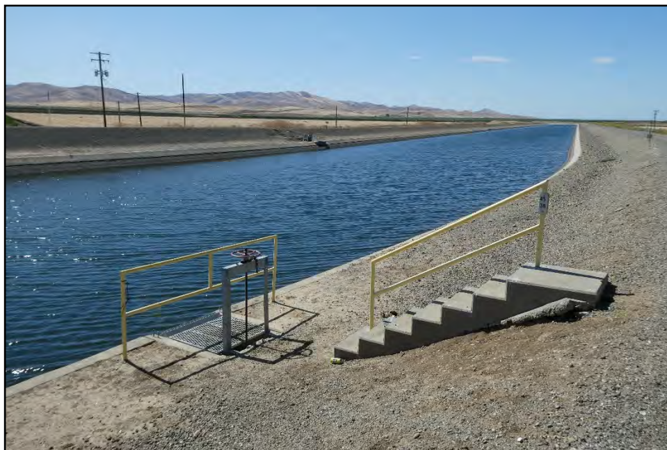
Figure 32: Turnout at M.P. 45.35; camera facing downstream from left bank, May 12, 2022.
