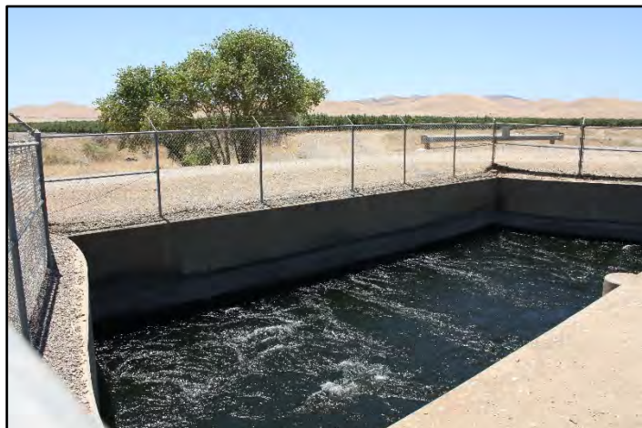
Photograph 278: Garzas Creek Siphon's inlet headwall; camera facing downstream from left bank, June 13, 2022 (C0085).
