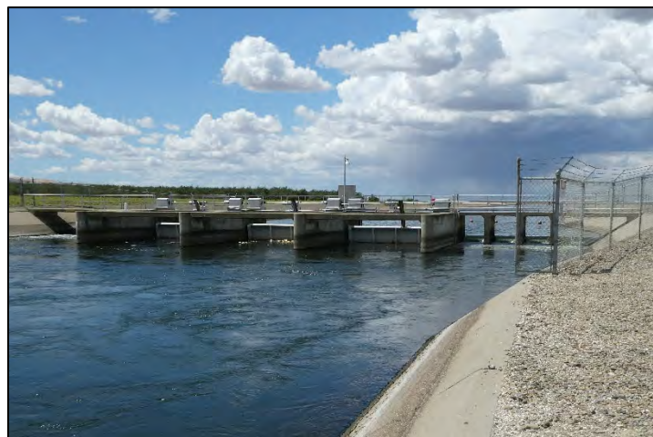
Photograph 165: Check No. 3; camera facing upstream from left bank, May 10, 2022 (B00091).
