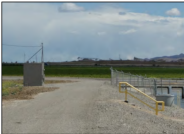
Photograph 28: View of check building (left) in relation to associated check structure (Check No. 3, right) with a stilling well in the foreground (bottom right), May 10, 2022 (B00084).
