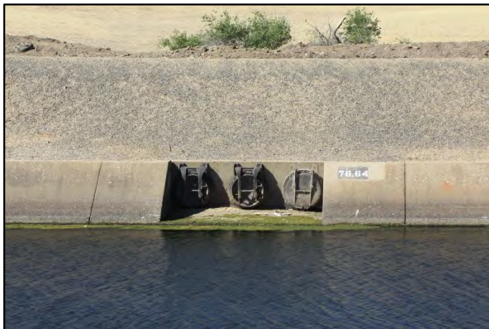
Photograph 47: Triple flap-gate inlet drain along the right bank at M.P. 76.64; camera facing from left bank, June 14, 2022 (C0253).
