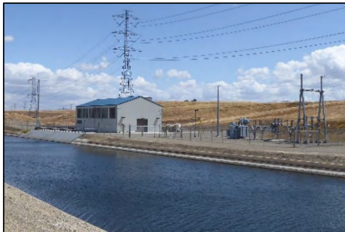
Photograph 129: View of electrical substation adjacent to pumphouse at M.P. 7.50; camera facing downstream from left bank, May 9, 2022. (A00250)
