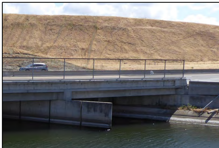
Photograph 85: Detail view of State Highway Bridge at M.P. 7.67 along Interstate 205, with replacement concrete parapet walls with additional metal fencing on top; camera facing downstream from left bank, May 9, 2022 (A00261).
