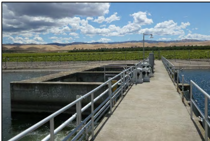
Photograph 166: Deck of Check No. 3; camera facing right bank from left bank, May 10, 2022 (B00090).
