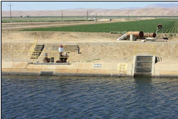
Photograph 37: An original turnout altered by the addition of an automatic, electronic gate-operating system (left) and a modern turnout (right) along the right bank at M.P. 90.53; camera facing from left bank, June 14, 2022 (C0365).
