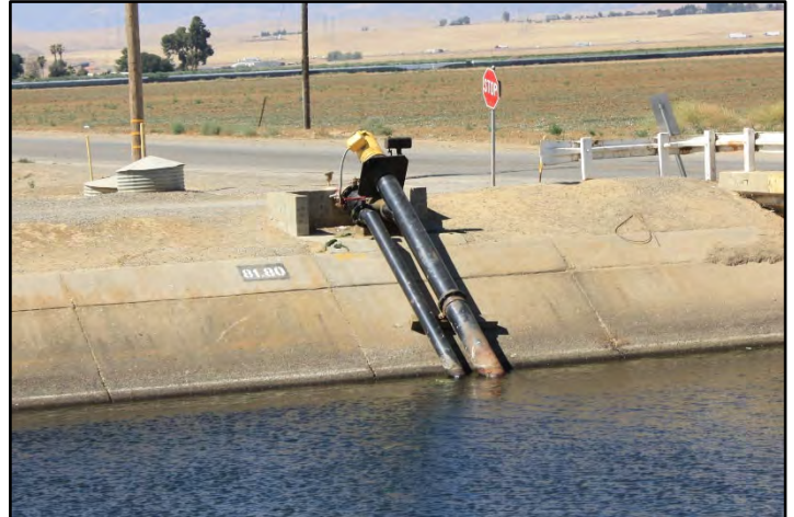
Photograph 40: Modern overlining turnout along right bank at M.P. 81.80; camera facing southwest, June 14, 2022 (C0310).
