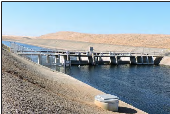
Photograph 305: Check No. 14; camera facing downstream from left bank, June 14, 2022 (D2216).
