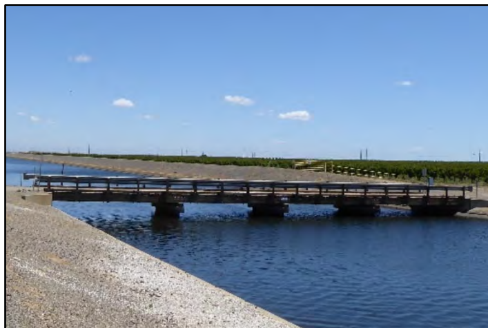
Photograph 93: View of replacement Timber Operating Bridge, constructed in 1998, at M.P. 33.29, with a 16-foot-wide timber deck supported by three concrete piers, with steel guard-rails; camera facing downstream from left bank, May 11, 2022 (A00684).
