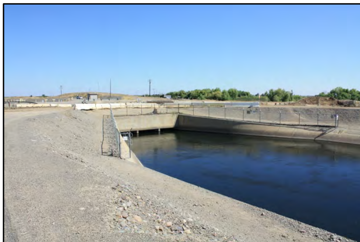
Photograph 319: Los Banos Creek Siphon outlet at M.P. 79.69; camera facing upstream from right bank, June 14, 2022 (C0293).
