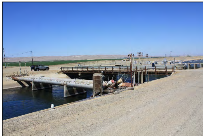
Photograph 336: View from approximately M.P. 90.57, showing a pipe crossing, operating bridge, and Check No. 17 in the background; camera facing upstream from left bank, June 14, 2022 (C0371).
