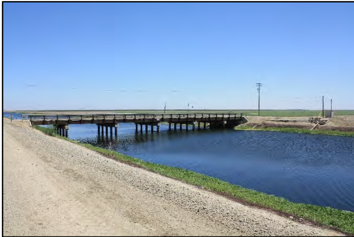
Photograph 72: View of 30-foot-wide Farm Bridge at M.P. 100.85, with original timber deck supported by five replacement concrete bents, with modern steel guard-rails; camera facing downstream from left bank, June 14, 2022 (C0436).
