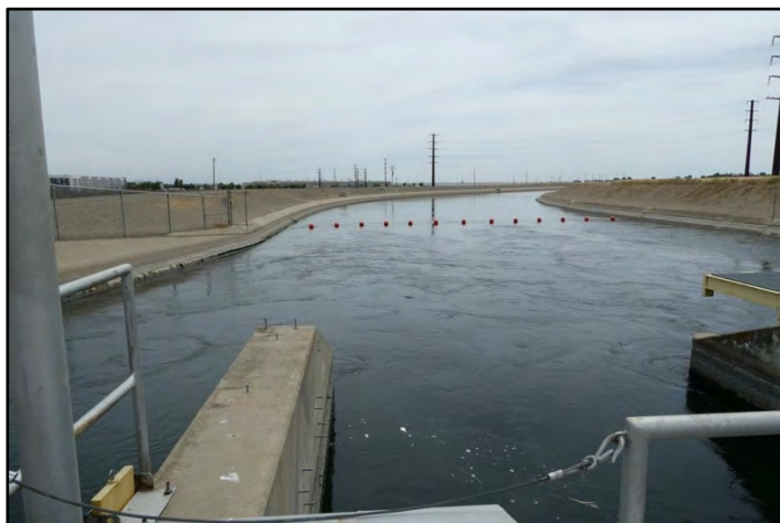
Photograph 218: Downstream view from the deck of Check No. 7; camera facing downstream, May 12, 2022 (B00318).
