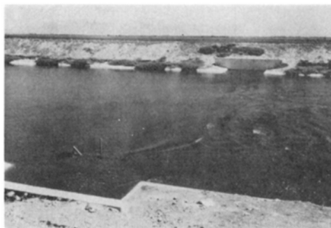
Fig. 9. Effect of Subsidence on Pipe Crossing at Near Capacity Flow
