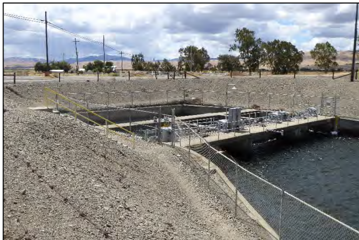
Photograph 149: View of Check No. 2, showing its transition into the Tracy Boulevard Siphon; camera facing downstream from left bank; May 10, 2022 (A00448).
