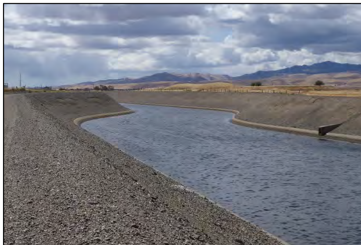
Photograph 136: Downstream view of deep excavation cuts at approximately M.P. 15.50; camera facing downstream from left bank, May 10, 2022 (A00431).
