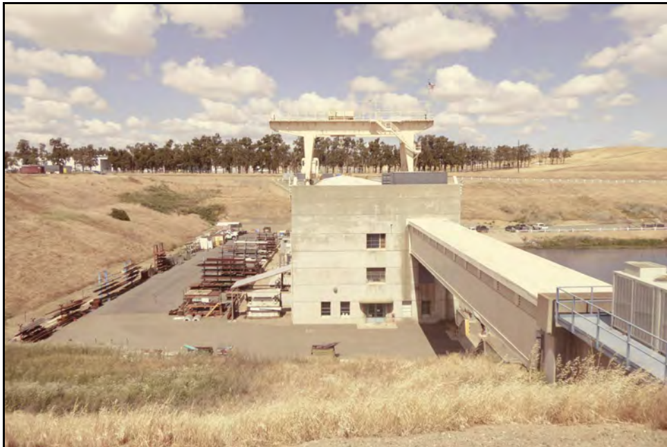
Figure 34: Tracy Pumping Plant; camera facing east, May 9, 2022.
