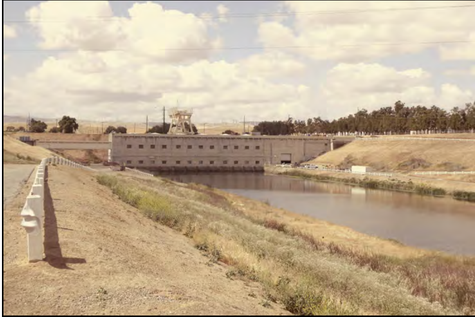
Figure 33: Tracy Pumping Plant; camera facing southwest, May 9, 2022.
