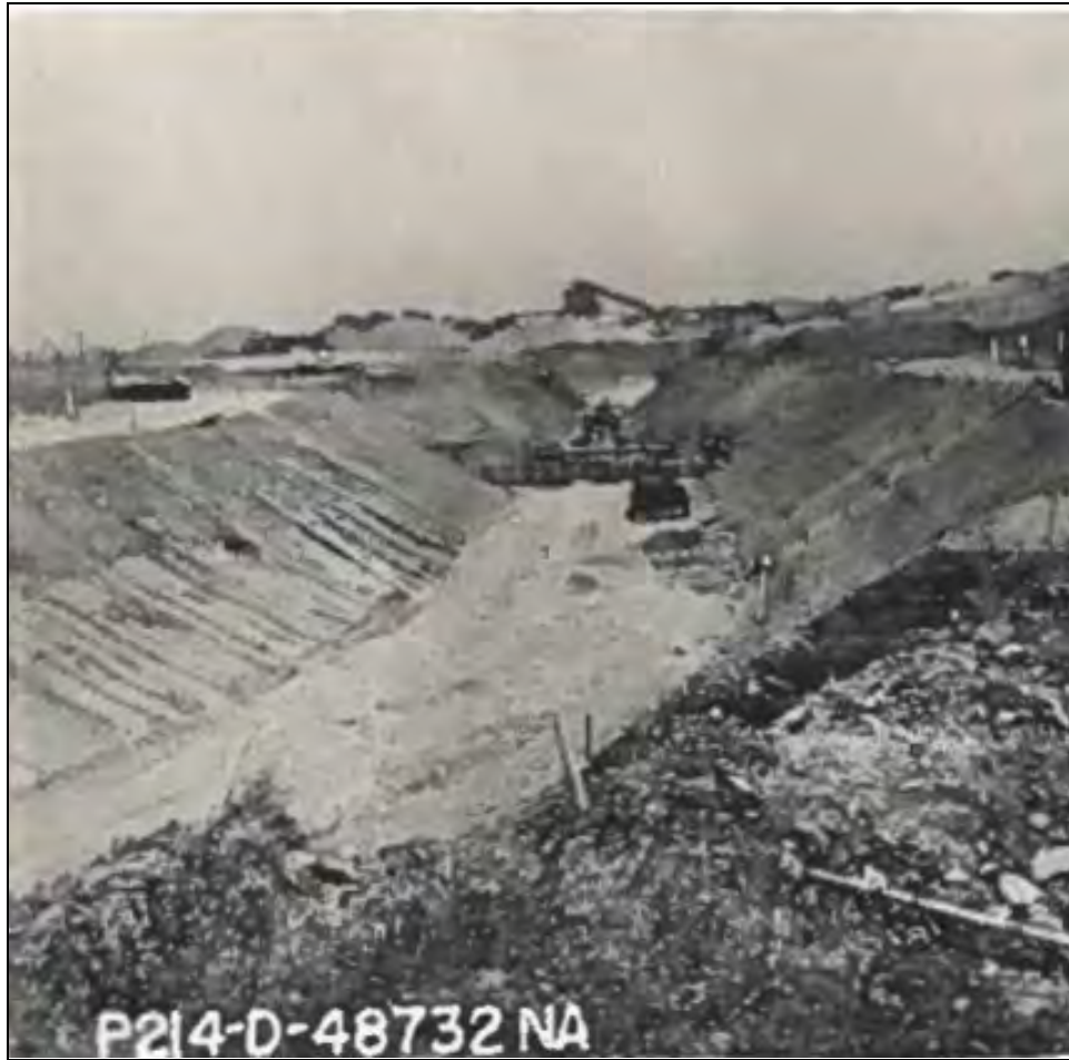
Figure 18: Baffled apron drop under construction, May 12, 1965. 71
