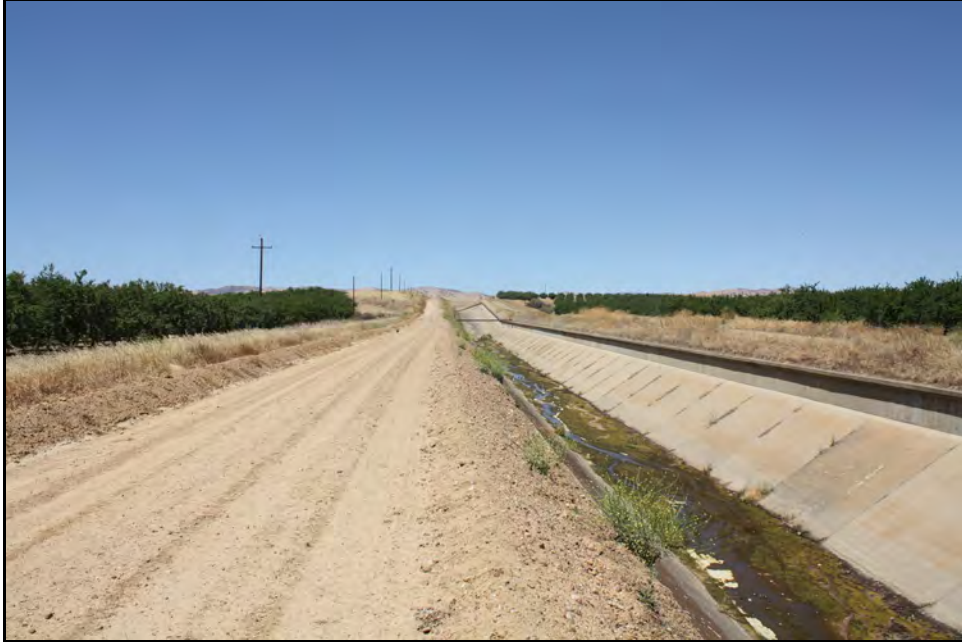
Figure 40: View of Newman Wasteway; camera facing upstream from right bank, June 13, 2022.
