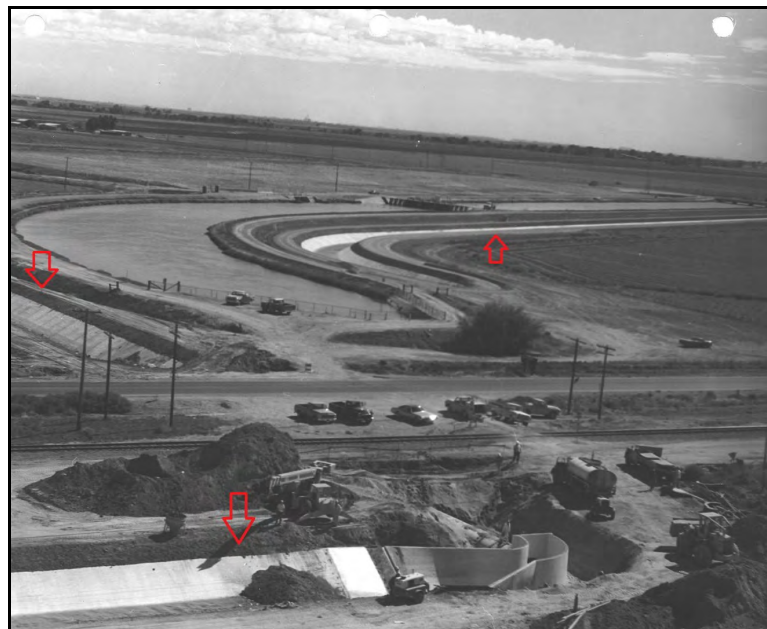
Figure 25: Archival photograph of Ball, Ball & Brosamer constructing outlet transition at UPRR / SR 33 siphon undercrossing, September 20, 1973. San Luis Drain indicated by arrows. Note Delta-Mendota Canal next to the SLD in the middle ground. 90
