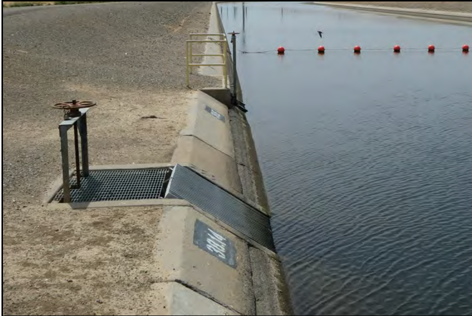
Figure 42: Two turnouts at M.P. 38.14; camera facing downstream from left bank, May 12, 2022.
