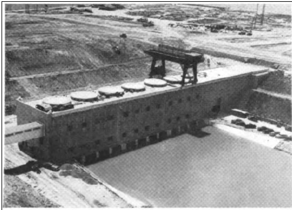
Figure 8: Tracy Pumping Plant, January 1951. 43
