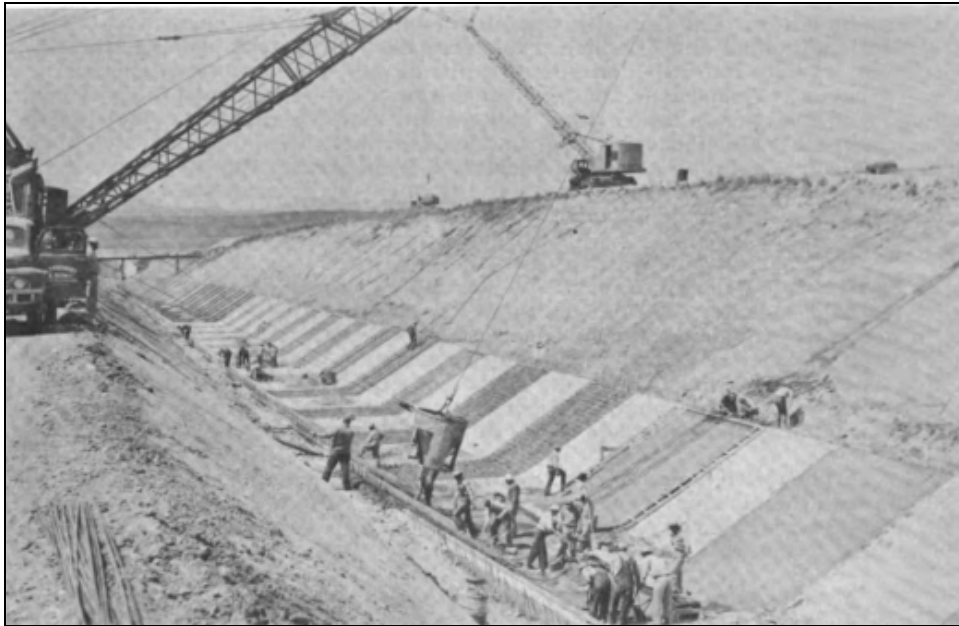
Figure 12: Placing alternate panels of reinforced concrete in Newman wasteway, April 1951. 49
