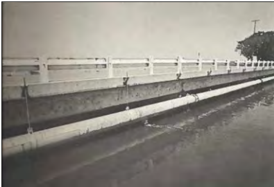
Figure 19: Discharge of barnyard manure into the canal, May 16, 1970. 73
