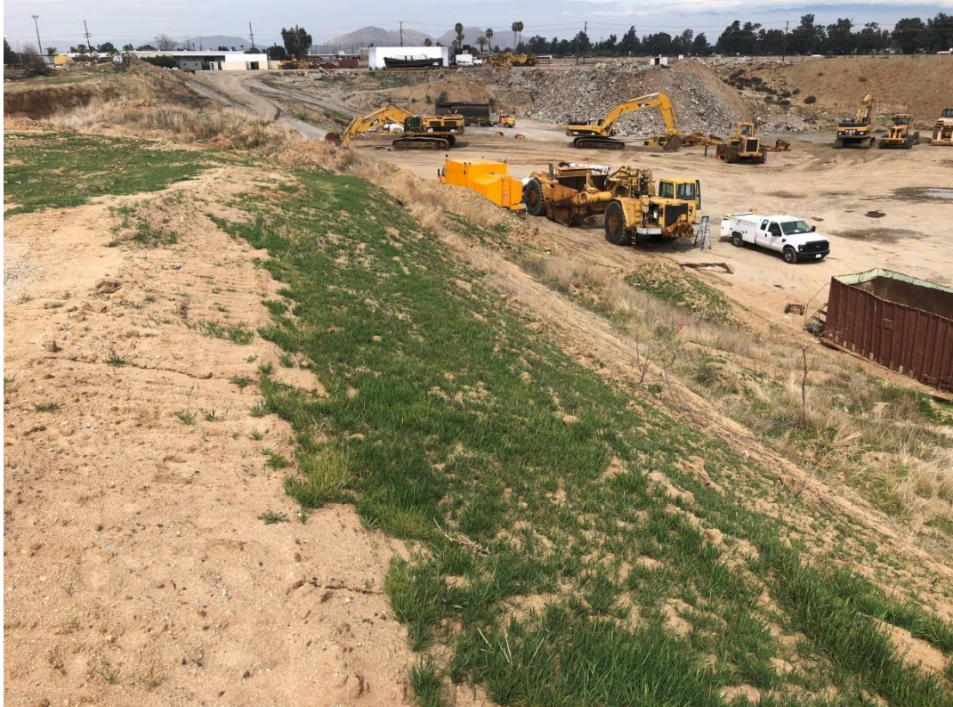
Figure 4. Overview of project site and heavy equipment, facing north
