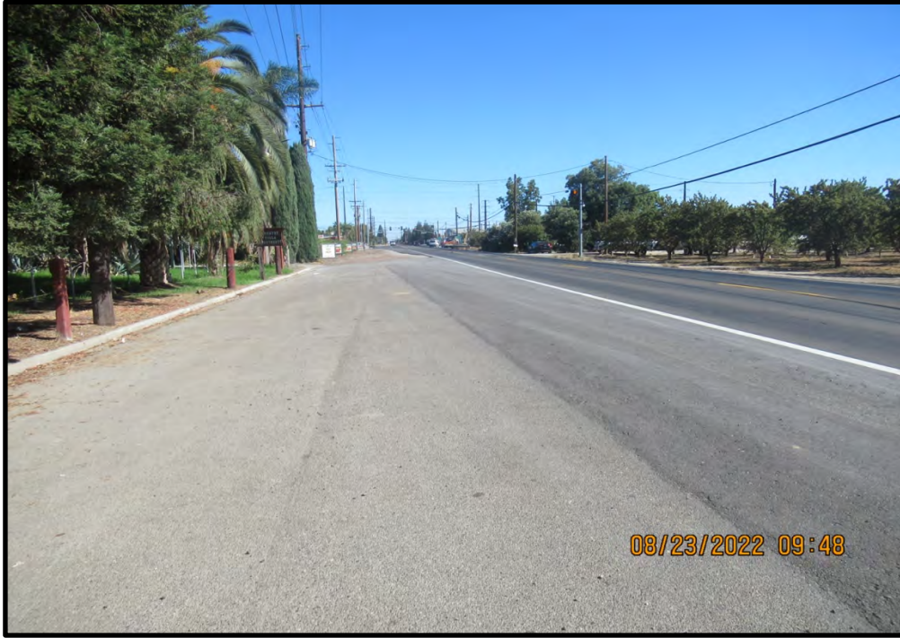
South end of the alignment, looking north along Geer Road; 08/23/22.
