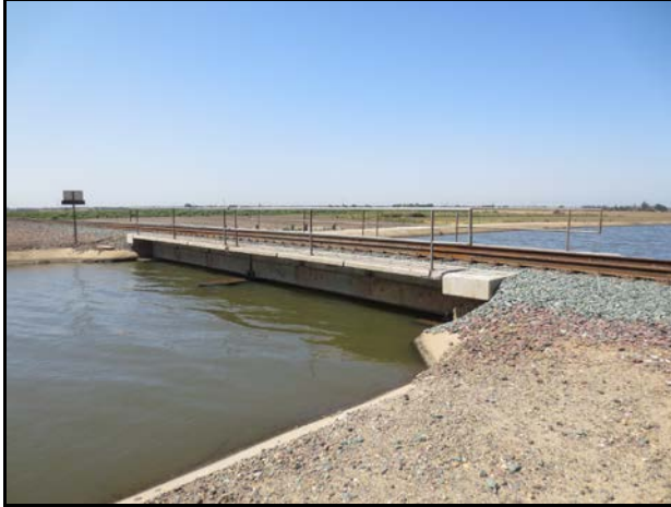
Photo 6: Feature B (bridge), facing southwest.
