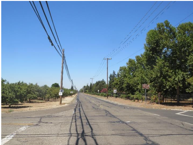
Photo 3156. APE overview, along E. Whitmore Ave. at Euclid Rd. – view to west
