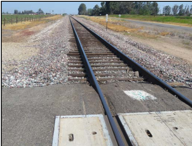
Photo 2: ATSF Segment 1 with Feature A in background, facing NW.
