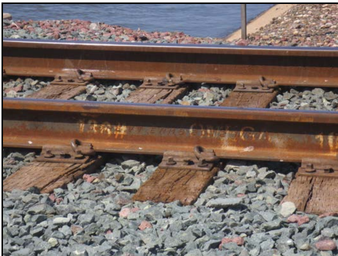
Photo 4: Detail of modern baseplates, spikes, and 1998 date-stamped rail.
