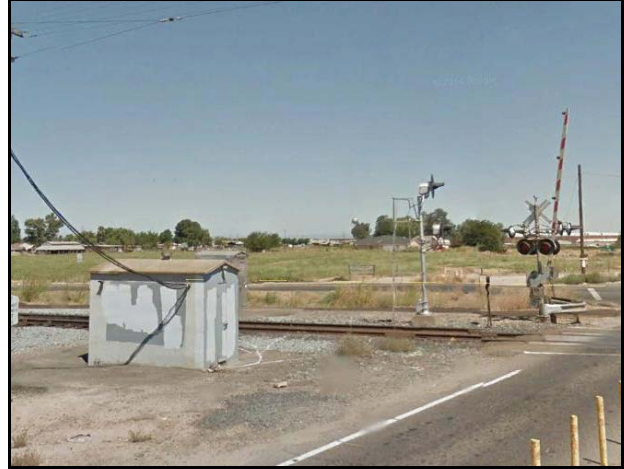
Photo 7: Feature C (crossing gate and shed), facing northeast.
