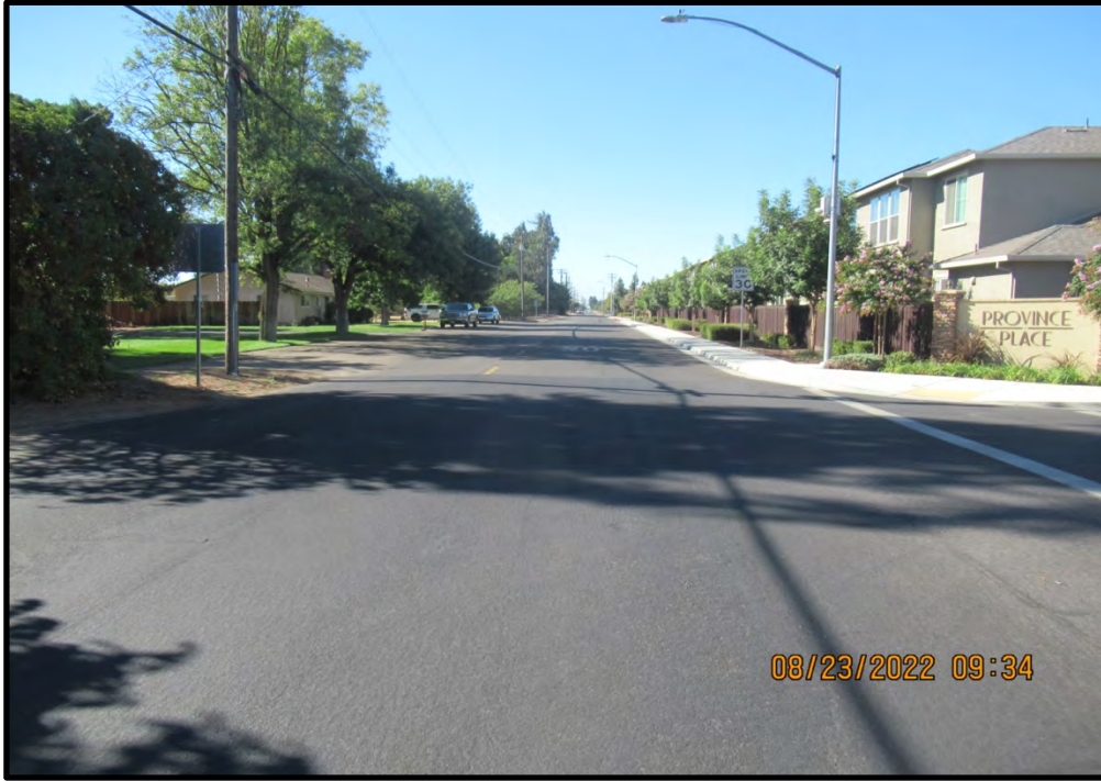
North end of the pipeline alignment, looking south down Euclid Avenue; 08/23/22.
