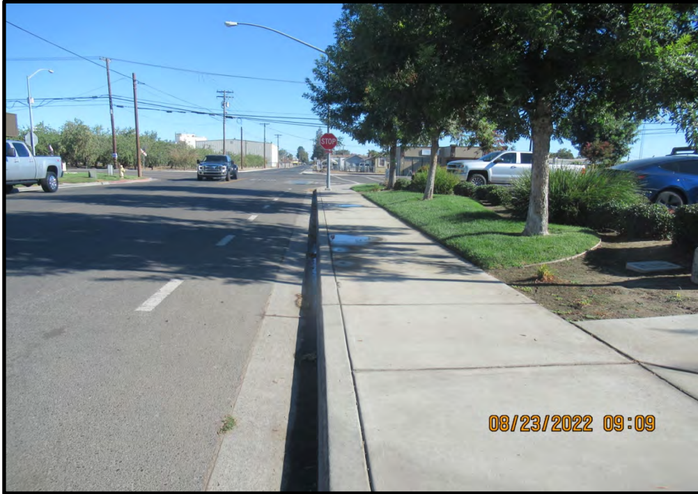
West end of the alignment, looking north along Tully Road; 08/23/22.
