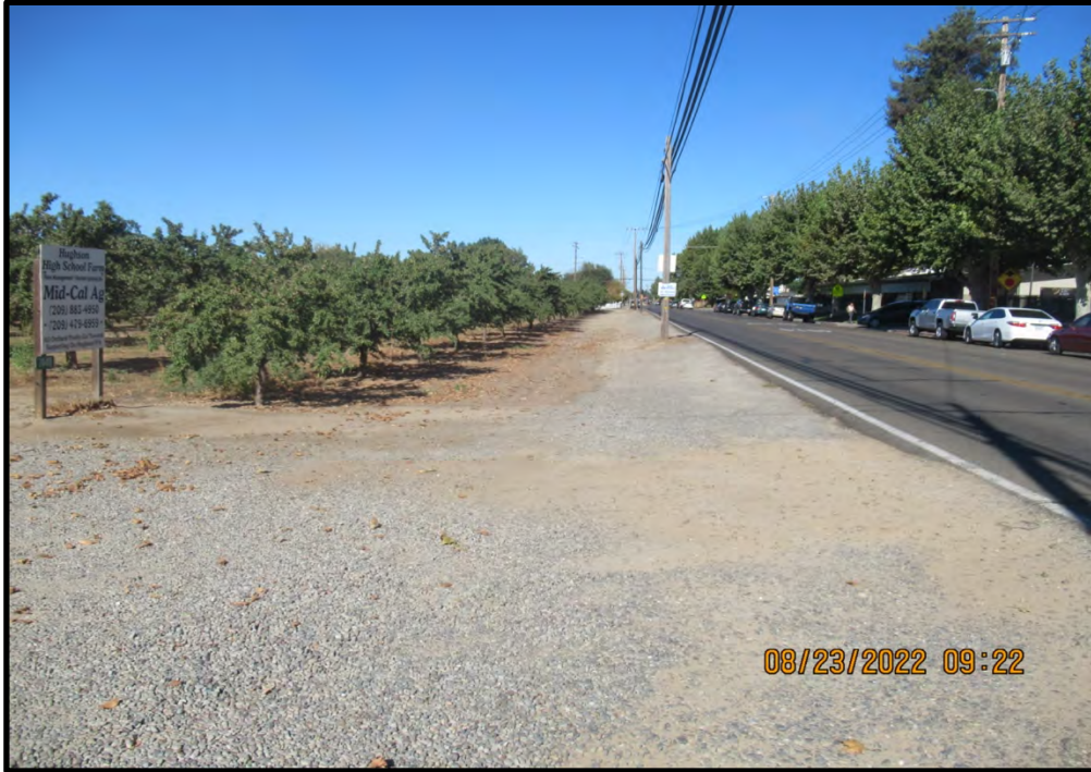
Road shoulder in the approximate central part of the alignment, looking west along E. Whitmore Avenue; 08/23/22.
