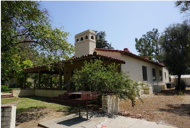
South and West Facades of South Wing, facing northeast.
