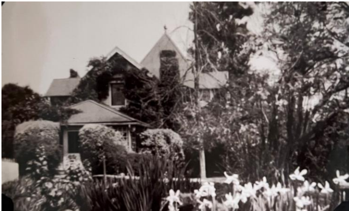
Santa Fe Station, first summer residence of Morrison family in Duarte (demolished), circa 1914. Source: Westminster Gardens.
