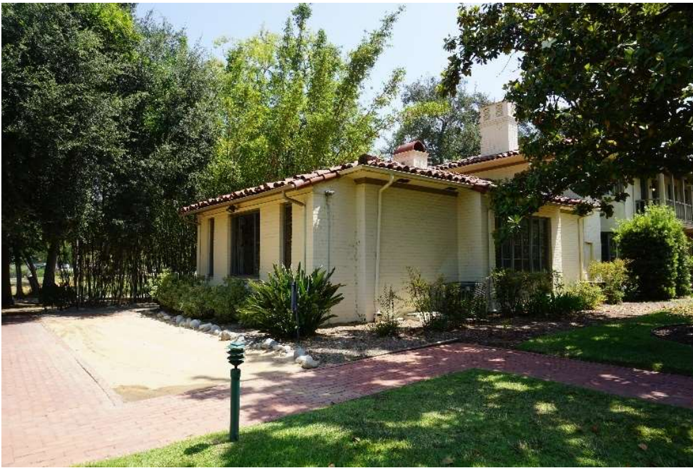
South and West Façade of North Wing, Morrison House, facing northeast.
