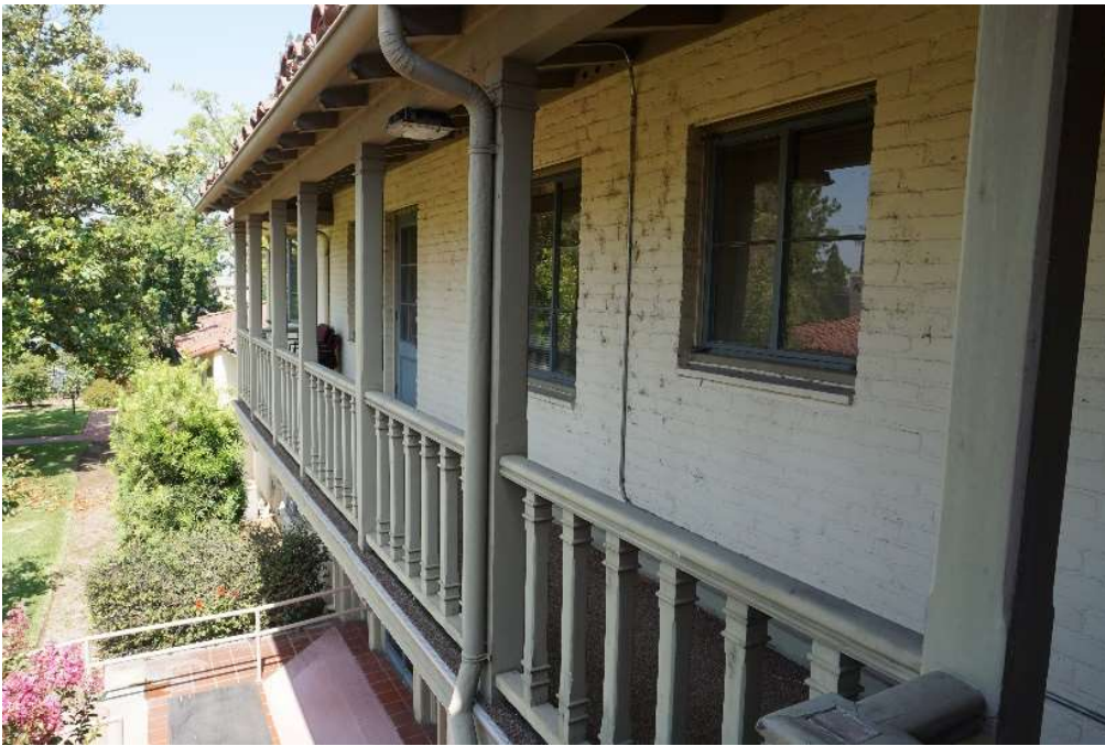
Balcony on South Façade of North Wing, Morrison House, facing west.
