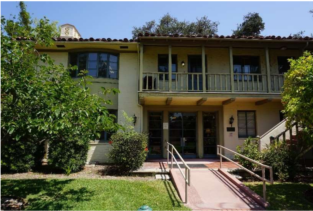
Primary Entrance, South Façade of North Wing, Morrison House, facing north.
