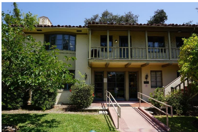
Primary Entrance, South Façade of North Wing, facing north.
