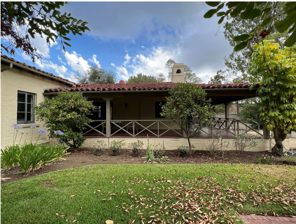
North Façade of South Wing, Morrison House, facing south.
