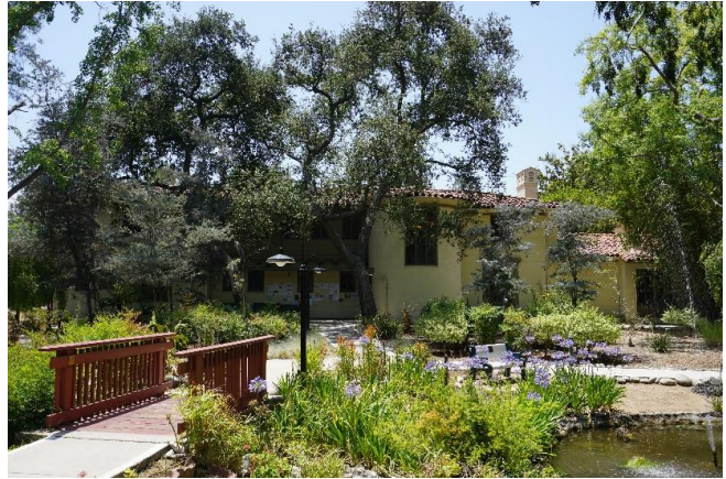
North Façade of North Wing, facing south.
