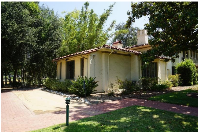
South and West Façade of North Wing facing northeast.
