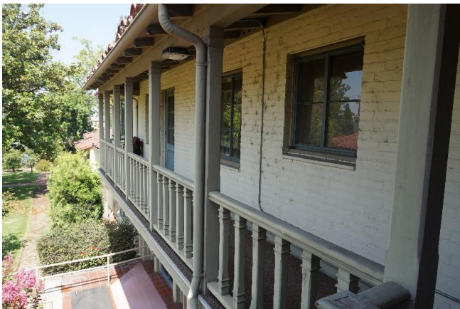
Balcony on South Façade of North Wing, facing west.
