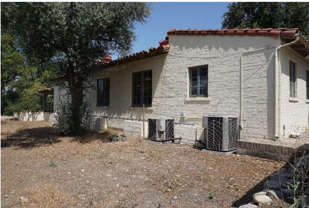
South Façade of South Wing, Morrison House, facing northwest.
