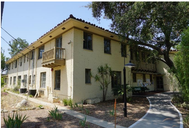
North Façade of North Wing, facing southwest.
