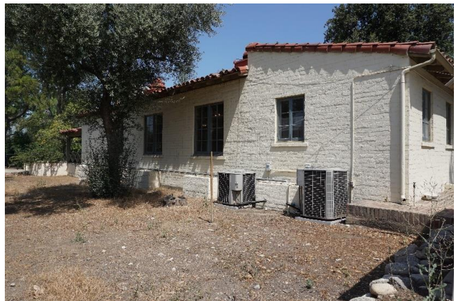
South Façade of South Wing, facing northwest.
