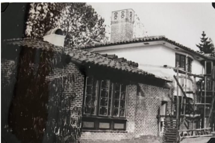
Completed North Wing (La Casa Soñada) of Morrison House, 1940. Source: Westminster Gardens.
