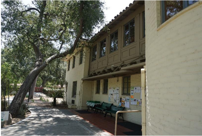
North Façade of North Wing, facing southeast.
