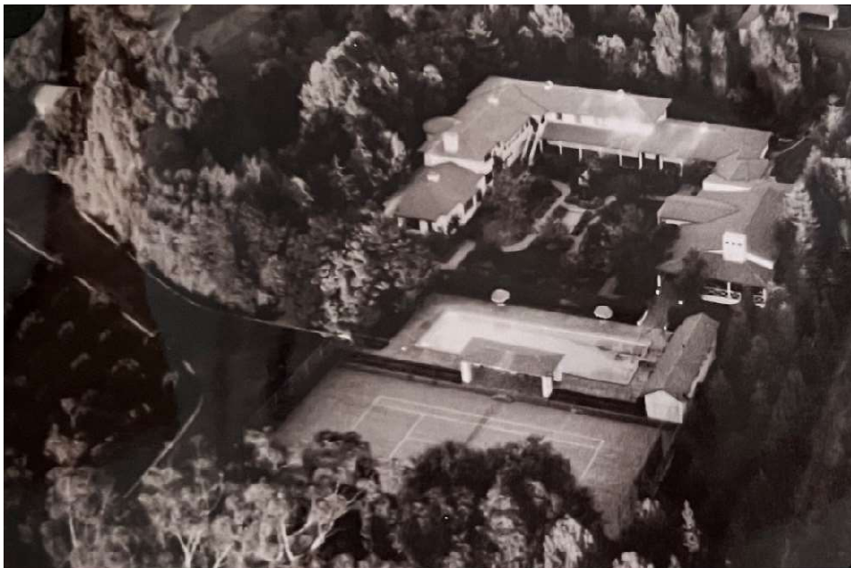
1940 oblique aerial photograph of Morrison House, facing east. Source: Westminster Gardens.
