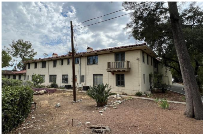
East Façade of Central Block, facing west.
