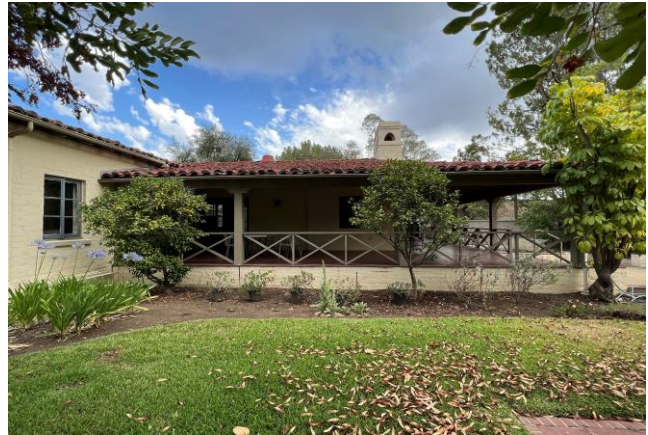
North Façade of South Wing, facing south.
