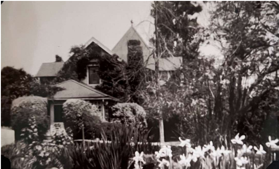
Santa Fe Station, first summer residence of Morrison family in Duarte (demolished), circa 1914. Source: Westminster Gardens.
