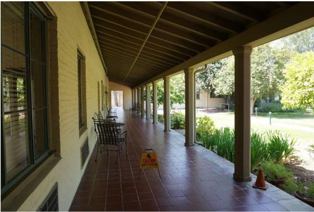
Colonnade on West Façade of Central Block, Morrison House, facing southeast.
