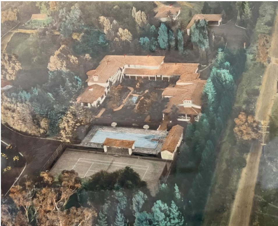
Oblique aerial photograph of Morrison House, facing east, 1940. Source: Westminster Gardens.
