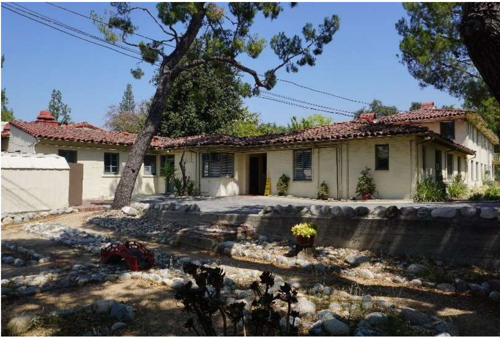
South Façade of Central Block and East Façade of South Wing, Morrison House, facing northwest.
