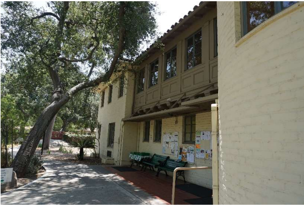
North Façade of North Wing, Morrison House, facing southeast.
