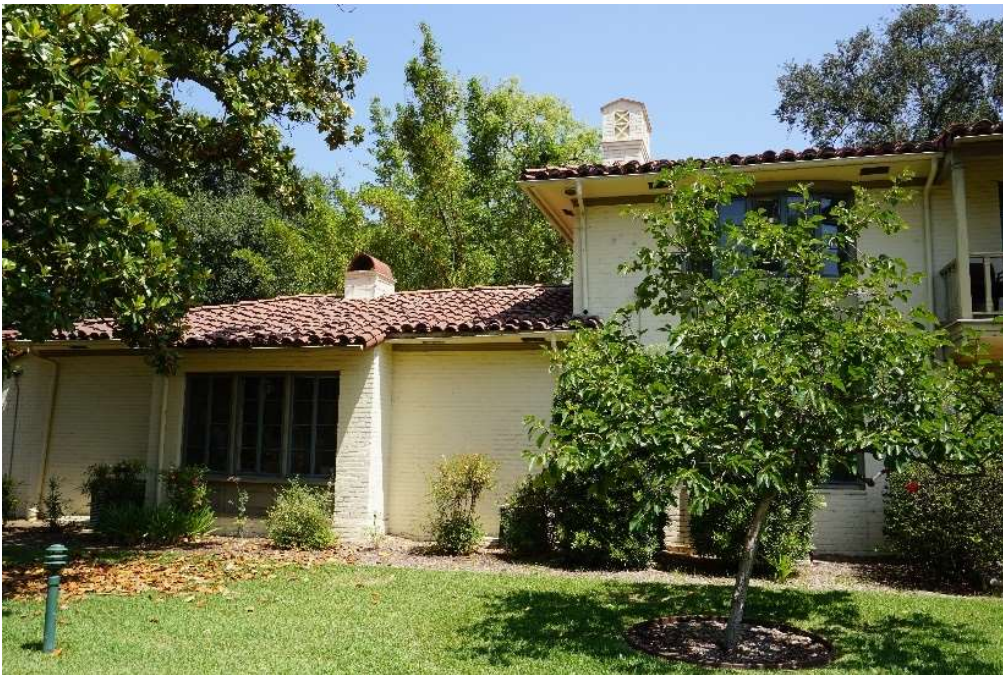
South Façade of North Wing, Morrison House, facing north.
