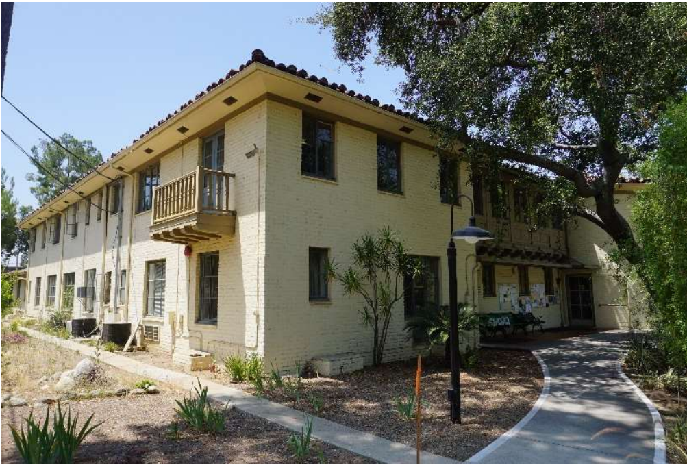
North Façade of North Wing and East Façade of Central Block, Morrison House, facing southwest.
