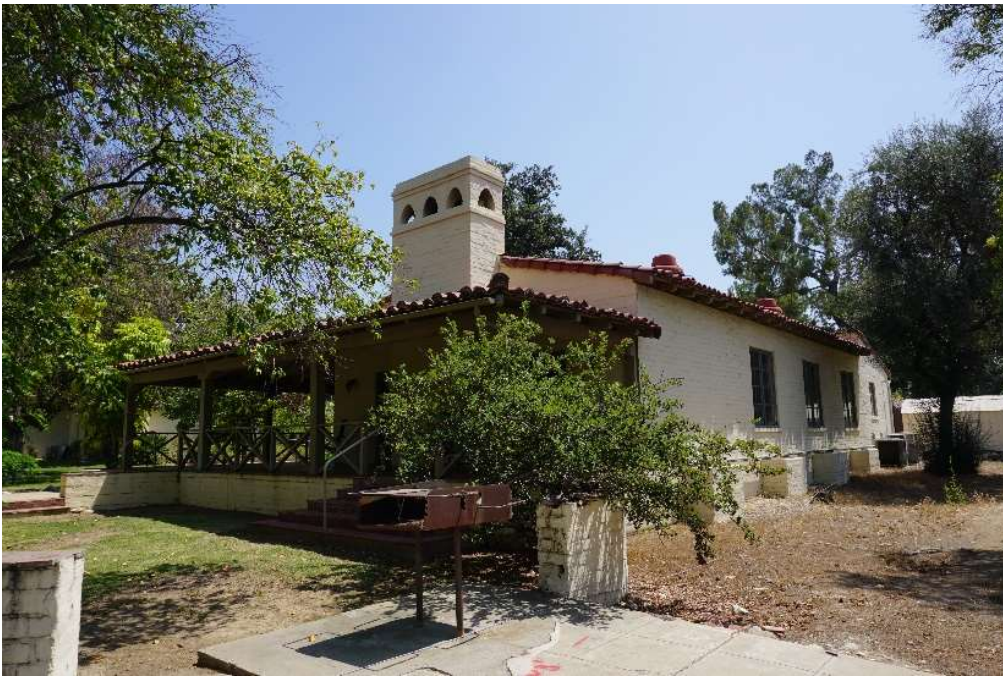
South and West Facades of South Wing, Morrison House, facing northeast.
