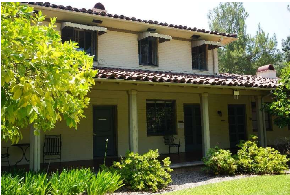
Colonnade on West Façade of Central Block, Morrison House, facing east.
