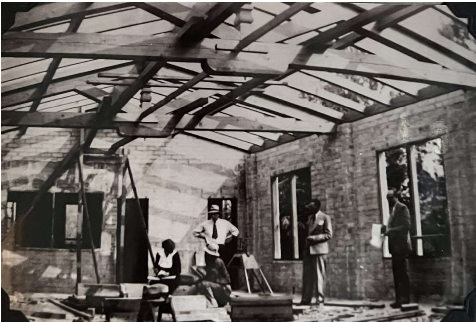
Construction of South Wing (El Sueño) of Morrison House, Lucile Morrison with builders, 1935. Source: Westminster Gardens.
