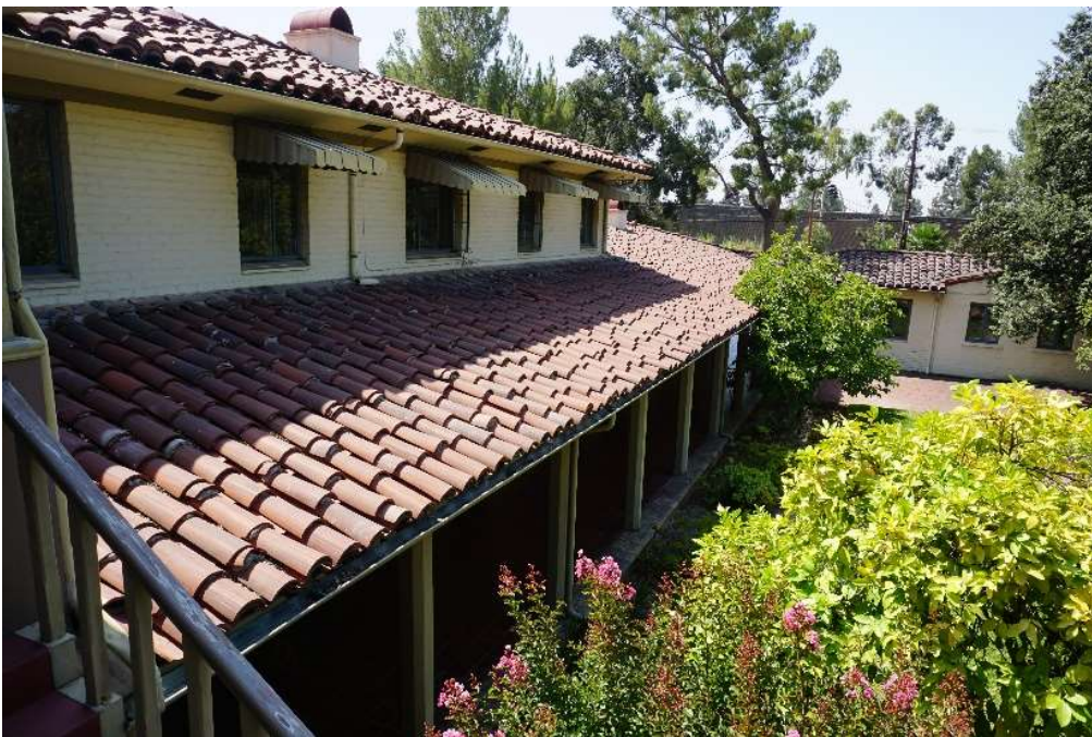
West Façade of Central Block, Morrison House, facing south.
