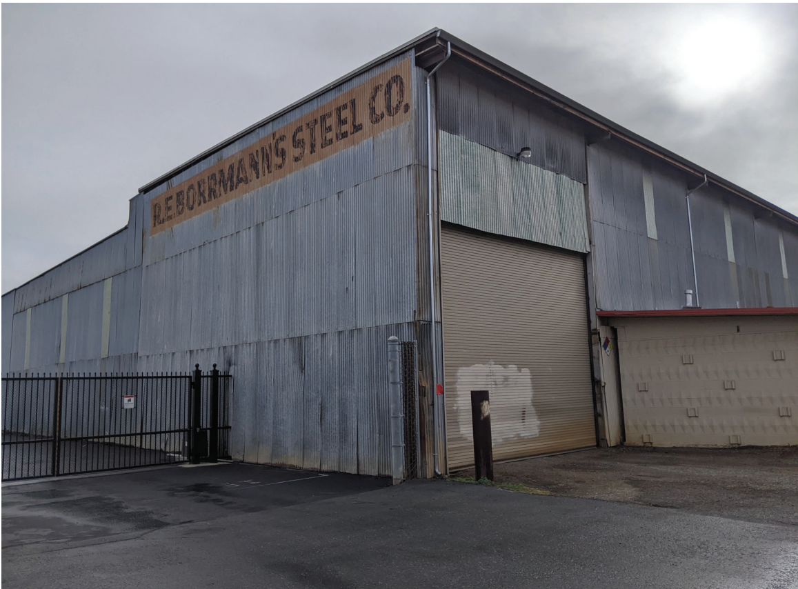
Photo 4: Industrial Uses adjacent to the south of the project site.
