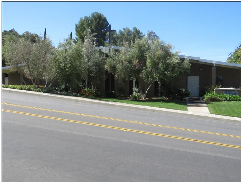
Figure 5-5. GC-001: Historic-period religious building (view south; April 8, 2022).
