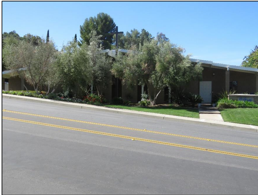
Photo 3. Grace Church building (view south; April 8, 2022).
