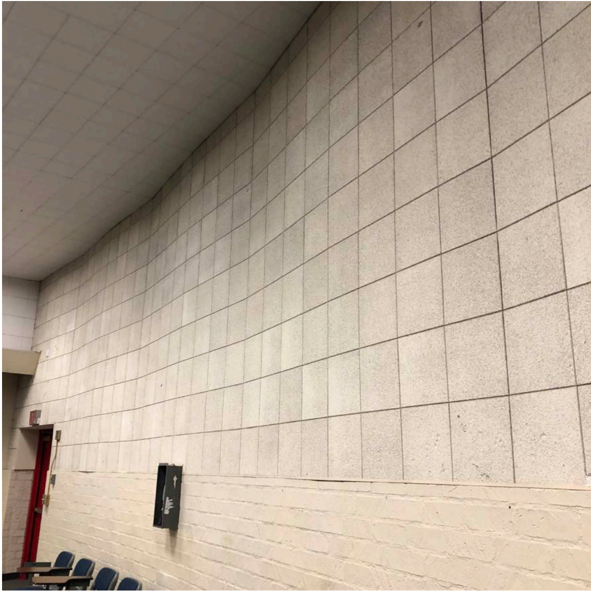
Auditorium wall tiles – no asbestos detected.
