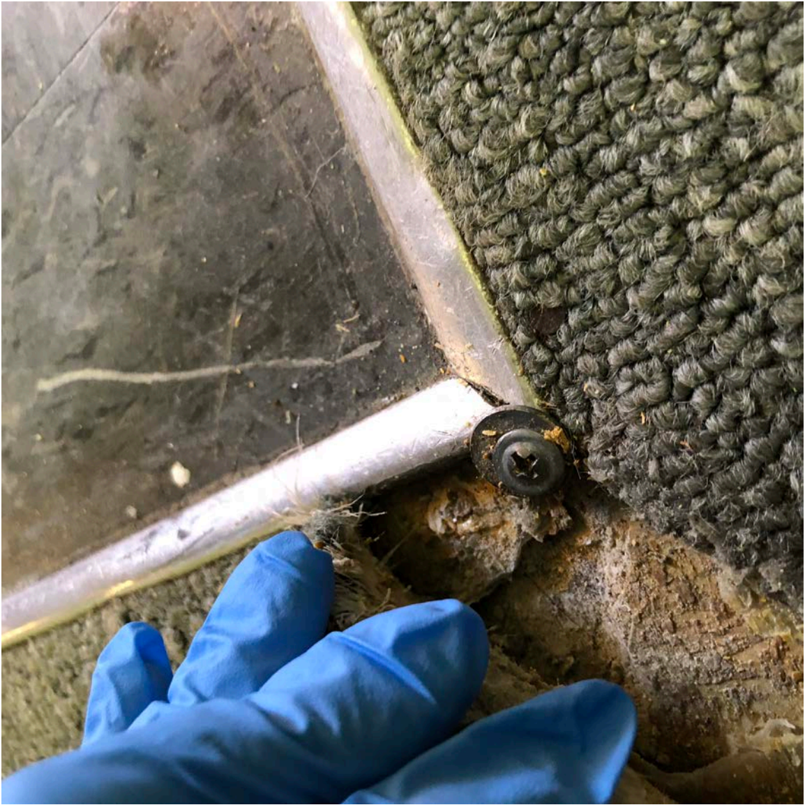
Beige 9-inch floor tile under carpet in Building B.
