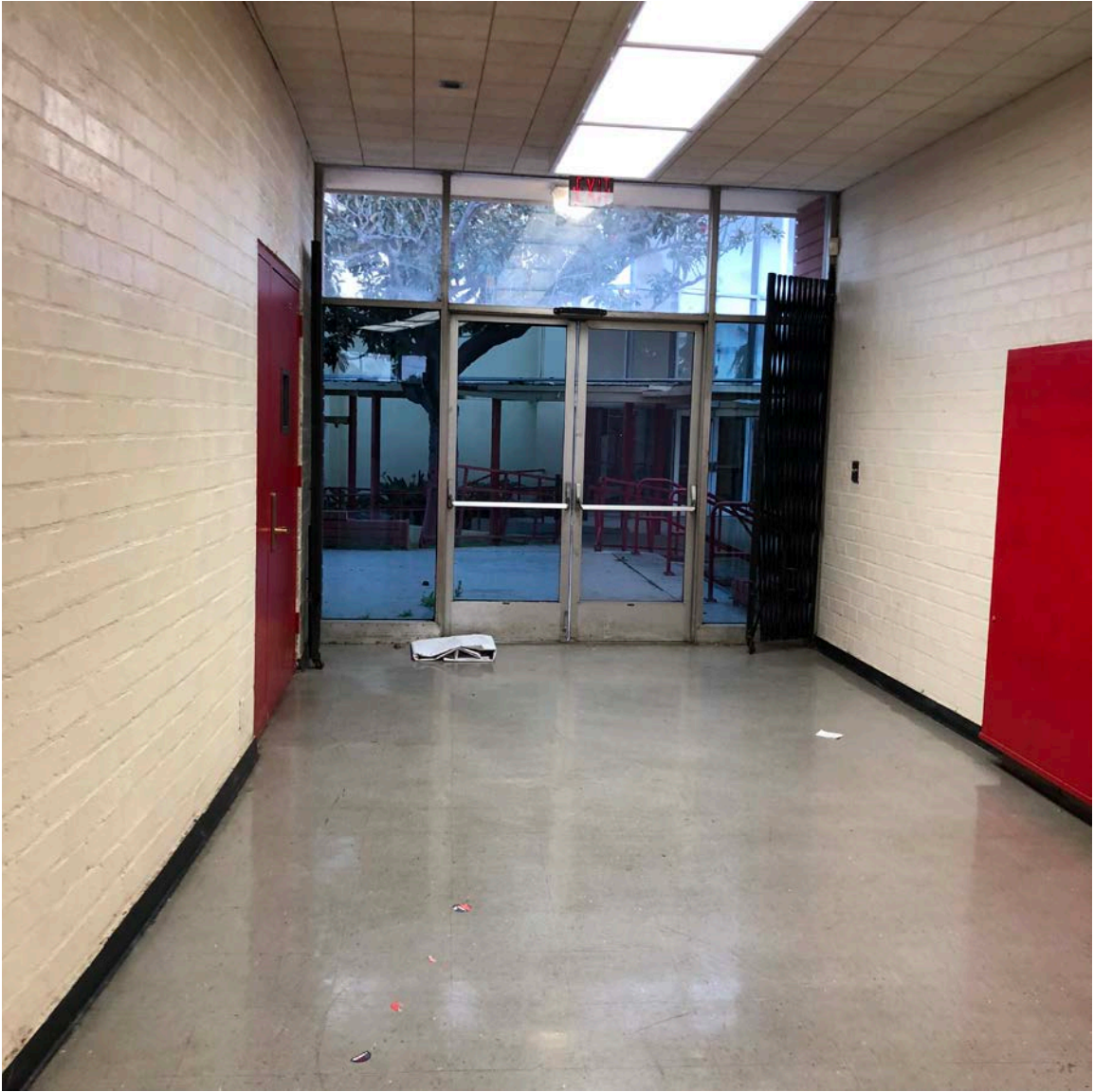
Building F lobby light fixtures.
