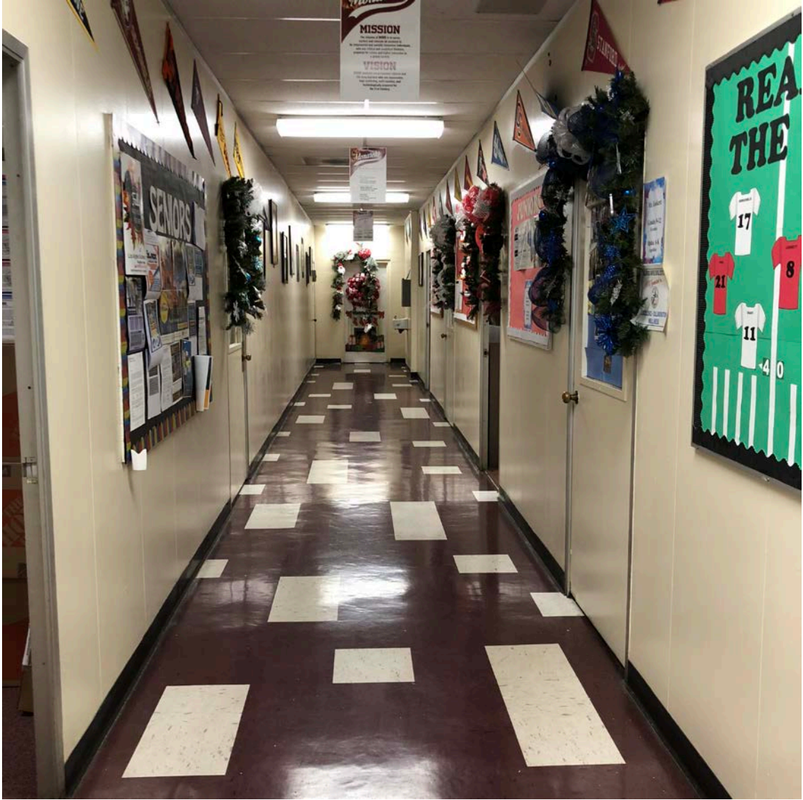
Building A corridor. Floor tile and cove base samples were negative for asbestos.
