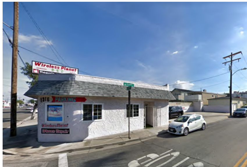
This lot within the Aviation Corridor is approximately 100 feet deep. The building is only 900 square feet, and the remainder of the property is dedicated to off-street parking.
