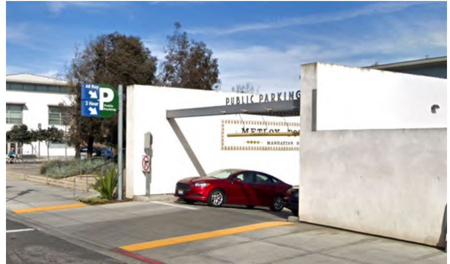
Introducing low-profile parking structures is a long-term solution to meeting parking demand while reducing on-site parking requirements and improving the pedestrian experience within the AACAP area.
