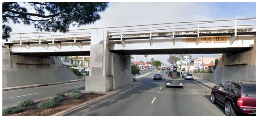
The eastern boundary of the Artesia Corridor passes under the transit easement, presenting an opportunity to create a memorable arrival experience.
