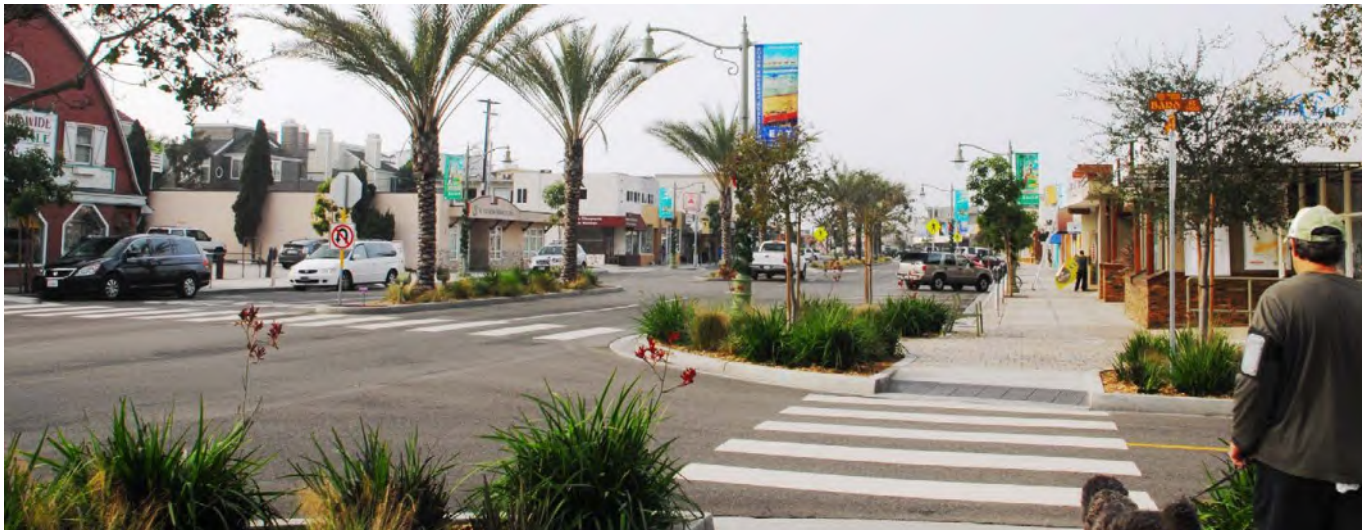
Bulb-outs at crosswalks with high-visibility continental striping improve pedestrian safety by limiting exposure to vehicles.
