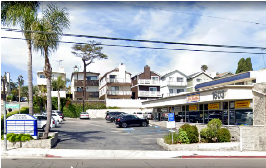
This commercial center, built in the 1970s, is small scale and auto-oriented. Note the orientation and relationship of the residential uses adjacent to the site.
