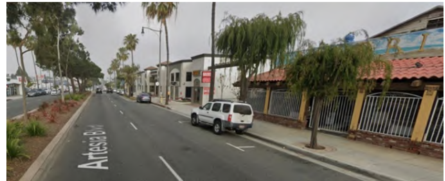
Artesia Boulevard currently is configured as two lanes with on-street parking. If a bike lane were to be introduced, adjustments to the median or the sidewalk widths might be necessary to create a safe buffer for cyclists.
