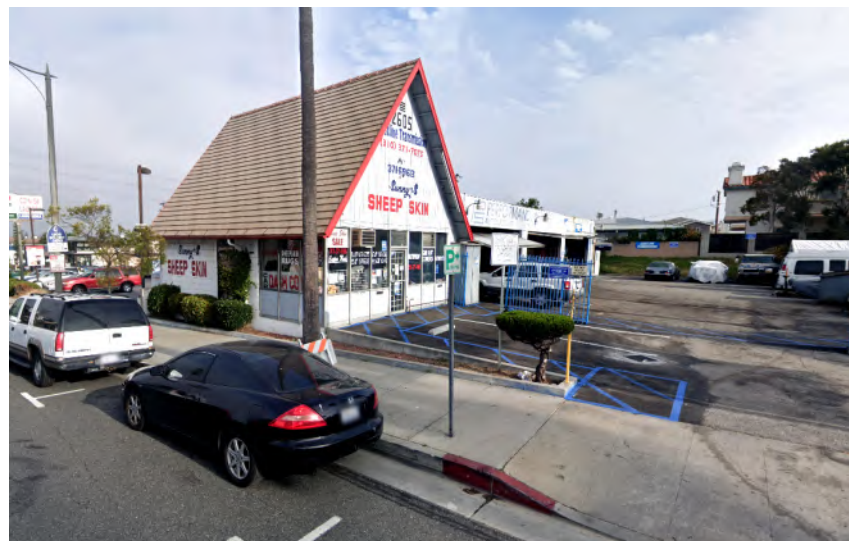
This A-frame structure with surface parking is characteristic of development along the Artesia Corridor in the 1960s.
