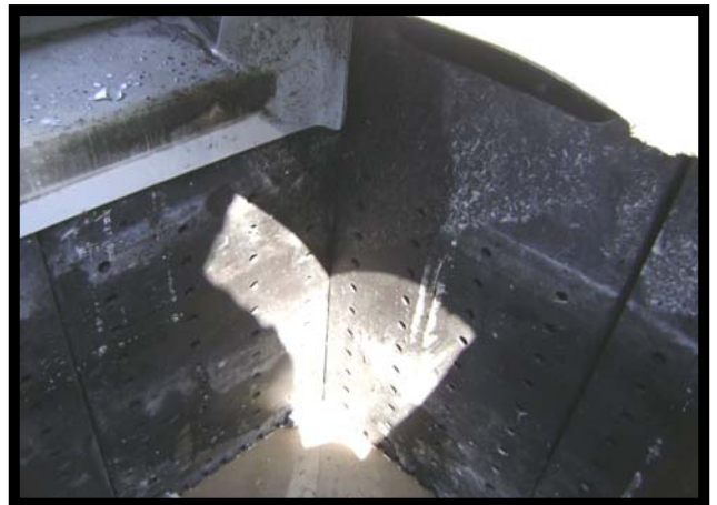
Replace Media Filter Panels And Lock Into Position.
