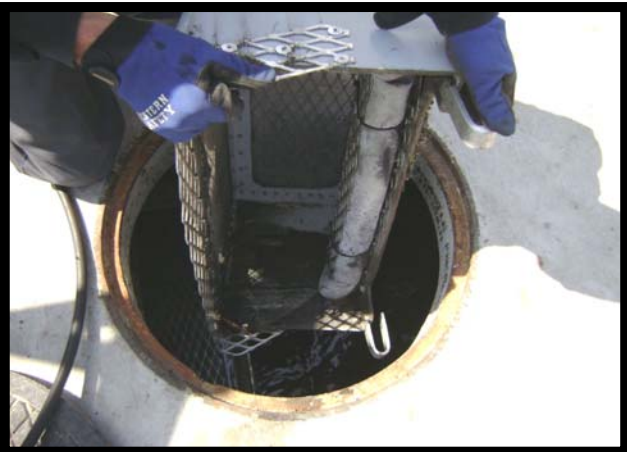
Cleaned Catch Basin Filters Are Removed Through Access Manhole To Allow For Unimpeded Access To Sediment Chamber.
