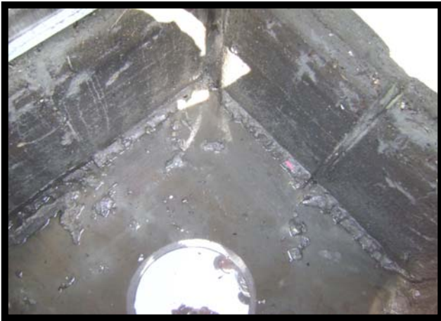
Exposed Filter Media Will Be Evaluated For Clogging And Loading Condition.
