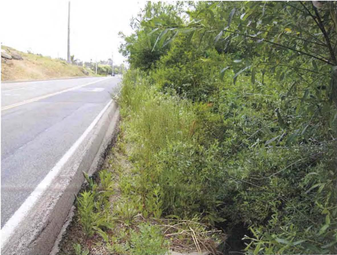
Figure 12. Looking Downstream along South Edge of Reach 3
