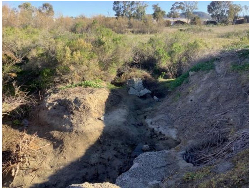
Figure 3. Drainage from sewer, view facing north.
