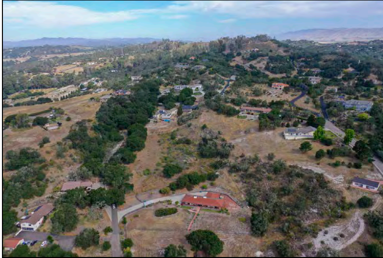
On Site Conditions - Surrounding property aerial.
