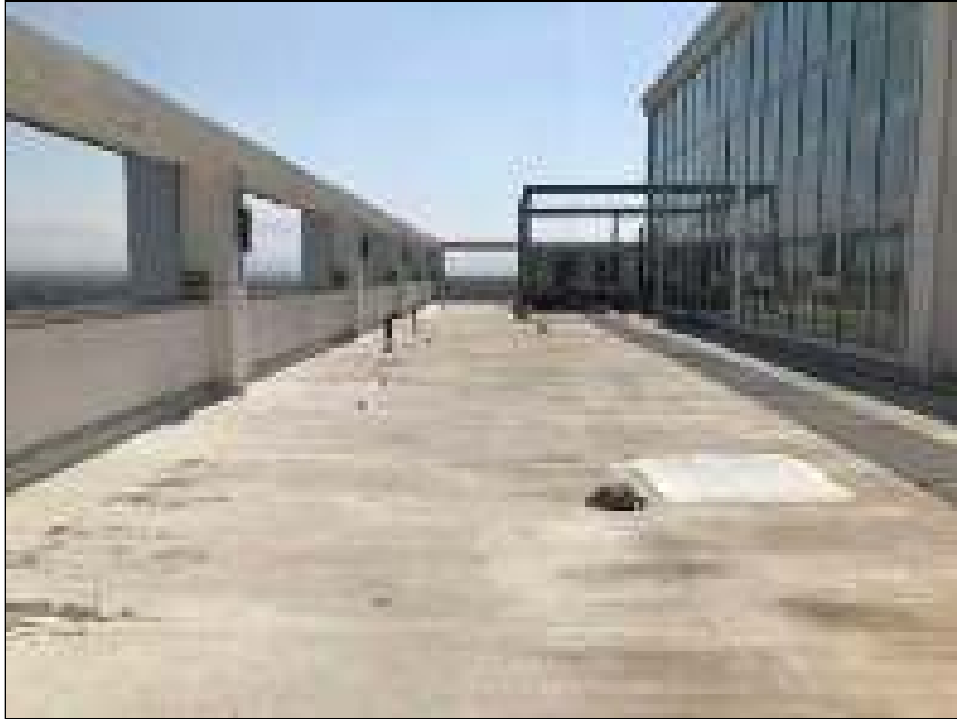
Photo 30: View of the roof.
