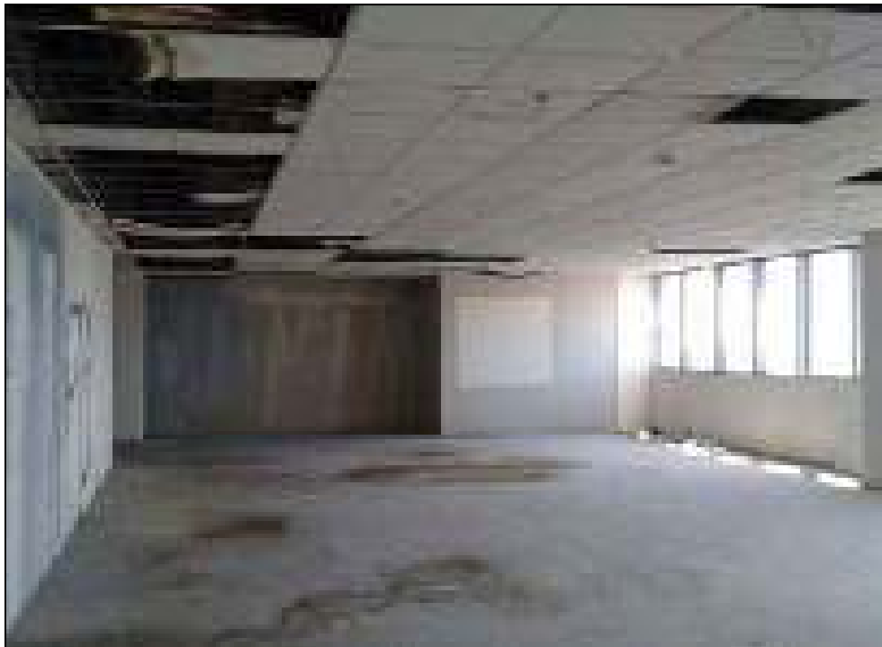
Photo 8: View of typical suite in office building
