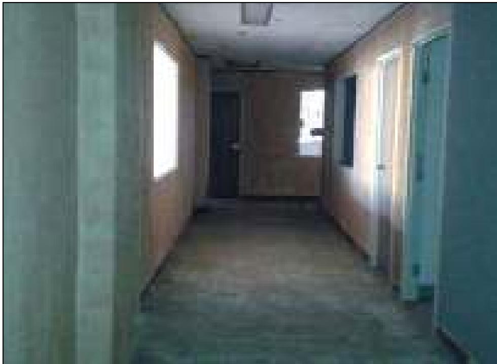
Photo 6: View of typical hallway in office building
