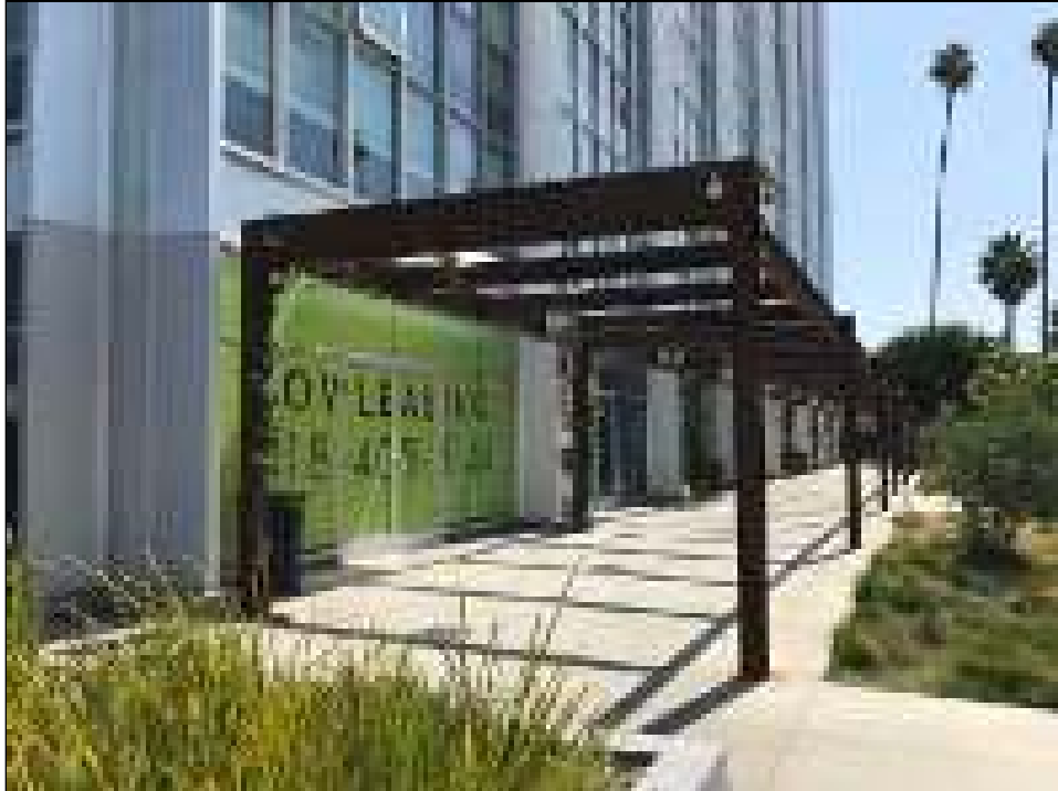
Photo 2: Additional view of the entrance to Panorama Tower.
