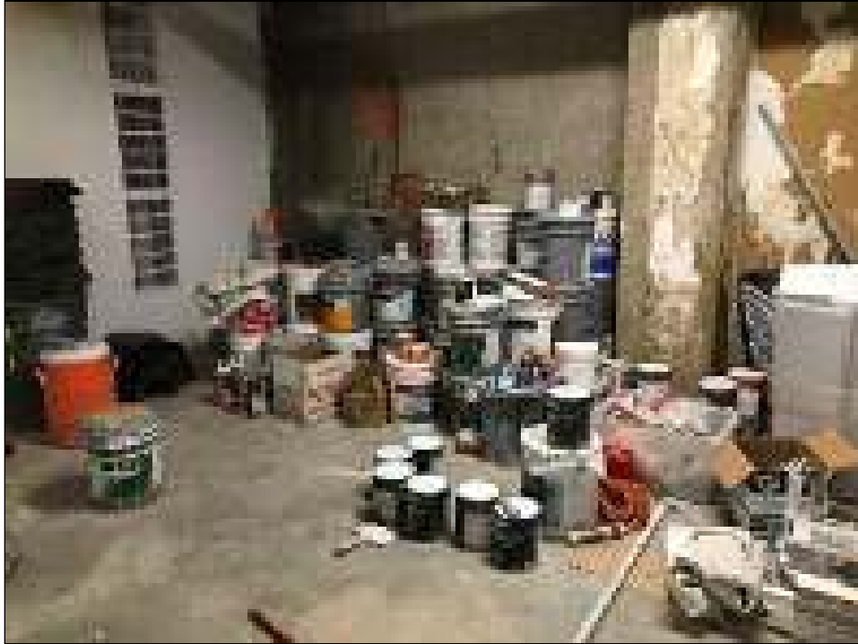
Photo 26: View of the storage and maintenance room (basement level).
