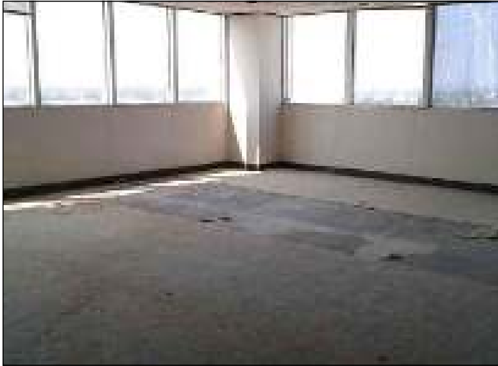
Photo 7: View of typical suite in office building
