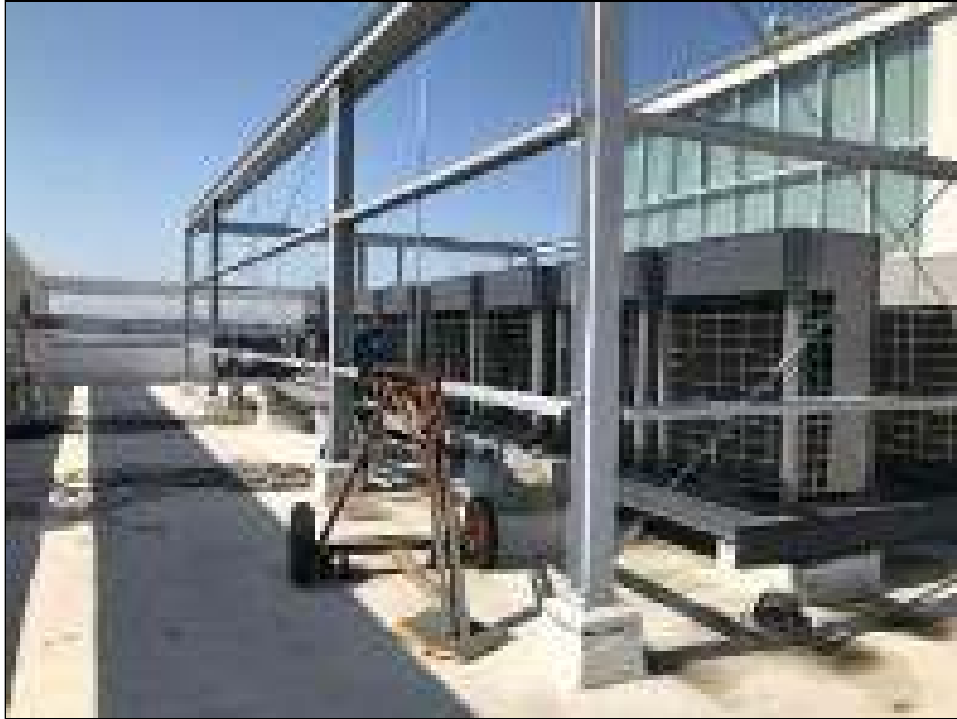
Photo 31: View of the roof and roof-mounted HVAC.
