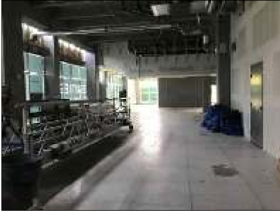
Photo 19: View of the undeveloped commercial space located on the ground floor.
