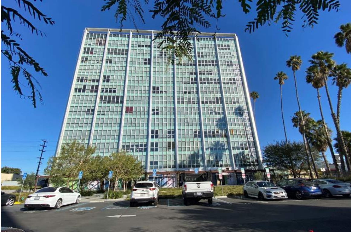
Figure 5: Panorama Towers, 8155 Van Nuys Blvd., south elevation, view north (Snow, 2022)
