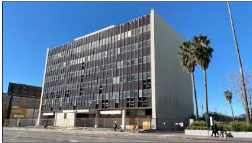
8121 Van Nuys Blvd, west façade, view southwest (Snow, 2022)
