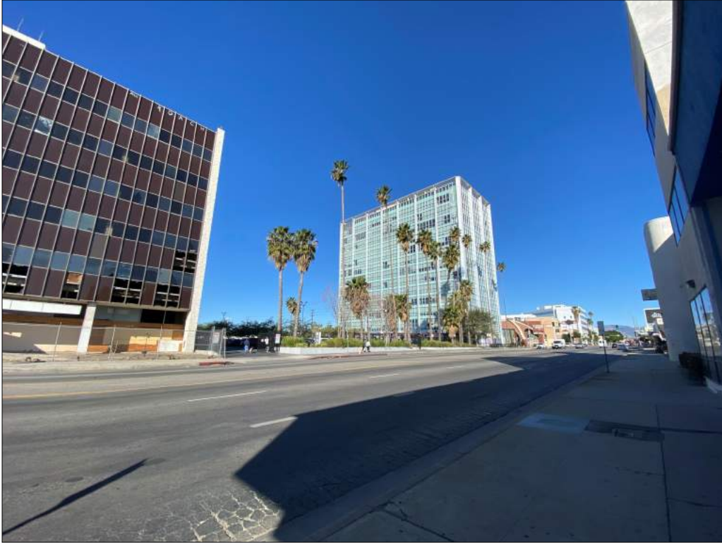
Figure 18: Panorama Plaza Building (right), Panorama Tower (center), and Panorama Bank Building (right), view northwest along Van Nuys Blvd. (Snow, 2022)
