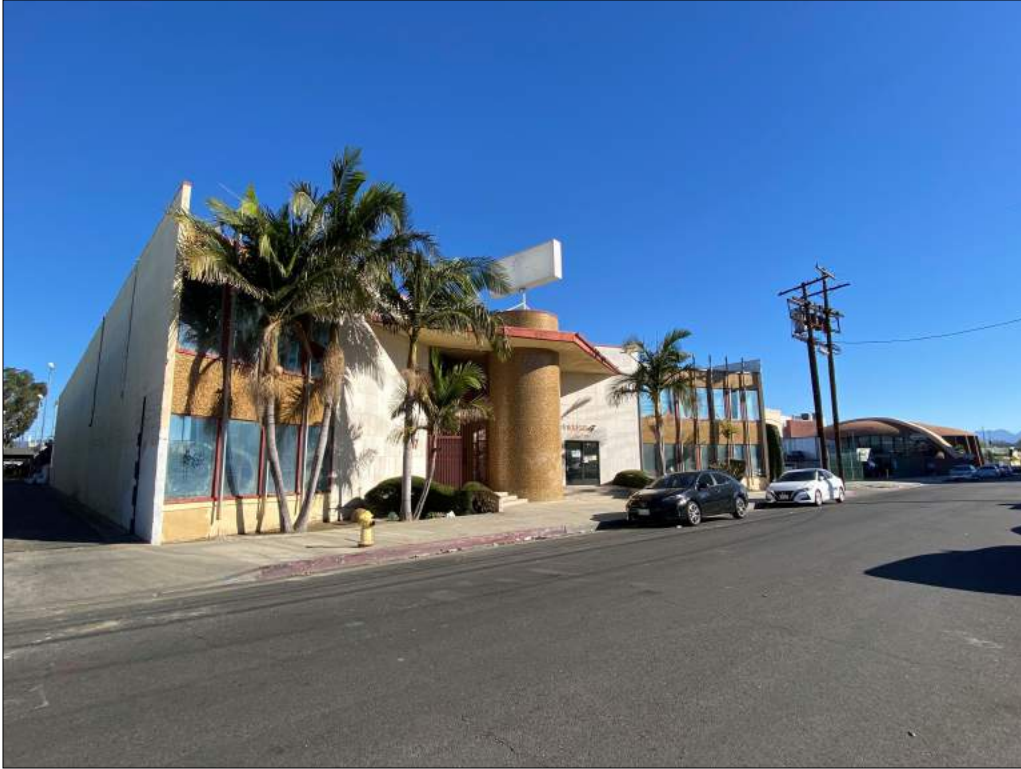
Figure 14: 14547 Titus St., west (left) and south (center) elevations, view northeast (Snow, 2022)
