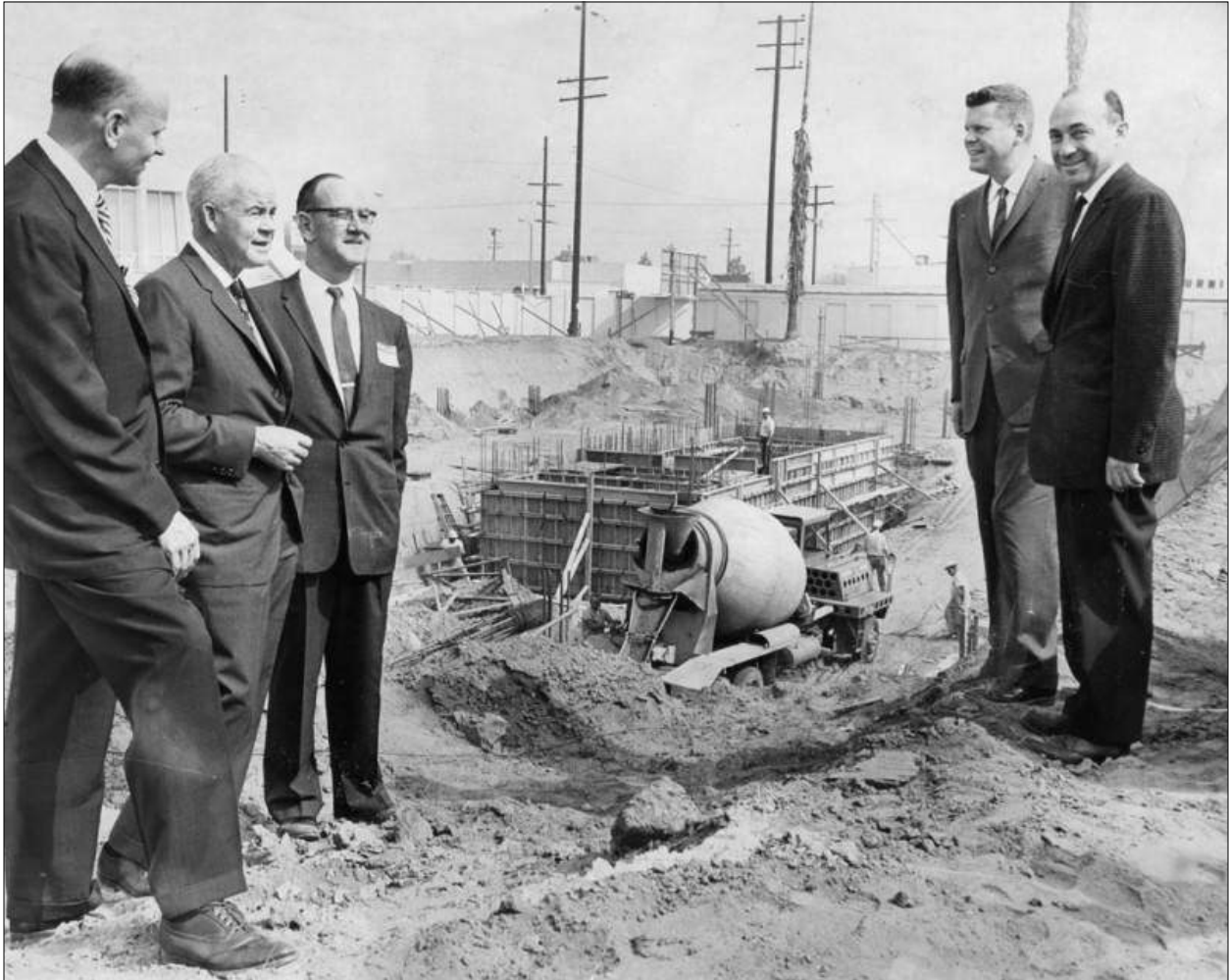
Historic Photo 3: Caption from The Valley Times reads: “Construction started on the above-ground phase of the first building of the $20 million, high-rise Panorama Towers project at Van Nuys boulevard and Titus avenue, Panorama City. The first building will rise 13 stories and will contain some 200,000 square feet of office space. Later, plans call for construction of another 13-story structure and a 20-story office facility... Included among those participating in the cement-pouring ceremony were: County Supervisor Warren M. Dorn, Councilman Ernani Bernardi, Welton Becket, architect on the project; William Brownyard, developer, and Henry C. Beck, Jr., contractor.” (source: Los Angeles Public Library, 1961)
