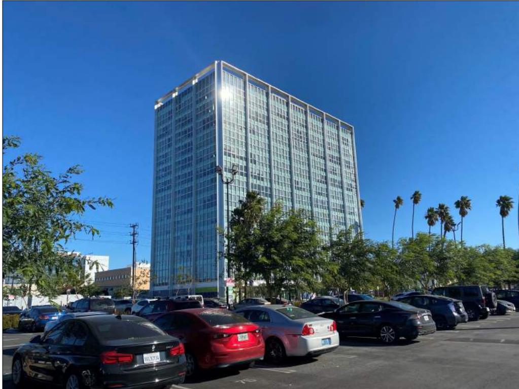
Figure 4: Panorama Towers, 8155 Van Nuys Blvd., east (left) and south (right) elevations, view northeast (Snow, 2022)
