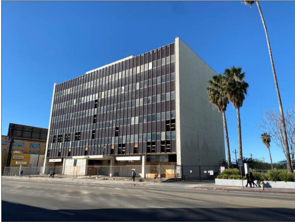
Figure 16: Panorama Plaza Building, 8121 Van Nuys Blvd., east (left) and north (right) elevations, view southwest (Snow, 2022)
