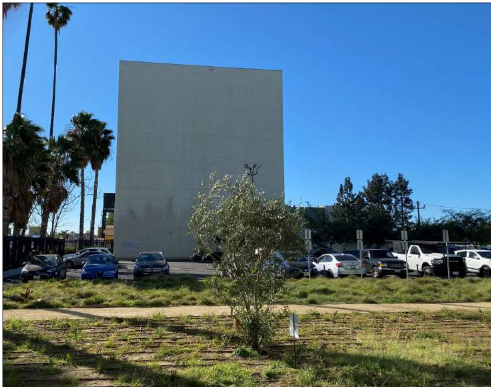
Figure 17: Panorama Plaza Building, 8121 Van Nuys Blvd., north elevation from Panorama Plaza, view south (Snow, 2022)
