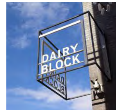
1: CORNER SIGN WITH 1" DEEP STEEL CUT OUT LETTERING, 1'-2" HIGH LETTER
