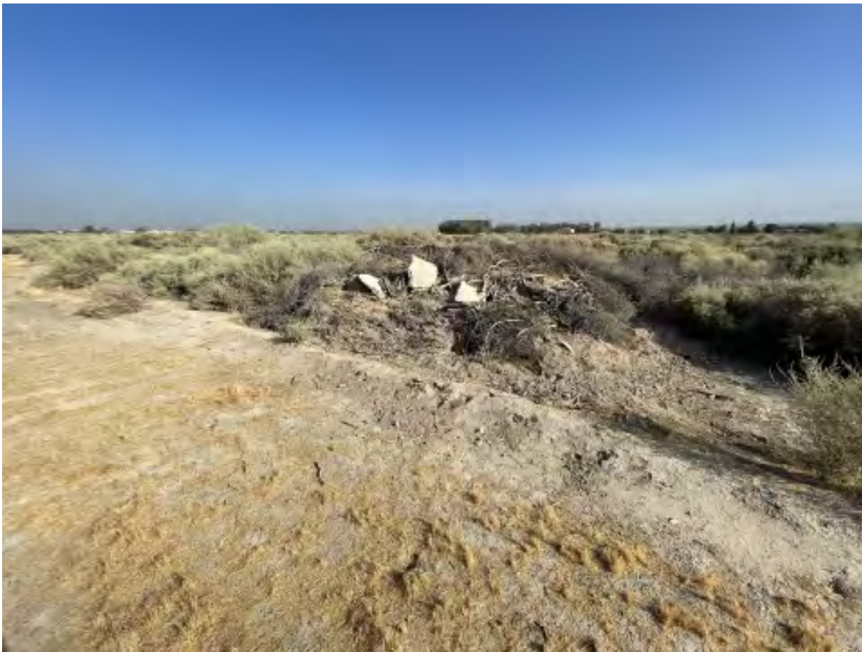
Picture 22 Looking at another pile with concrete, vegetation, and soil along the southern border.
