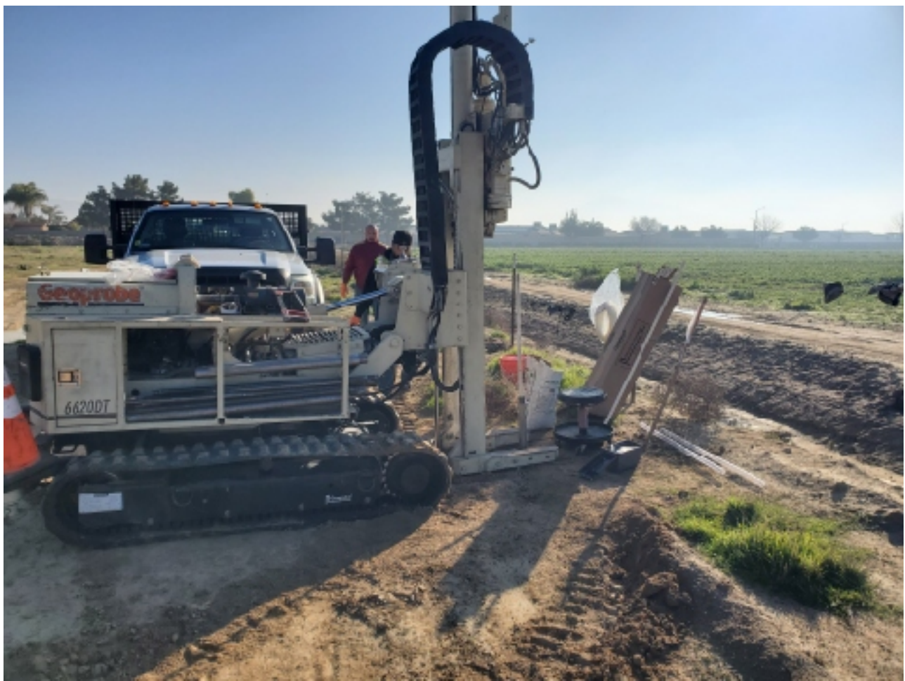
GeoProbe Rig Drilling at SG-1
