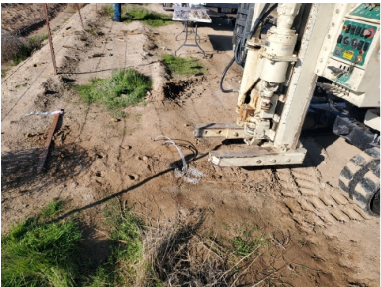
3 Finished Vapor Probes at SG-1
