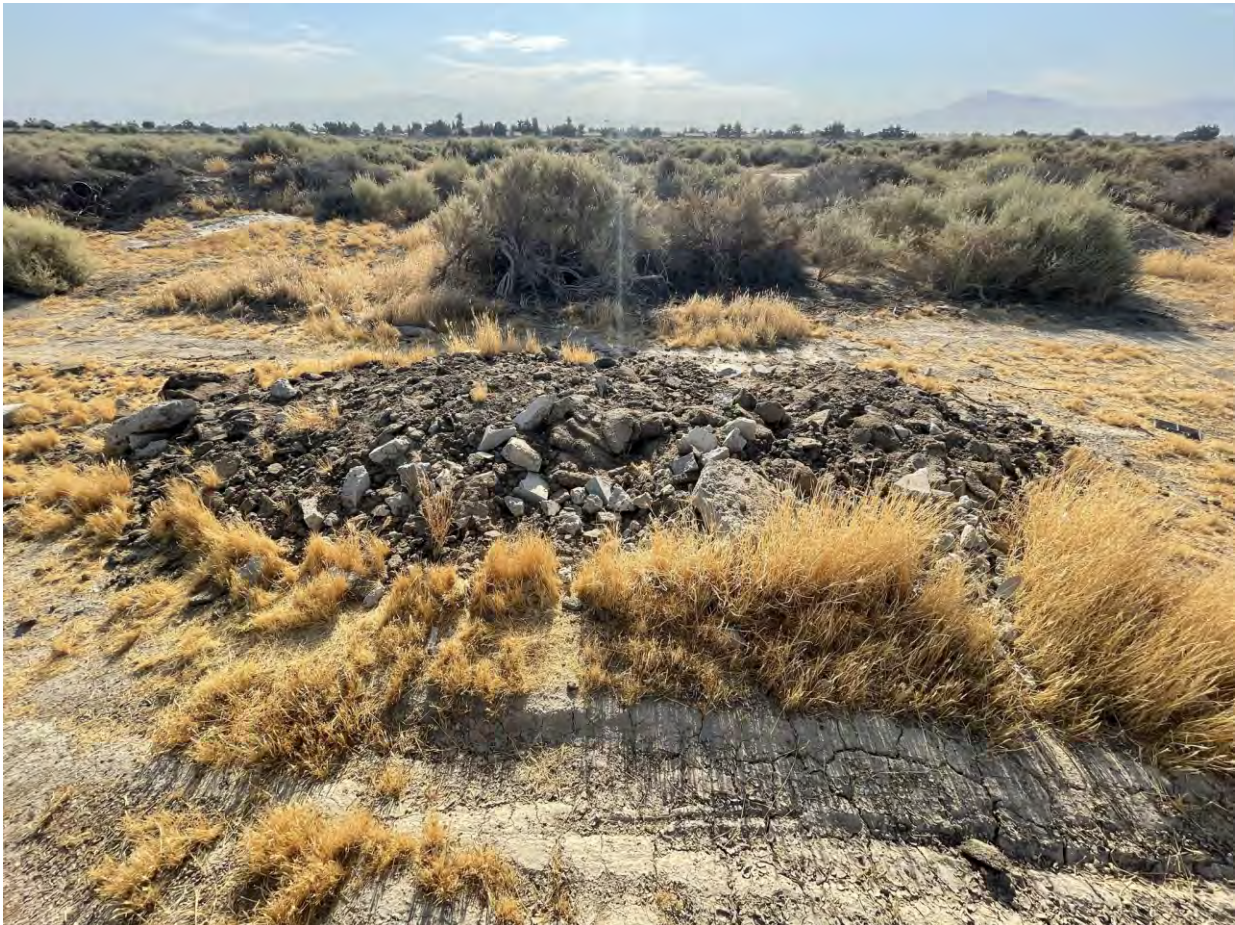
Picture 25. Looking at a concrete pile in the NW portion of the site.
