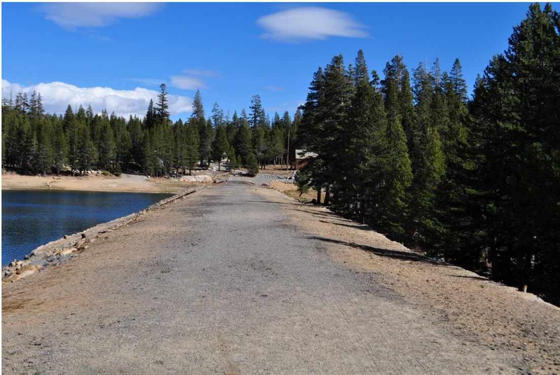
Key View 4. View from the western end of the dam looking east across the dam crest.
