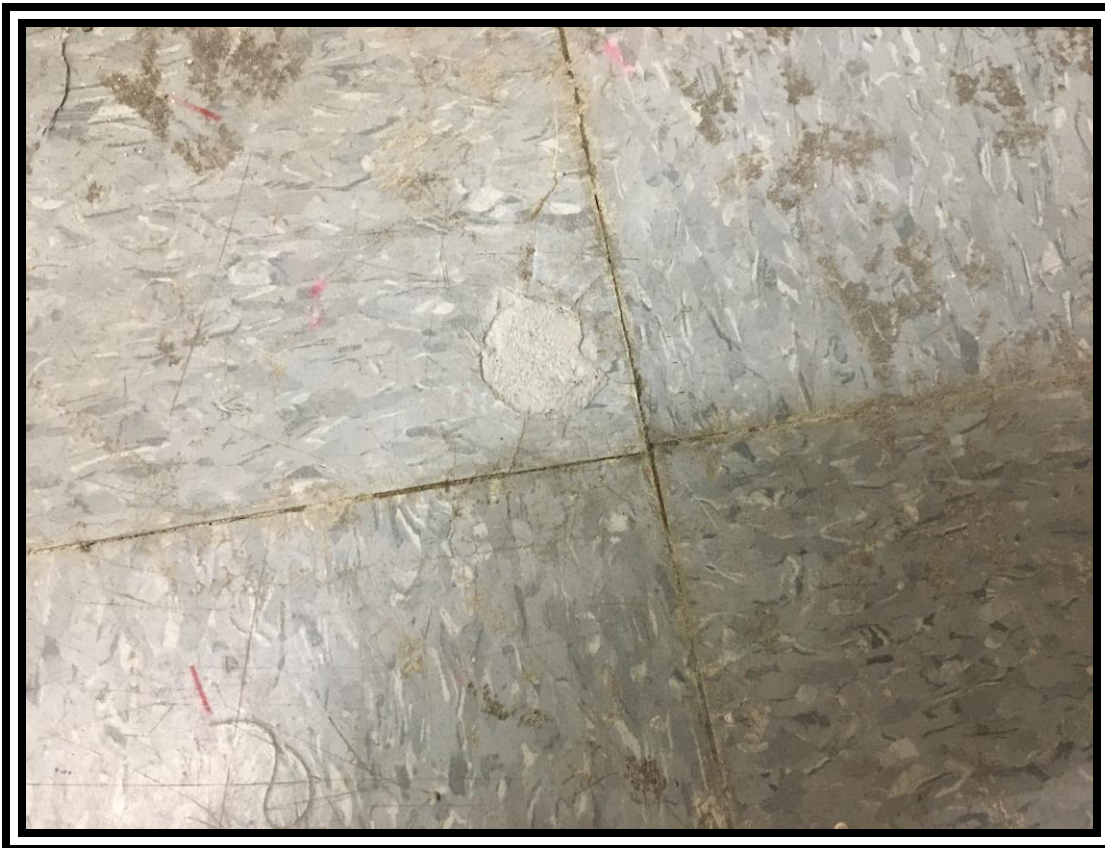
4. FINISHED PROBE LOCATION SV-2 INSIDE SOUTH AREA OF UNIT.
