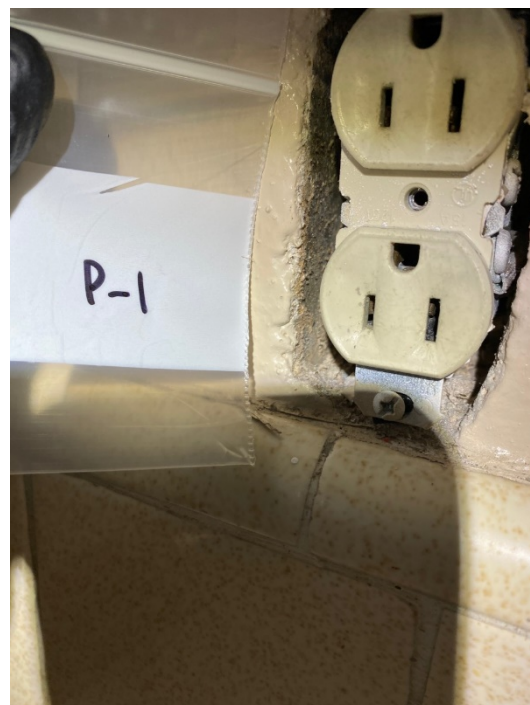
Picture 2: Plaster sampled was found to not contain asbestos
