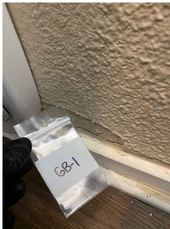
Picture 4: Gypsum board sampled was found to not contain asbestos
