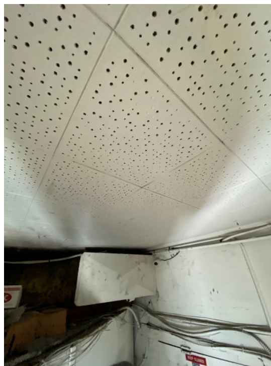
Picture 2: Ceiling tile sampled was found to not contain asbestos
