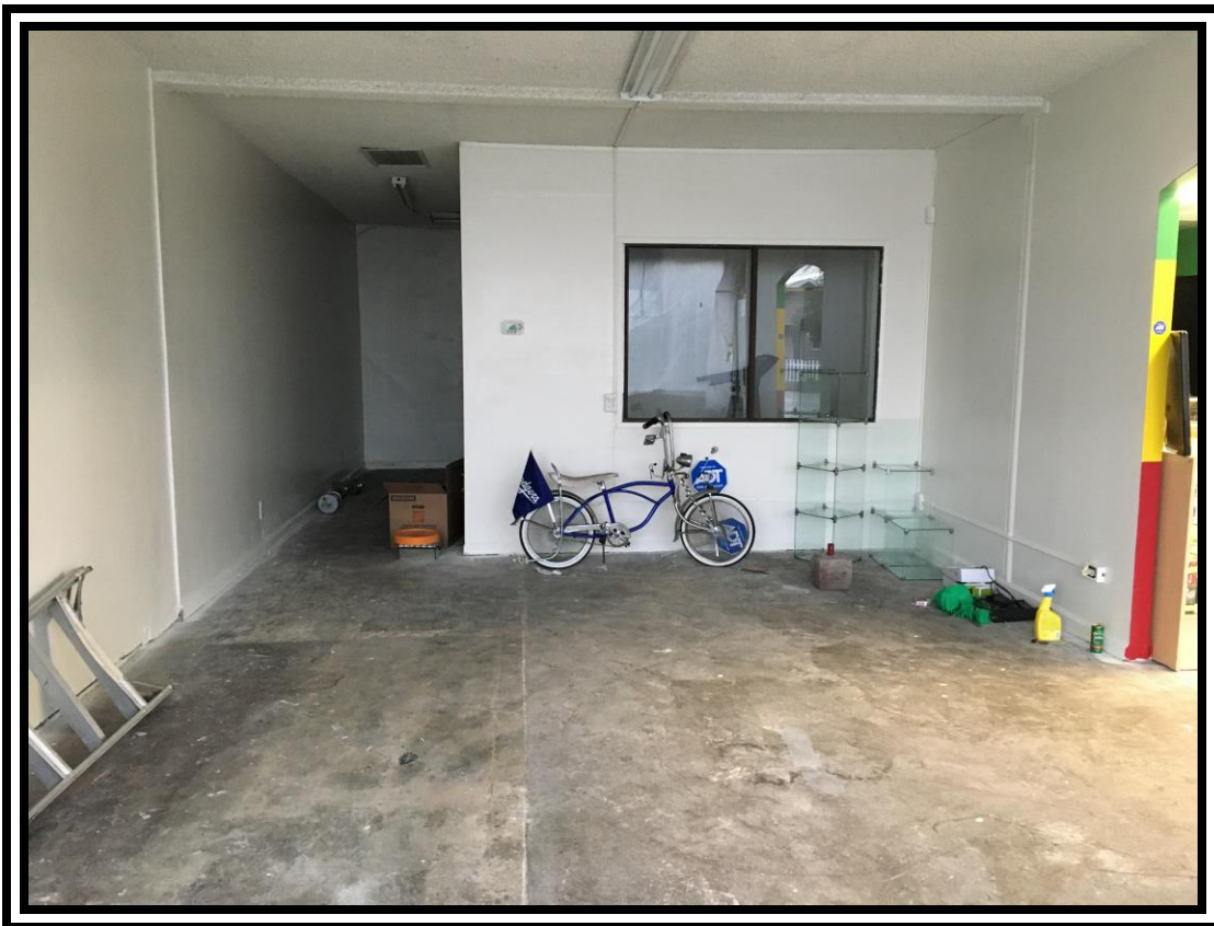
4. 6014 S. NORWALK BUILDING INTERIOR AT EAST AREA (VACANT).
