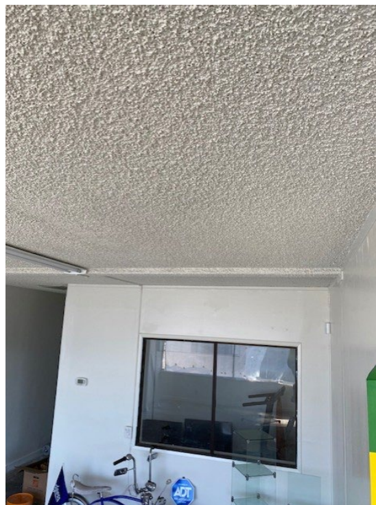
Picture 2: Acoustic ceiling sampled was found to not contain asbestos
