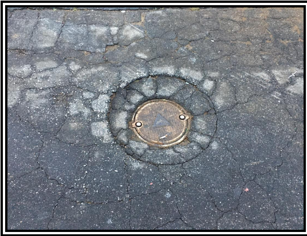
21. GROUNDWATER MONITORING WELL MW-9 IN ADJACENT WEST ALLEY, ASSOCIATED WITH ARCO CASE LOCATED ADJACENT EAST OF PROPERTY.
