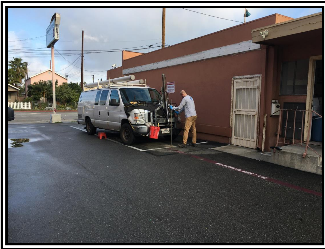
6. ADVANCING PROBE LOCATION SV-5 AT WEST SIDE OF BUILDING.
