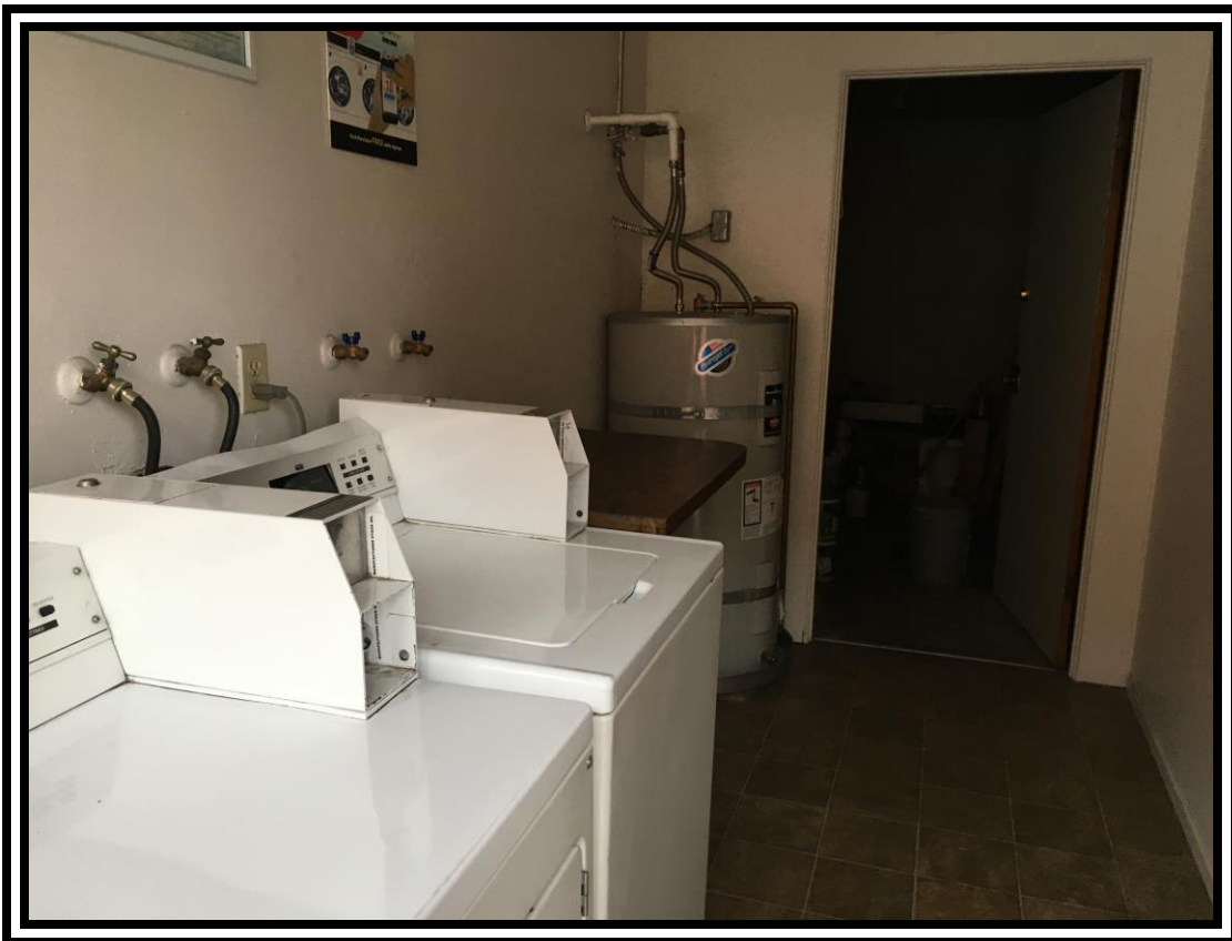
6. LAUNDRY ROOM AT 6016 S. NORWALK BUILDING.
