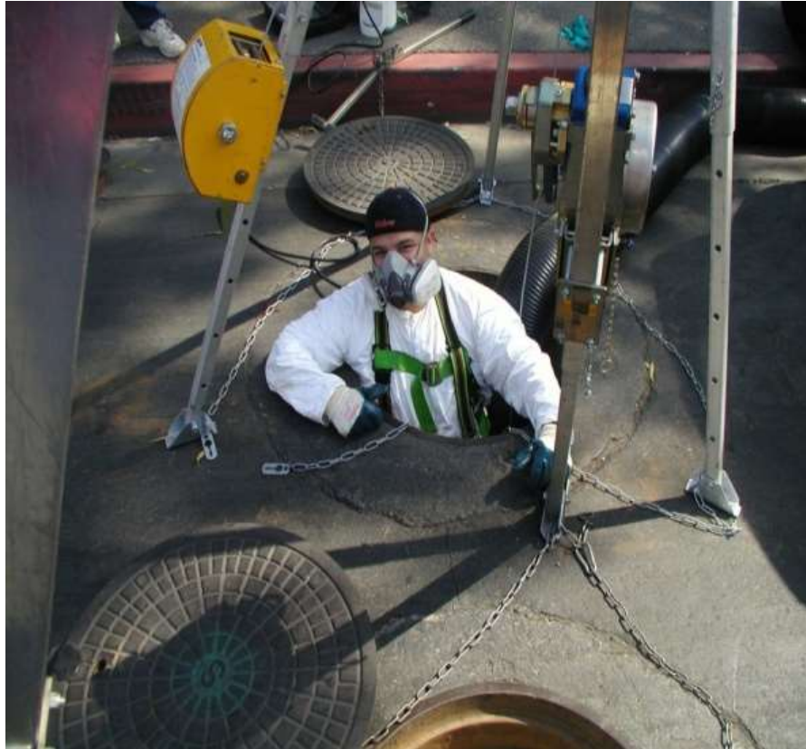
Figure: All technicians are certified for Confined Space Entry.
