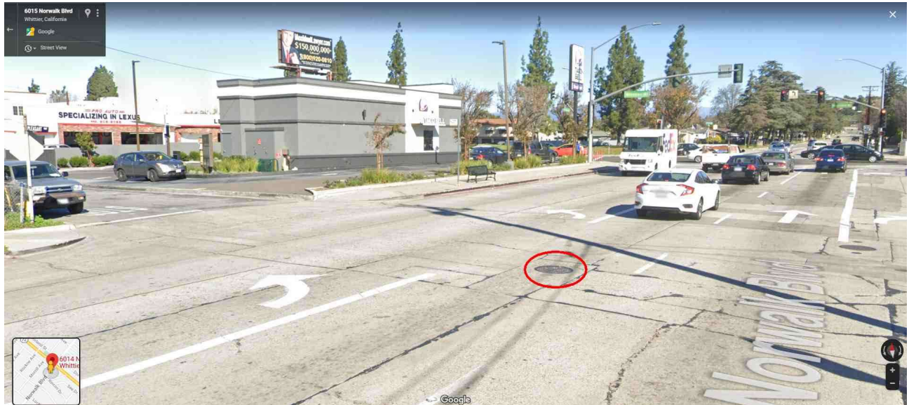
Figure 5 below: The photo shows City MH 25 in the left-hand northbound lane of Norwalk Blvd at its intersection with Pleasant Way. The manhole is northwest of 6014 Norwalk Blvd.
