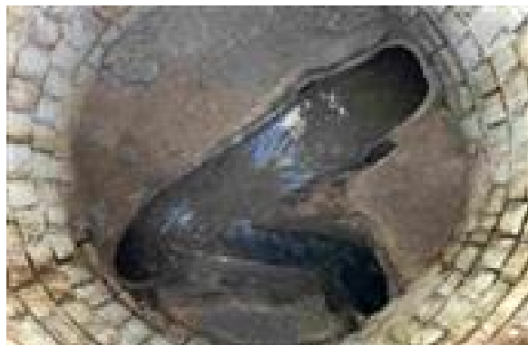
Manhole Before Install
