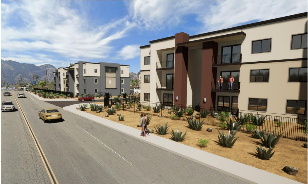
Above: View of entry access on Avenue 50.
