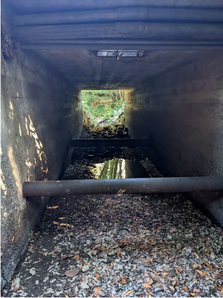
Photo 2. Tamalpais Creek Crossing 1 in Area 1. Photo taken October 6, 2022.
