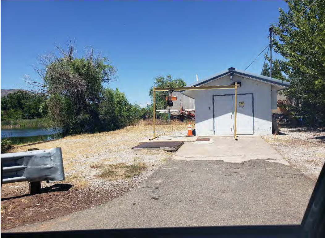
Image of Lift Station 1 (Bridge Street) showing perennial stream (Fall River) and barren habitats. View toward the northwest.
