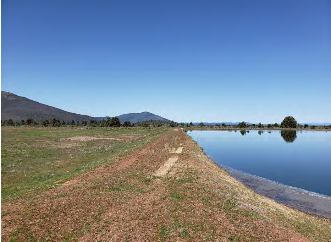
Image of the WWTP. View toward the north.
