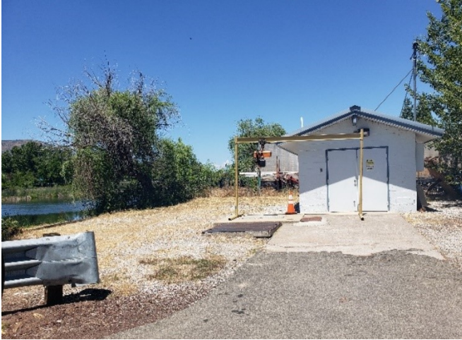
Photo 2. Lift Station 1 (Bridge Street)
