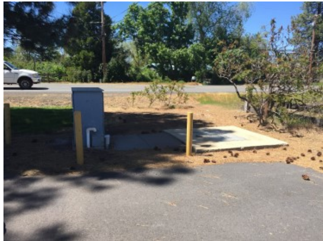
Photo 1. Lift Station 2 (Hospital)
