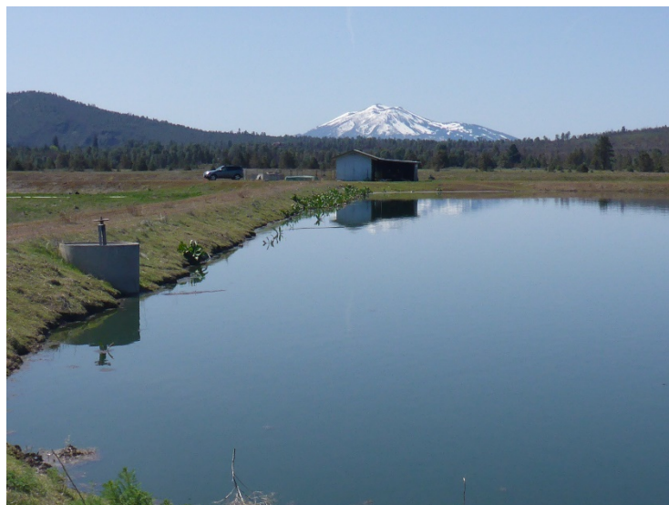
Photo 4. Wastewater Treatment Plant Pond
