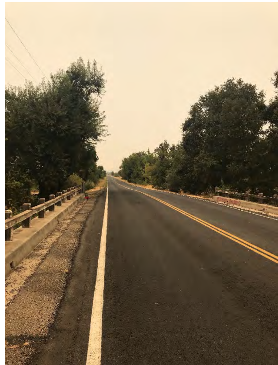
Photo 12: View to the southeast of the Project alignment along Rancho Road crossing Reed Creek.
