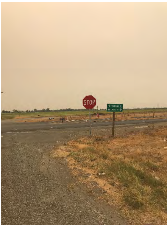
Photo 14: View to the south long the Project alignment of the intersection of Highway 65, Rancho Road, and Morrison Road.
