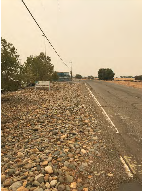
Photo 13: View to the northeast along the Project alignment of the PG&E facility on Rancho Road.
