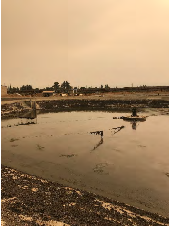
Photo 5: View of OPUD wastewater treatment facility retention basin.
