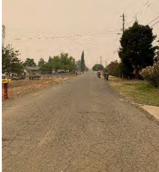
Looking south along Project alignment near Station 118+00.
