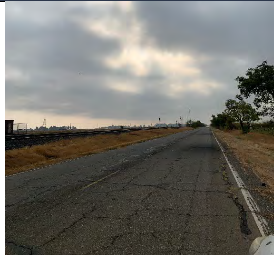
Looking southeast along Project alignment near Station 442+30.
