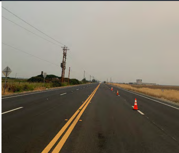
Looking north along Project alignment near Station 119+90.
