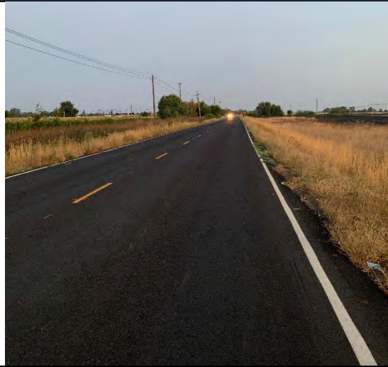
Looking northwest along Project alignment near Station 329+60.
