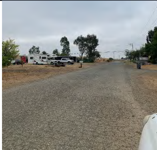
Looking south along Project Alignment towards intersection of Shimer Road and Plute Road near station 33+00.
