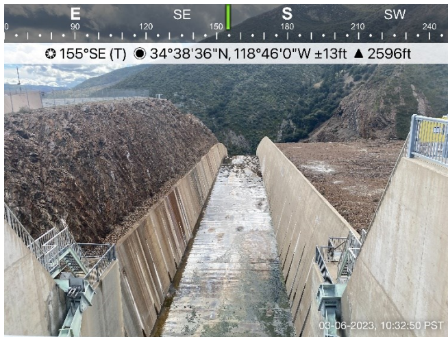
Photo 7. Looking south down spillway.
