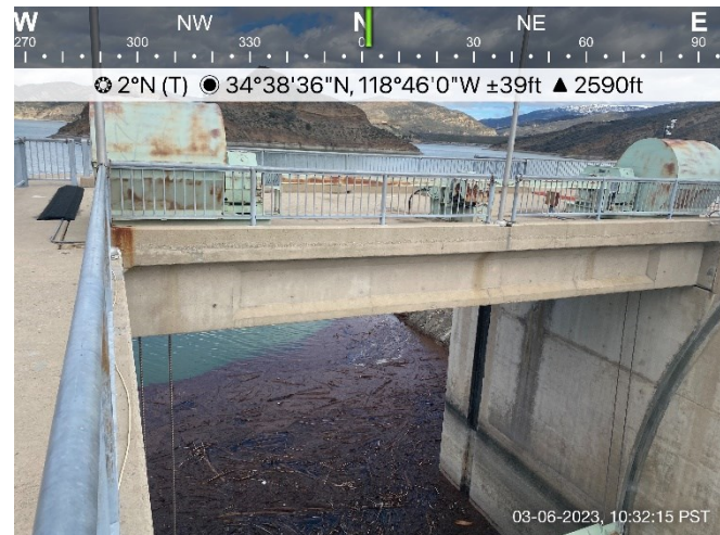
Photo 8. Looking upstream along the spillway.
