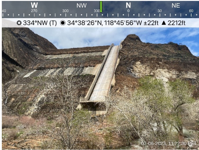
Photo 1. Looking towards base of spillway at scaffolding area.
