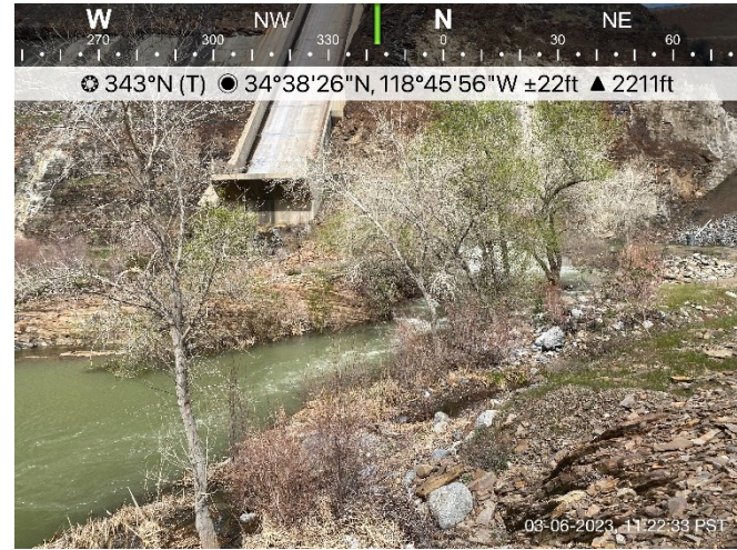
Photo 2. Looking at area to place scaffolding.
