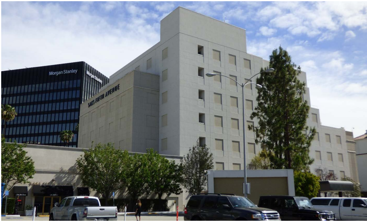
Image 15: South (rear) façade, view northeast from parking lot
