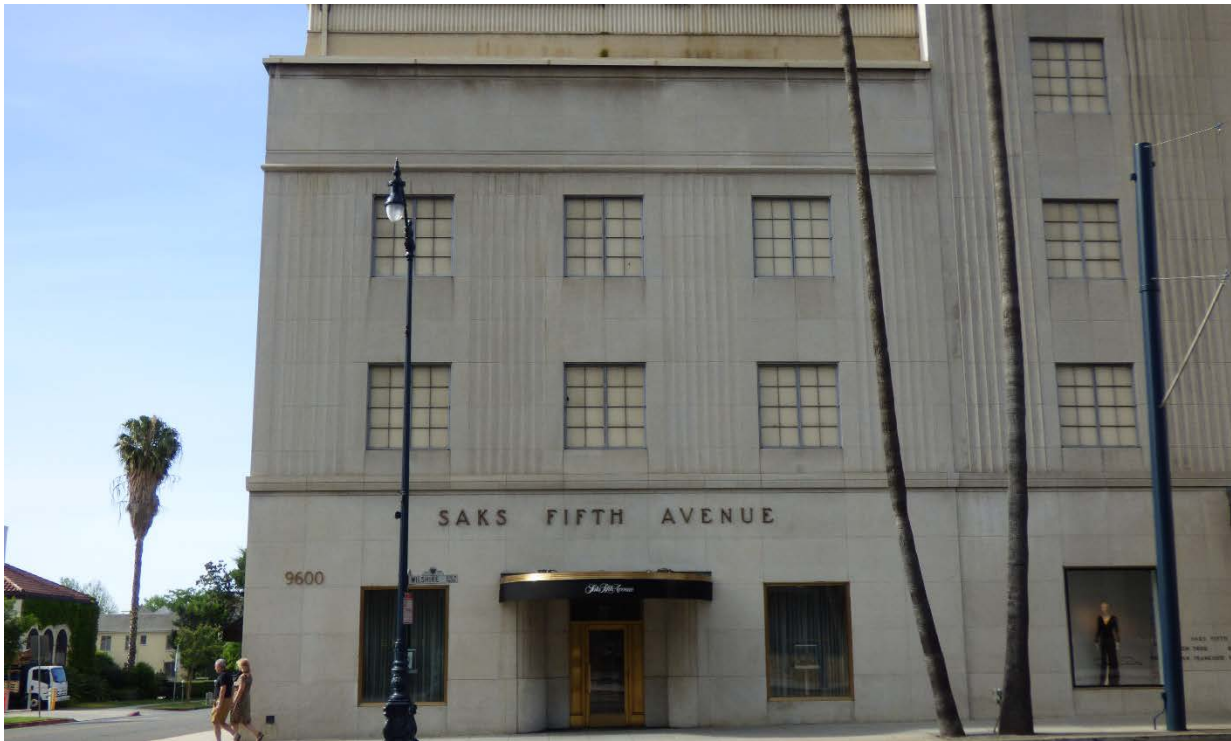
Image 3: Unit #1, north (primary) façade, view south from Wilshire Boulevard
