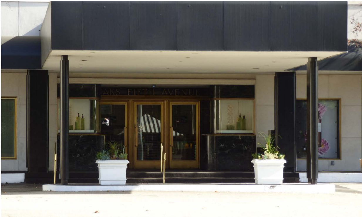
Image 16: South (rear) entrance, view northeast from parking lot
