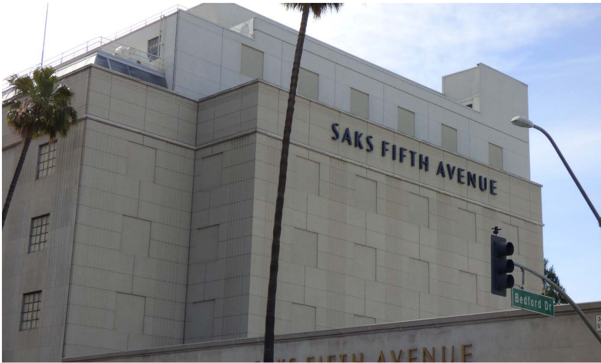
Image 13: Escalator tower, view southeast from Wilshire Boulevard
