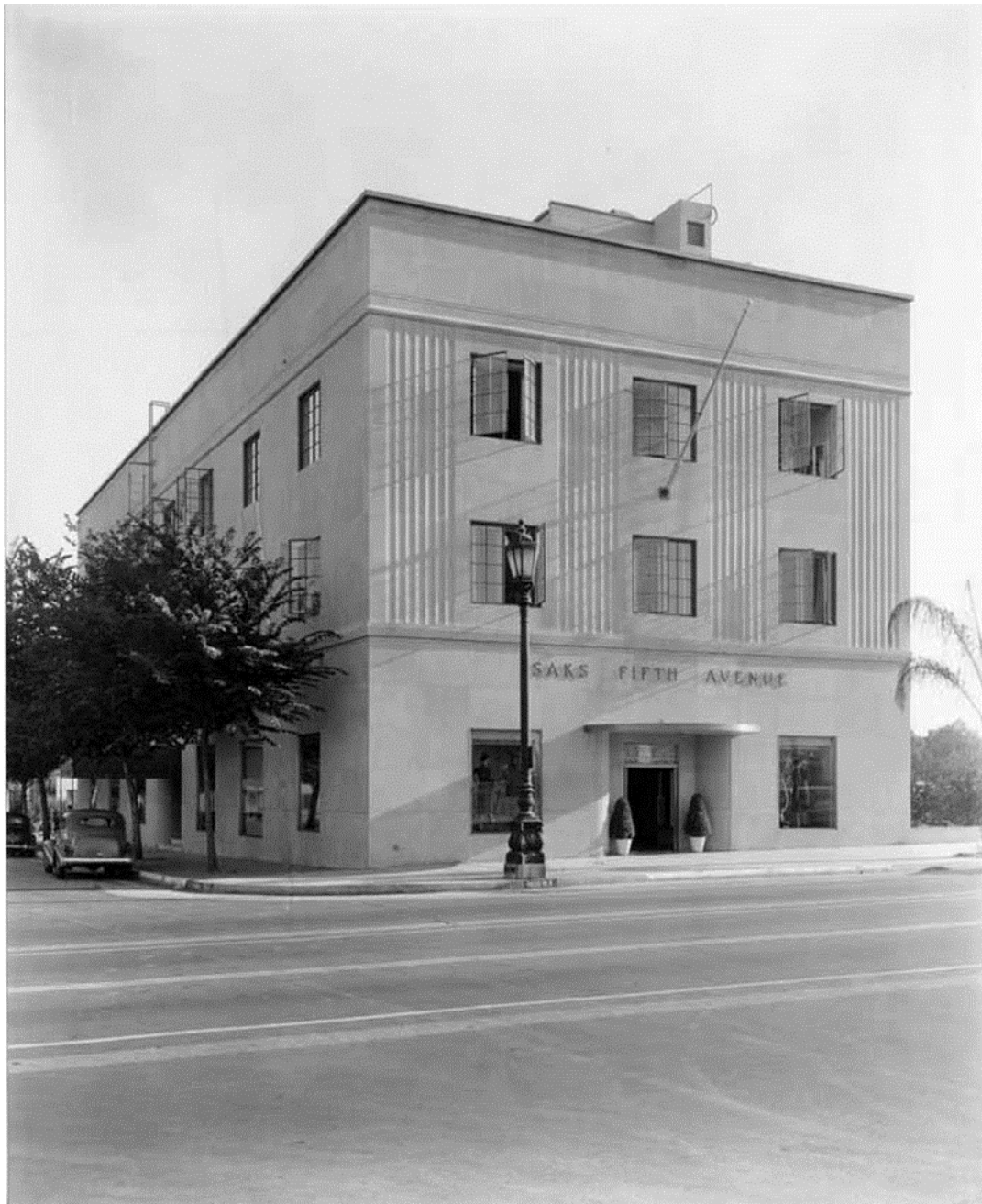
The initial store building (Unit #1) completed for Saks Fifth Avenue at 9600 Wilshire Boulevard, view southeast. California State Library
