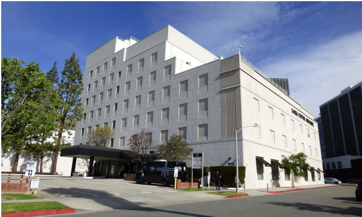
Image 17: South (rear) and east façades, view northwest from Peck Drive
