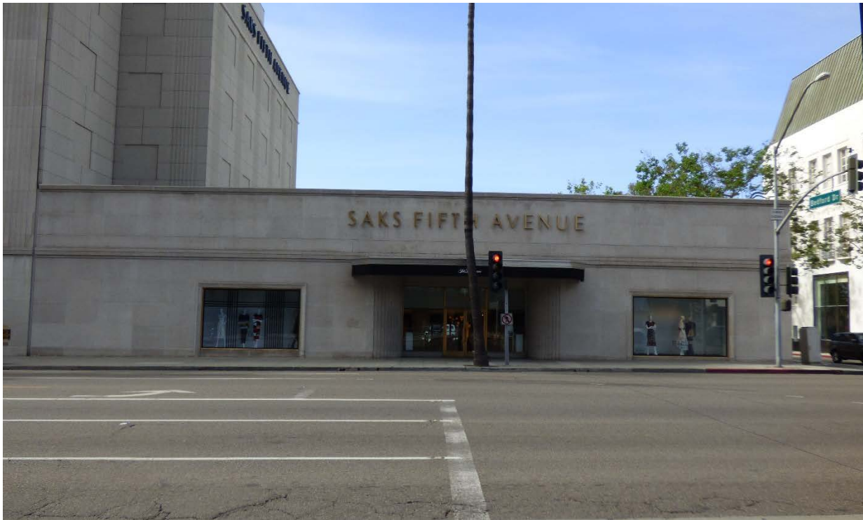
Image 11: 1994 addition, north façade, view south from Wilshire Boulevard
