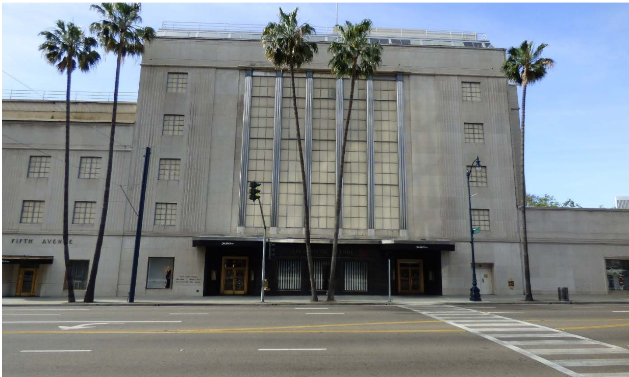
Image 6: Units #2/#3, north (primary) façade, view south from Wilshire Boulevard
