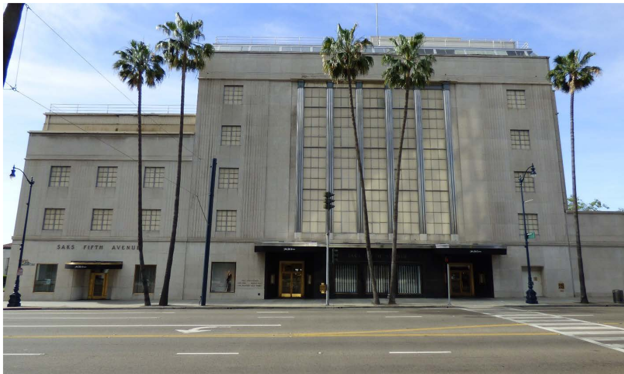
Image 2: North (primary) façade, view south from Wilshire Boulevard
