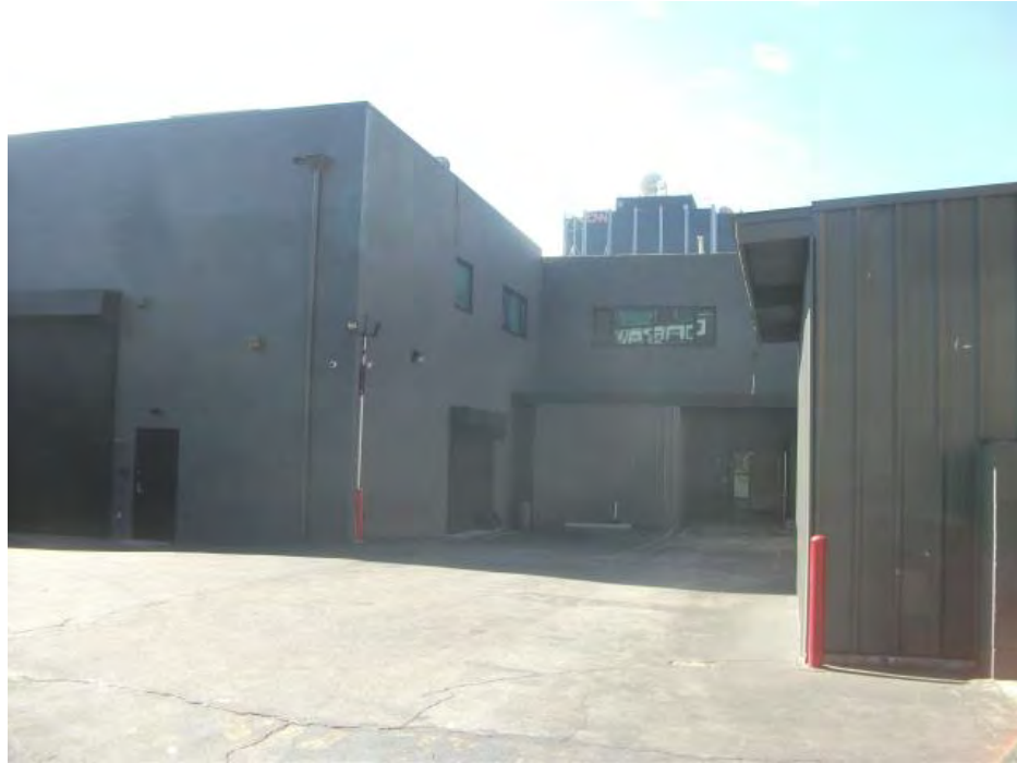
13. Goya Studios Sound Stage (1531 N. Cahuenga Blvd.) adjacent to east
