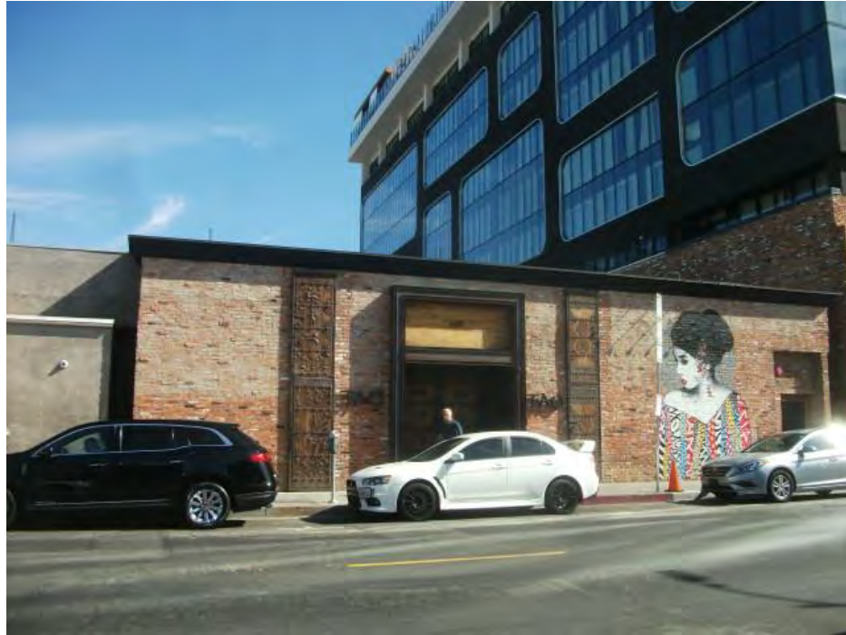
11. Tao Restaurant (6421 Selma Avenue) adjacent to north
