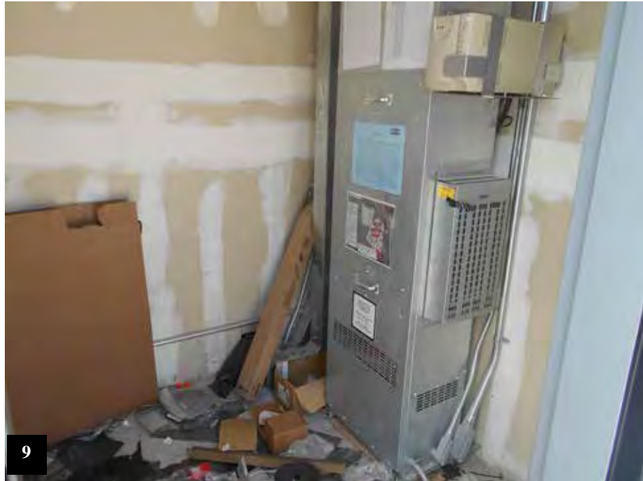
Elevator Room, 1550 North Wilcox Avenue
