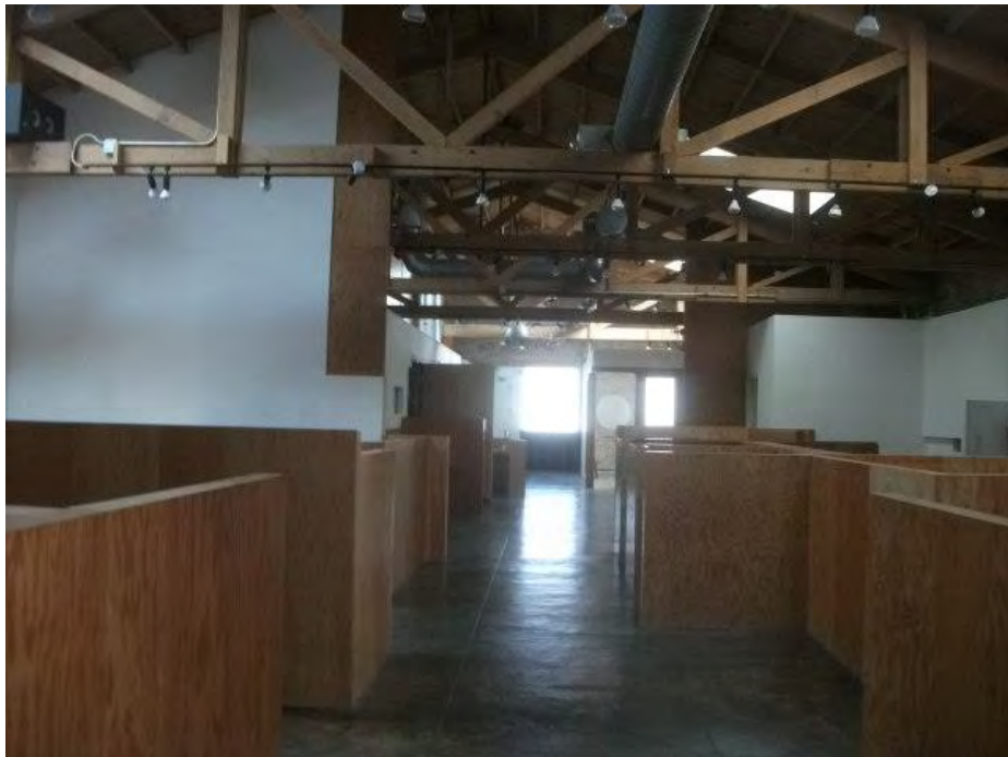
4. Interior looking north
