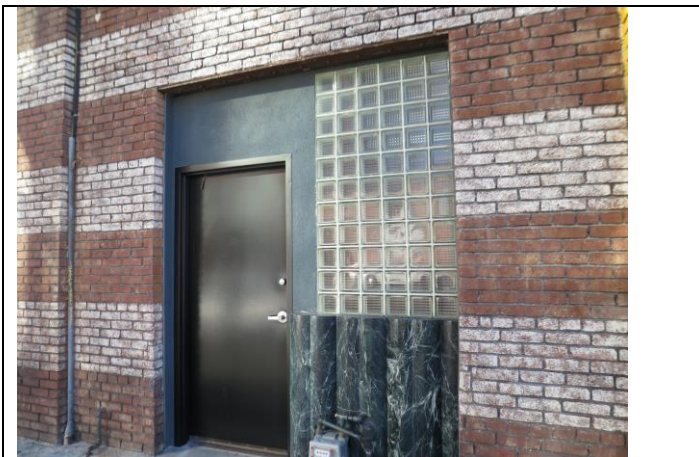
Image 3. Detail of east bay on north façade looking southwest.
