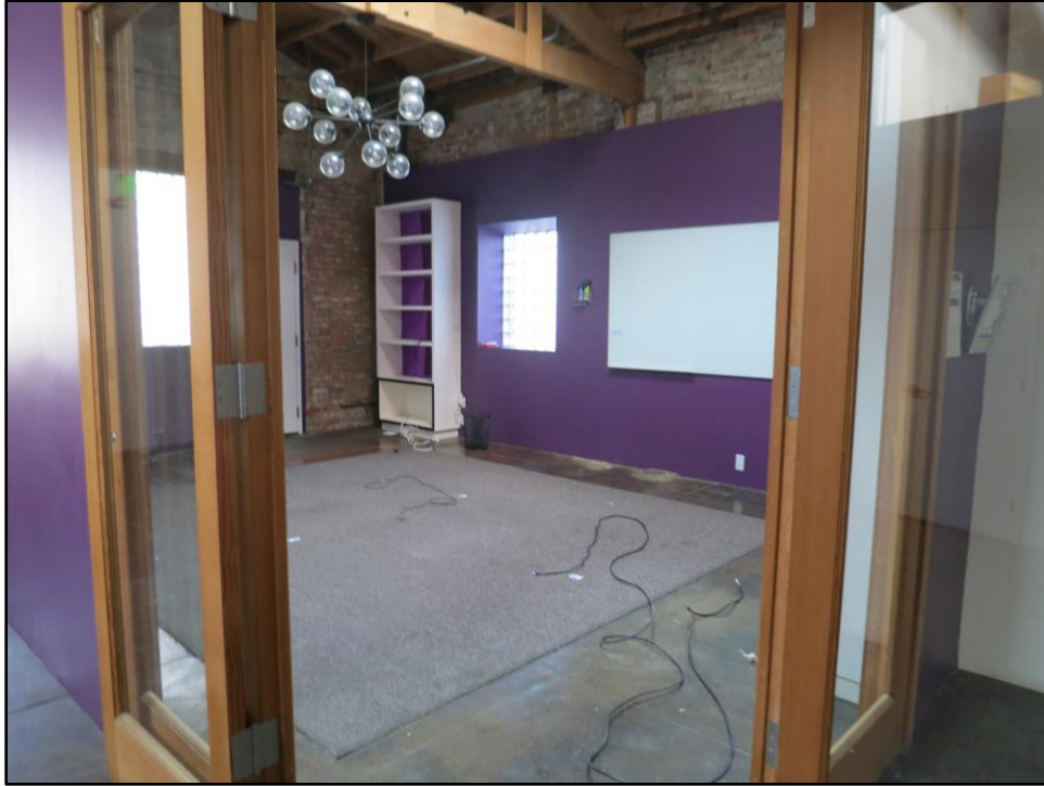
Figure 35. Interior view showing added walls below ceiling (2021).
