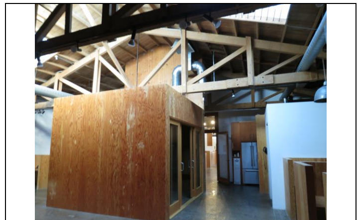
Image 6. Interior view showing ceiling truss.
