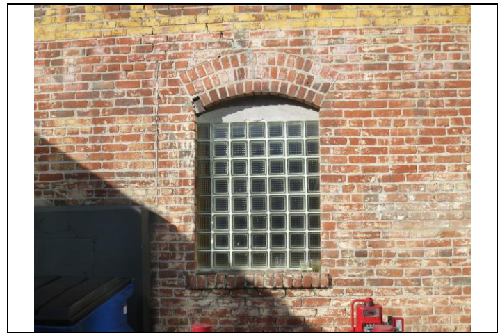
Image 4. Detail of window on east façade looking west.
