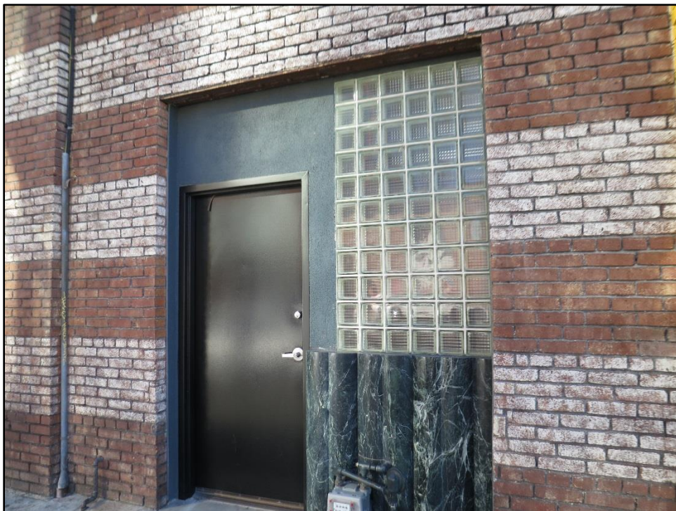
Figure 30. Detail of entrance in east bay, looking southeast.
