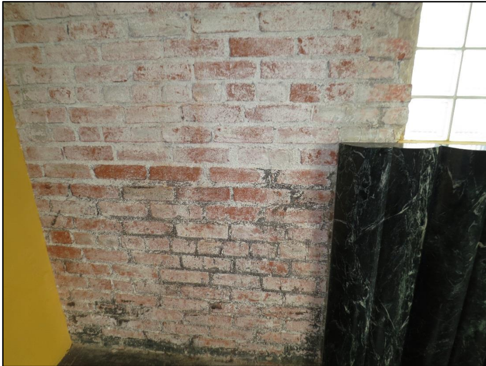
Figure 37. Detail of north wall showing added marble (2019).
