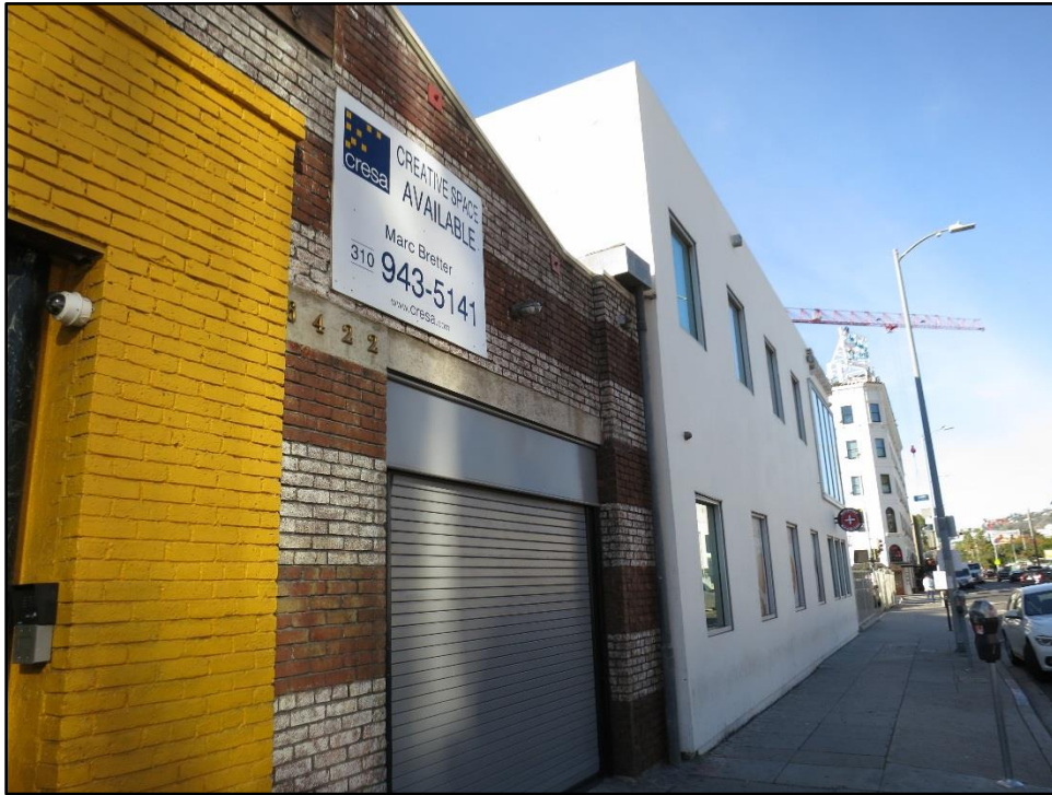
Figure 31. Roll-up door in west bay, looking southwest.
