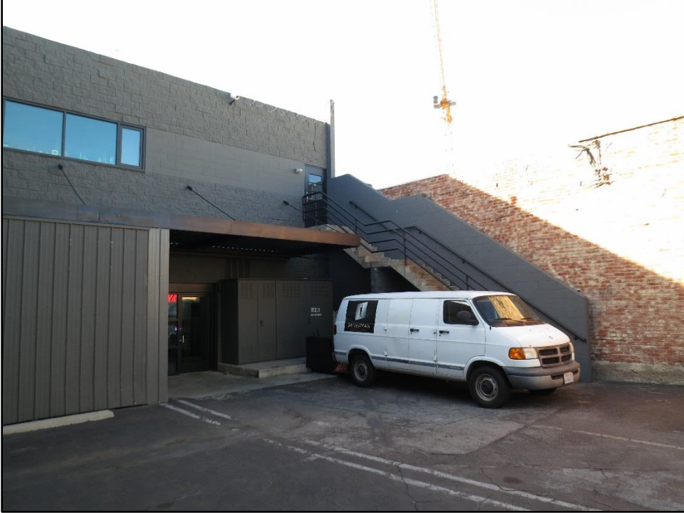
Figure 5. East façade of 6422 Selma Avenue, looking southwest.
