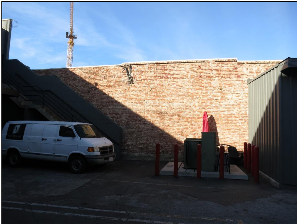
Figure 32. East façade, looking west.
