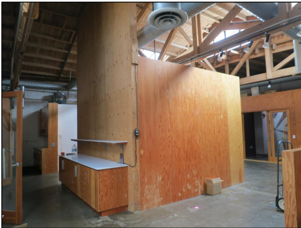
Figure 36. Interior view with ceiling trusses (2021).
