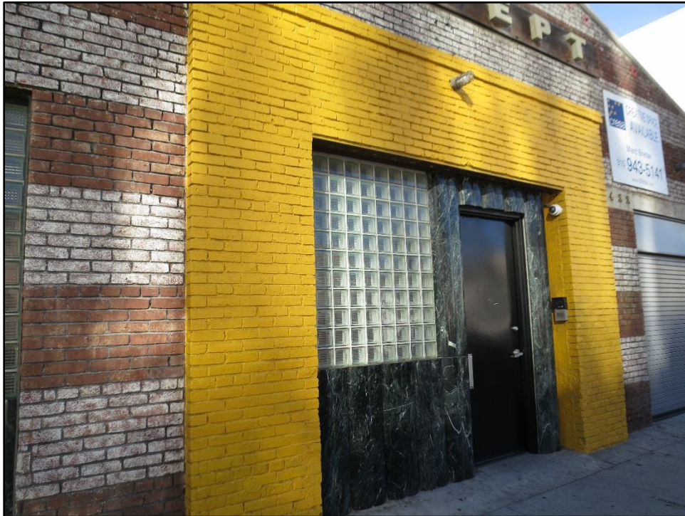
Figure 29. Detail of central glass block window and marble addition.
