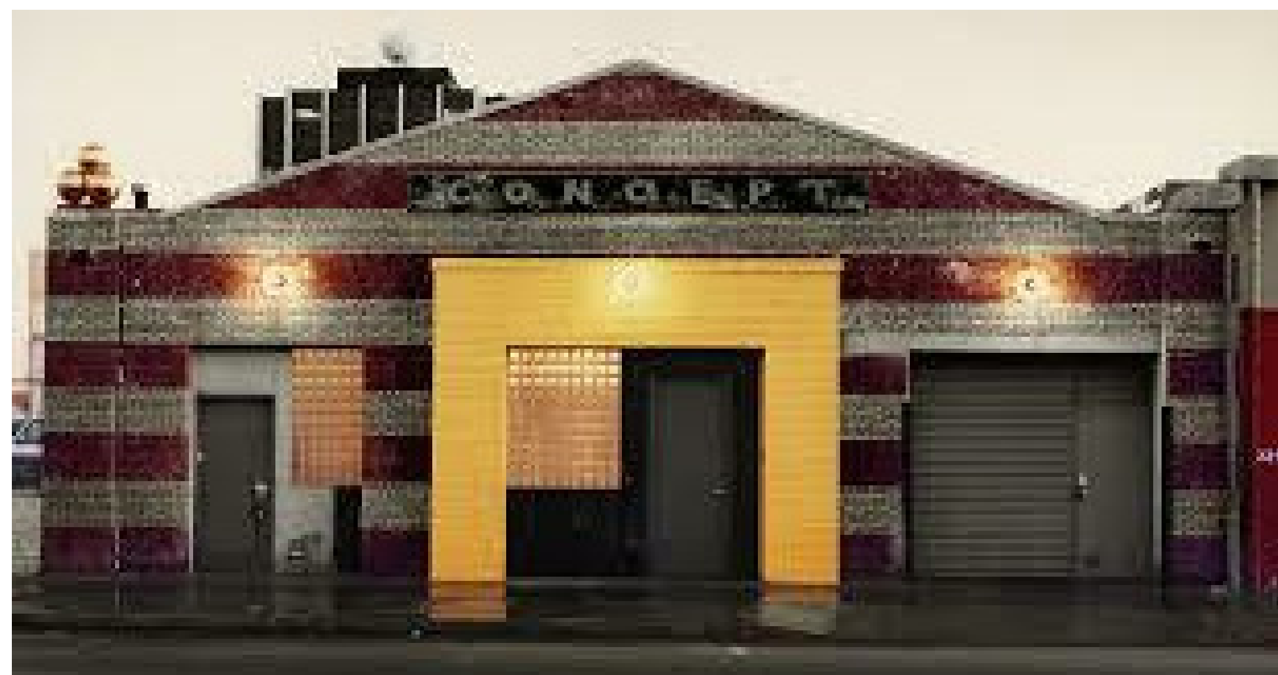
EXISTING FACADE OF 6422 SELMA AVE. (2020)
