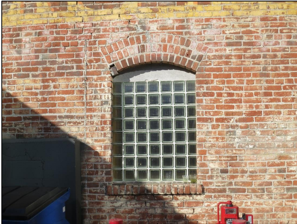
Figure 33. Detail of window on east façade.
