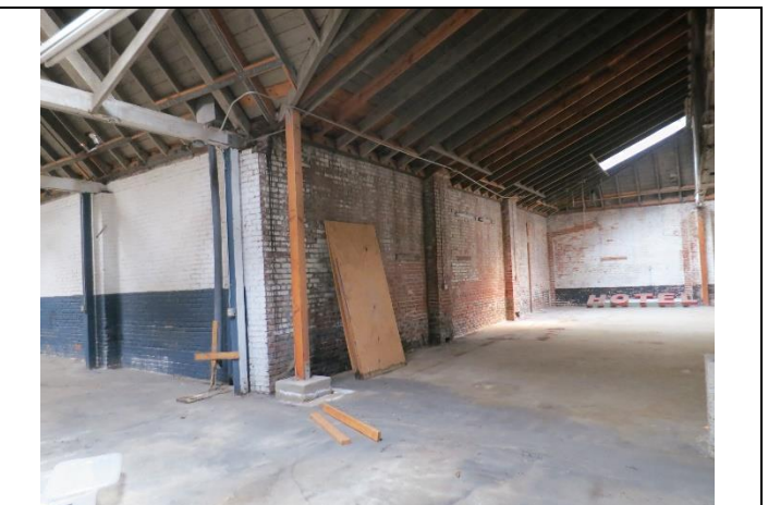
Image 4. View of interior looking northeast.
