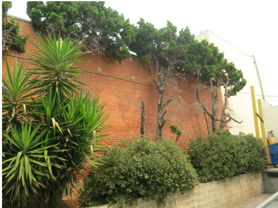
Figure 45. South façade of Gilbert Garage at 1550 North Wilcox, looking northeast.
