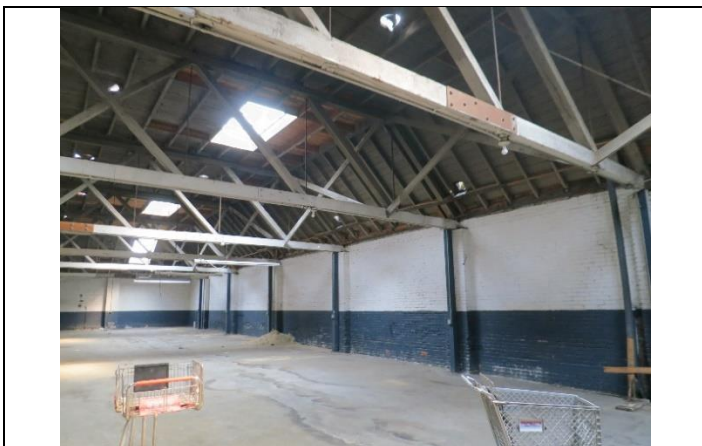
Image 5. View of interior looking northeast.
