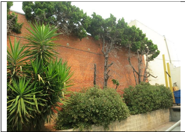
Image 1. View of south façade looking northeast.
