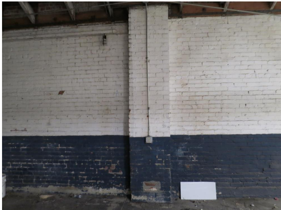
Figure 53. Detail of brick pilaster in Gilbert Garage.
