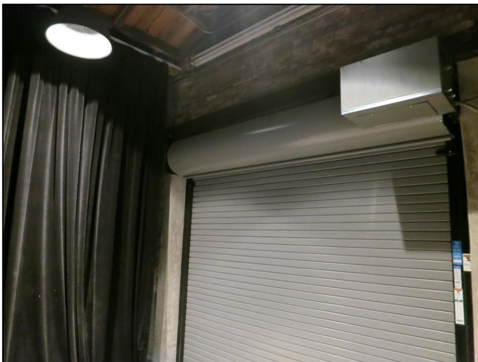
Figure 38. View of roll-up door in northwest corner room (2021).
