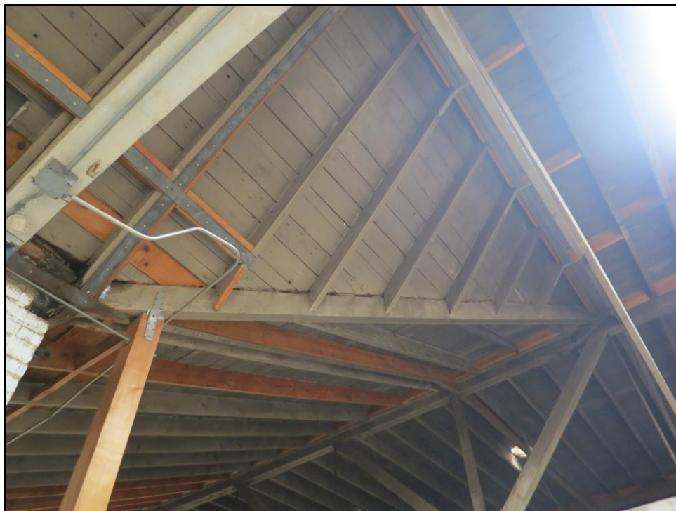
Figure 49. Detail of roof and trusses of Gilbert Garage.
