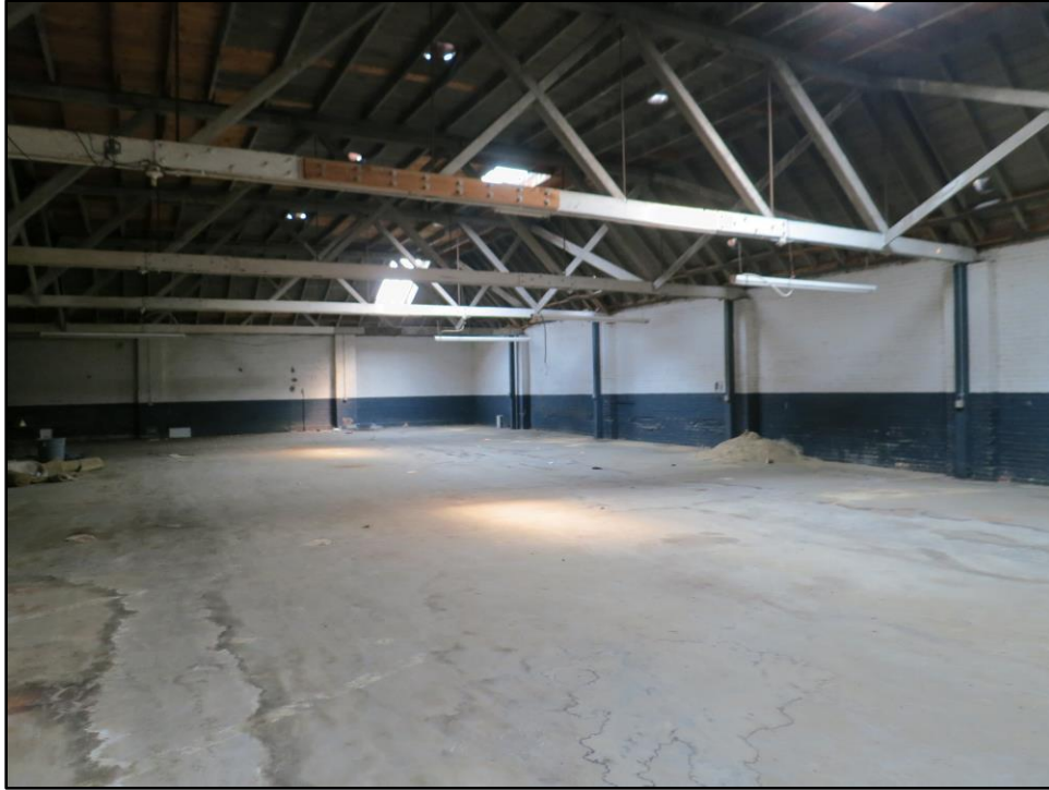
Figure 50. Interior view of Gilbert Garage, looking east.
