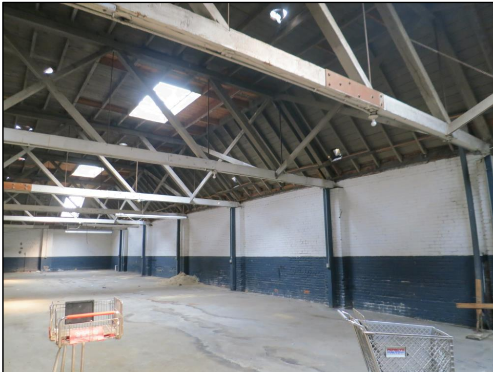
Figure 54. Overview of interior showing skylights in the Gilbert Garage.
