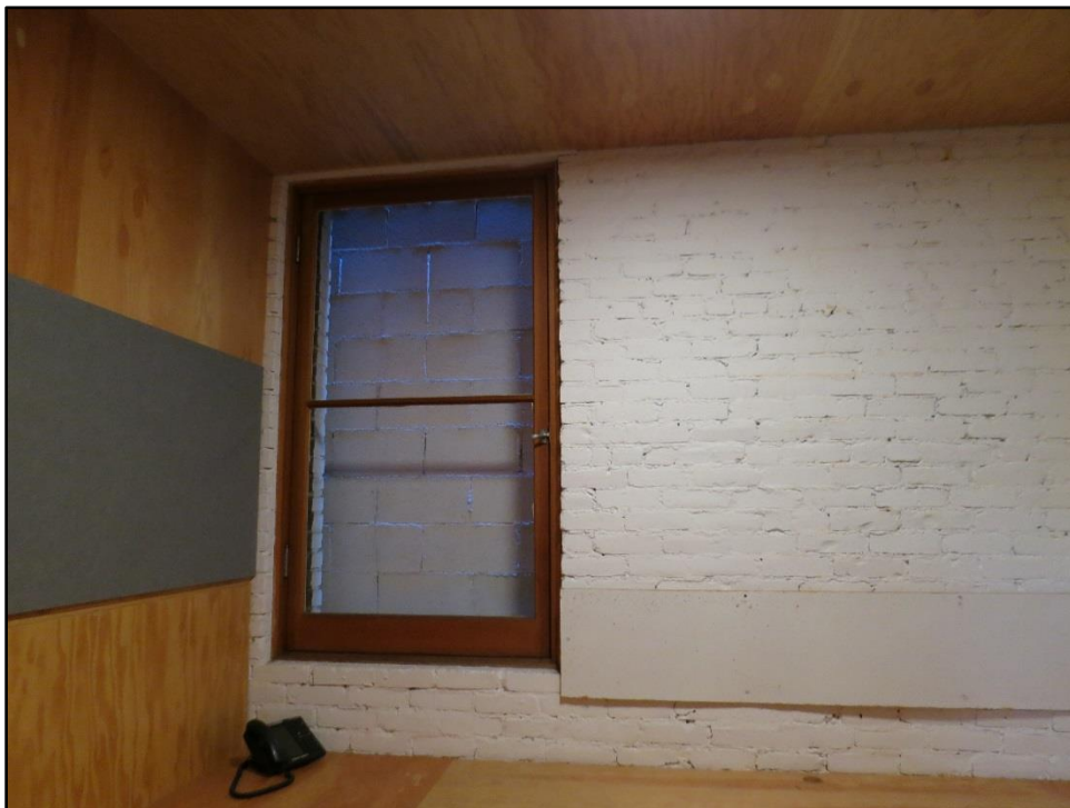
Figure 42. Window on east wall (2019).
