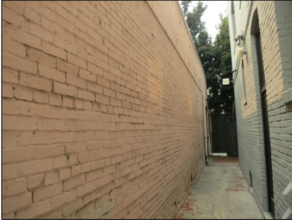
Figure 44. Detail of brickwork on west façade of Gilbert Garage, looking south.
