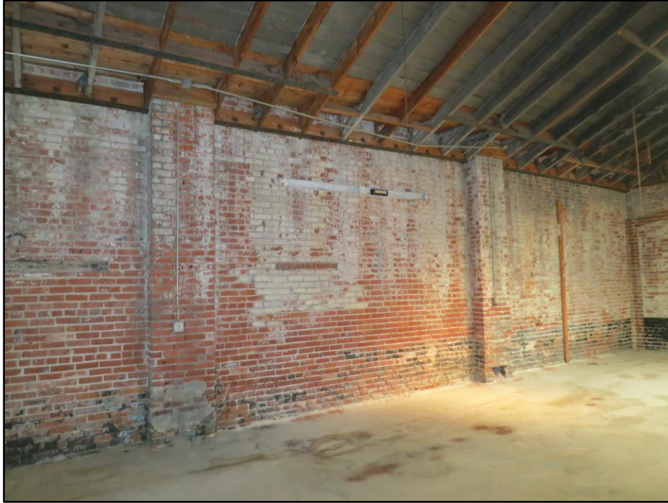
Figure 52. View of brick and pilasters on interior of Gilbert Garage.
