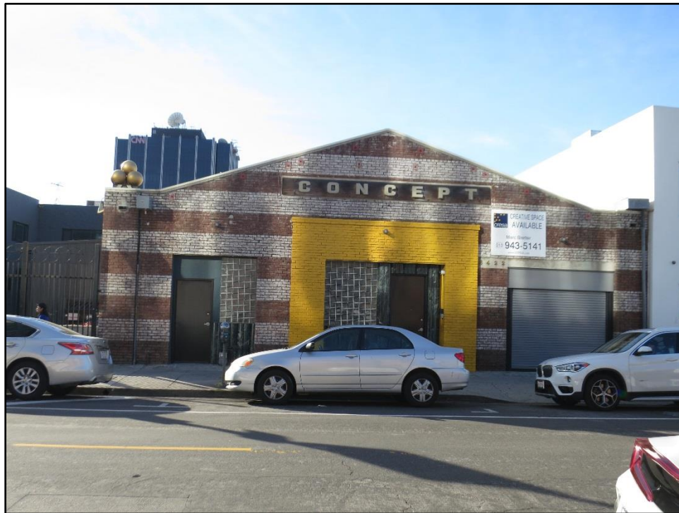
Figure 27. North façade, looking south.
