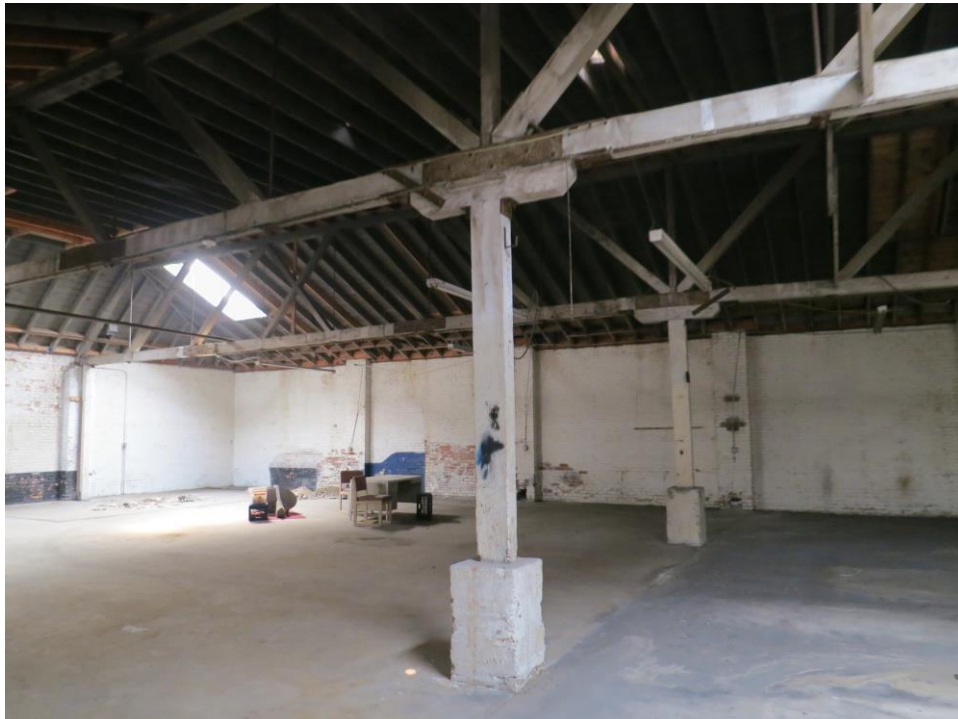
Figure 51. Detail of support post in center of Gilbert Garage, looking southeast.
