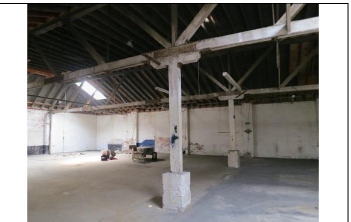
Image 6. Interior view showing ceiling truss support.
