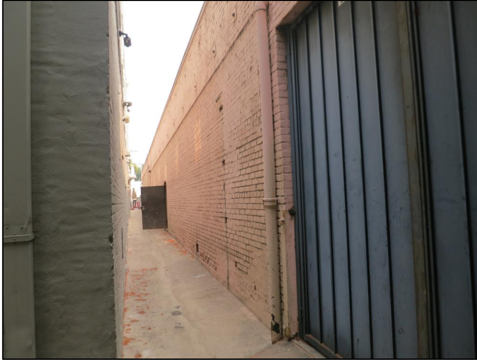
Figure 46. Detail of south door on west façade of Gilbert Garage, looking north.
