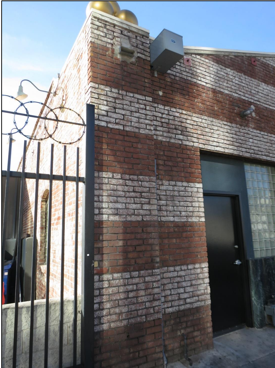
Figure 28. Detail of corner pilasters, looking south.
