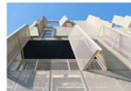
OPERABLE PERFORATED METAL PANEL MANUFACTURER: MANHOLD
