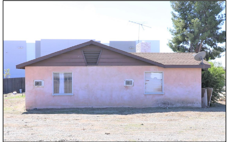
North elevation, view south (10/28/22).
