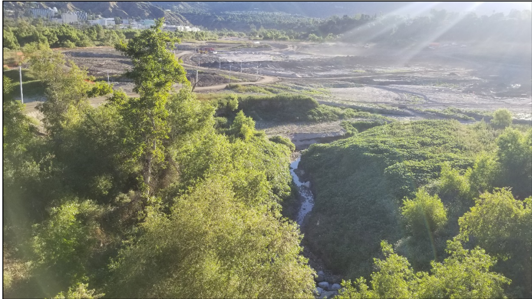
Photo 1. Looking northeast from pedestrian bridge at Flint Canyon Wash outlet into Devil's Gate Reservoir. June 10, 2020.
